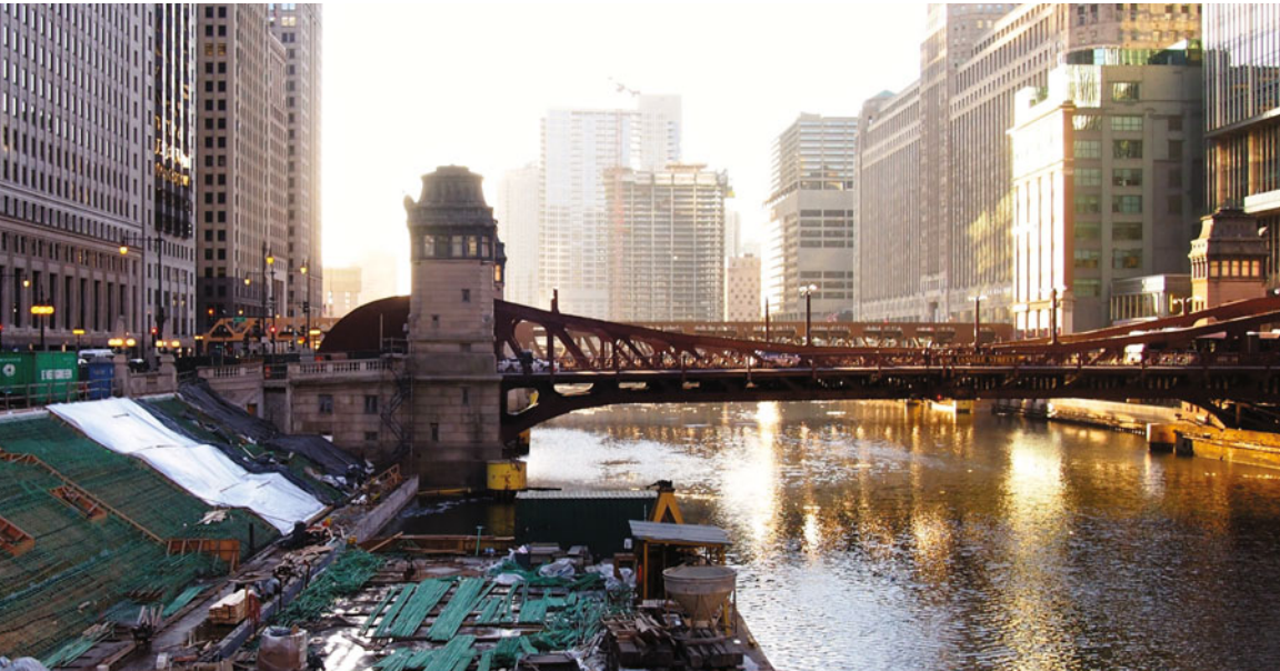
Construction of the Chicago Riverwalk (Shuja Kazi)
