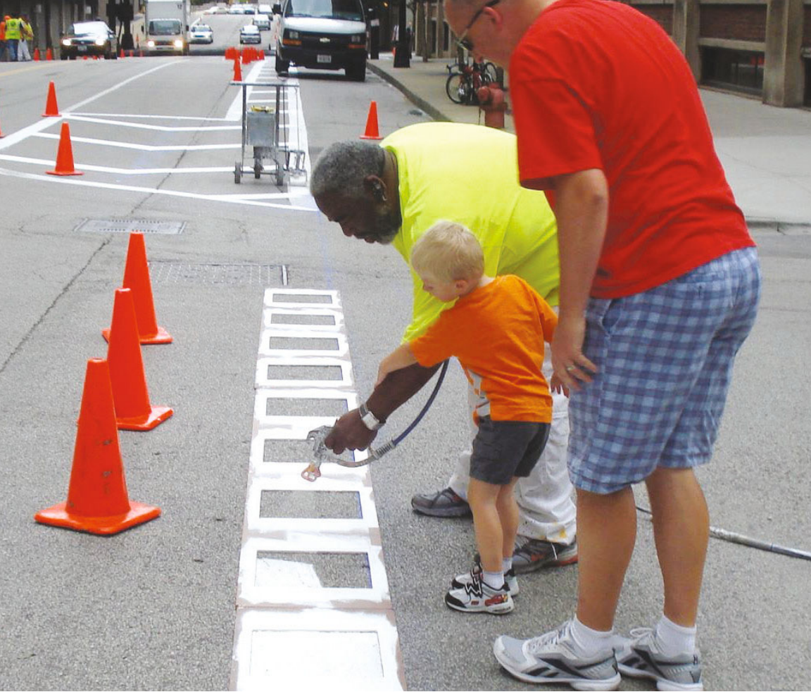
A young Chicagoan helps with bike lane construction (Chicago Bicycle Program)
