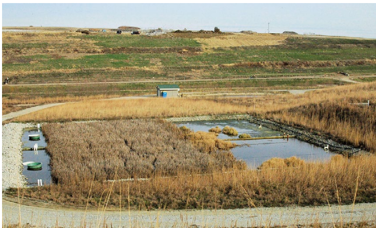
Fig. 11.19 Wetlands leachate treatment system located adjacent to an operating landfill
