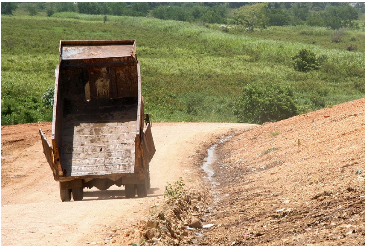
Fig. 11.3 Leachate seep flowing at base of landfill slope next to access road
