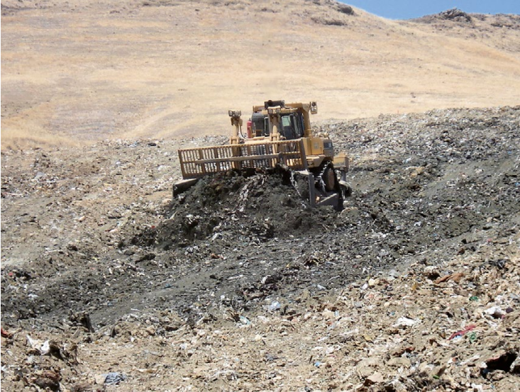
Fig. 17.11 Landfilled material reclaimed using scraping technique
