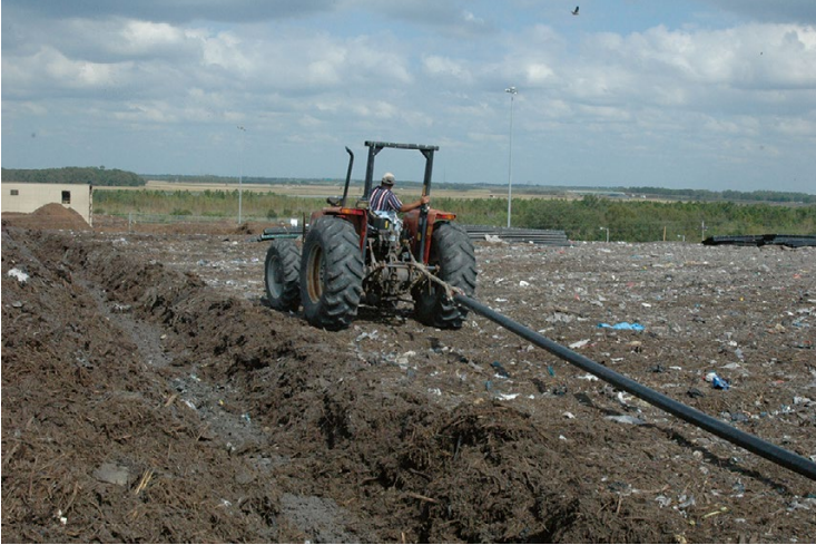
Fig. 9.9 Pulling welded HDPE pipe with tractor to proximity of excavated trench
