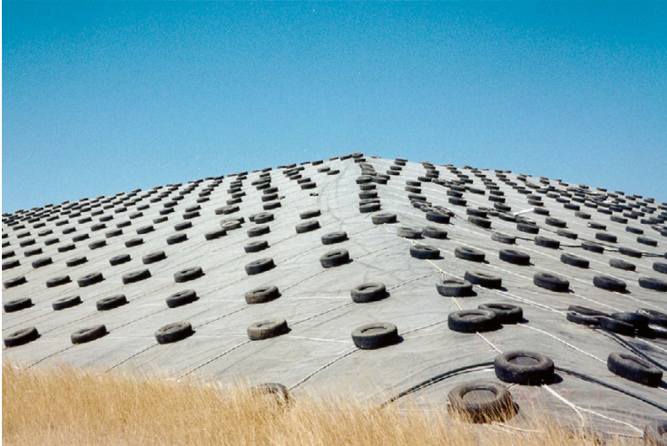
Fig. 4.8 View of Yolo County Landfill northeast anaerobic bioreactor cell; upon completion the slopes were covered with a geomembrane cap ballasted by tires (Photo courtesy of Ramin Yazdani)
