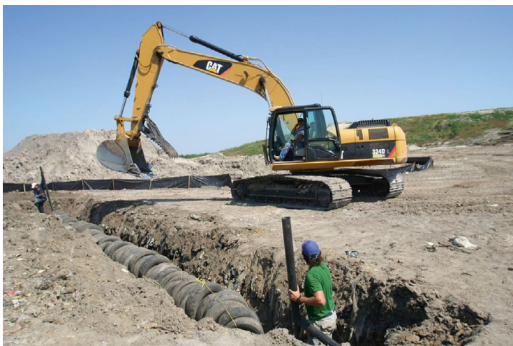
Fig. 7.6 Installation of liquids addition trench at the surface of a landfill
