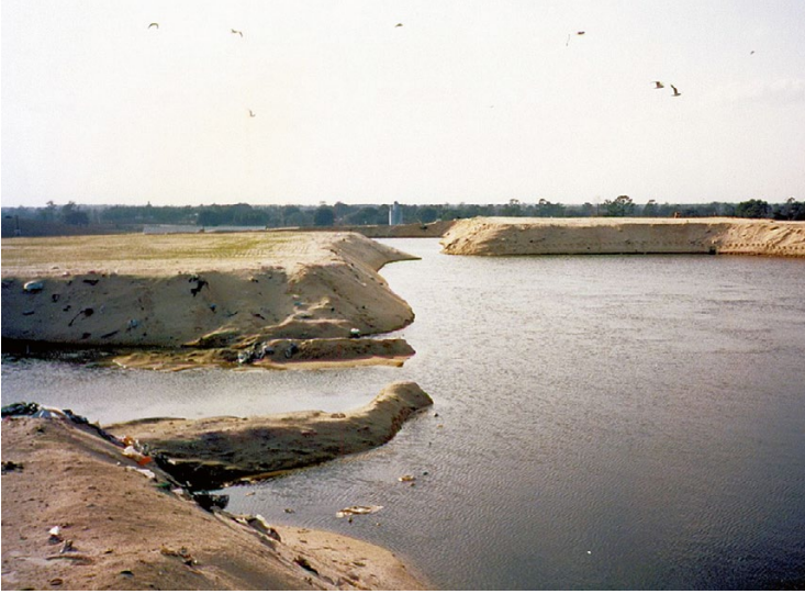
Fig. 4.4 Completed surface infiltration pond system ACSWL
