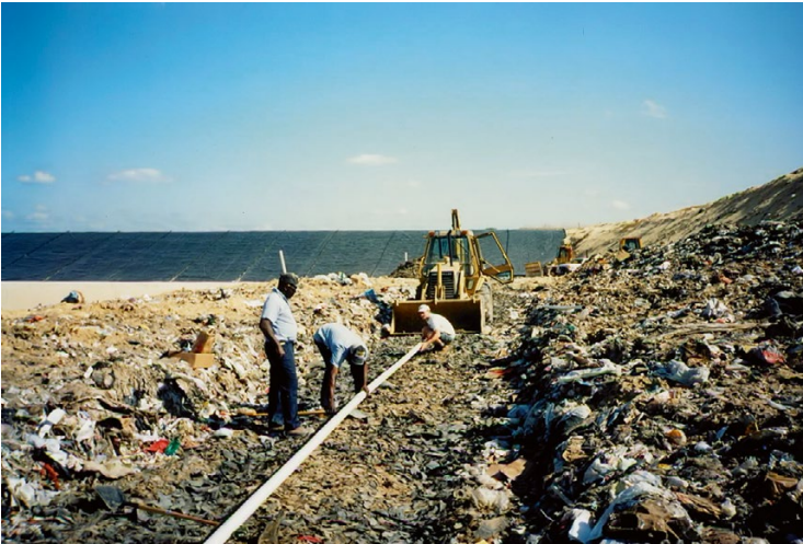
Fig. 4.5 Construction of horizontal leachate recirculation line at ACSWL
