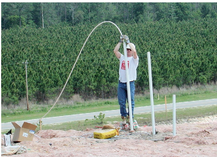
Fig. 4.15 The pipes were dislodged from the instrument bundles using a small diameter pipe to provide separation force required
