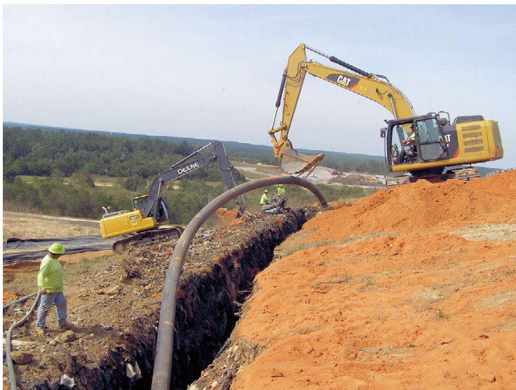
Fig. 13.7 Construction of LFG collection header
