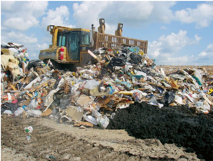
Fig. 6.9 MSW pushed on top of biosolids at the working face of landfill
