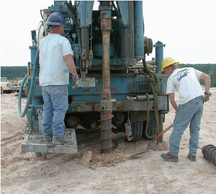
Fig. 8.3 Hollow stem auger equipment for drilling vertical wells in landfill waste
