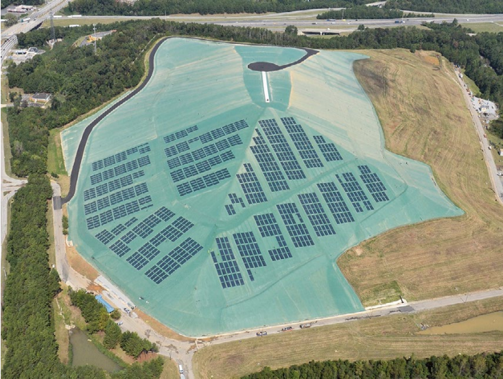
Fig. 19.5 Flexible solar panels on the EGC at a landfill in Georgia, US
