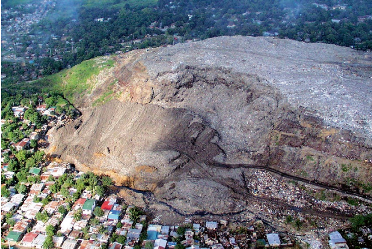
Fig. 12.1 Slope failure at the Payatas landfill, Philippines (Photo courtesy of Scott Merry)
