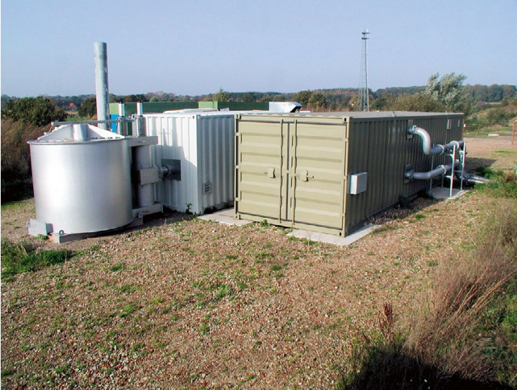
Fig. 4.30 Off-gas treatment system at German landfill undergoing aeration (Photo courtesy of Marco Ritzkowski)
