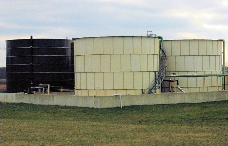
Fig. 11.16 Glass-lined steel leachate storage tanks surrounded by secondary containment system
