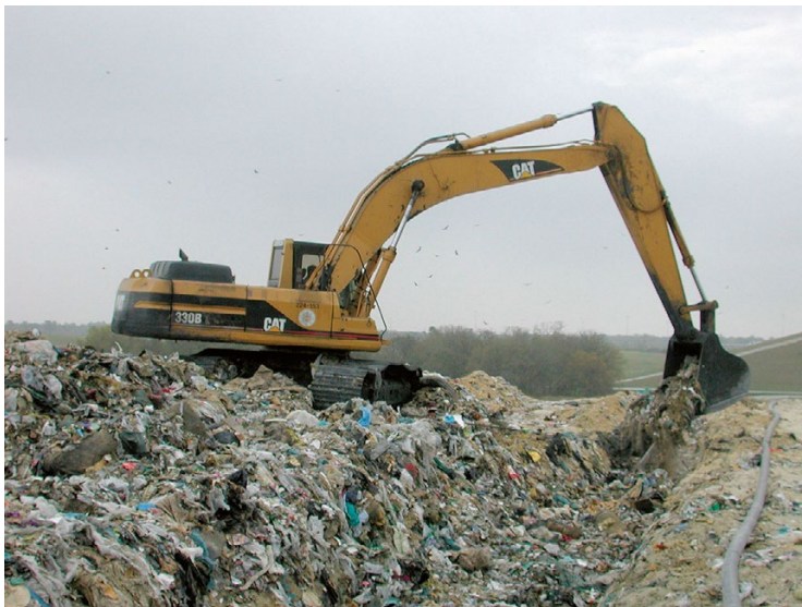
Fig. 9.3 Excavation of horizontal injection trench using a track excavator
