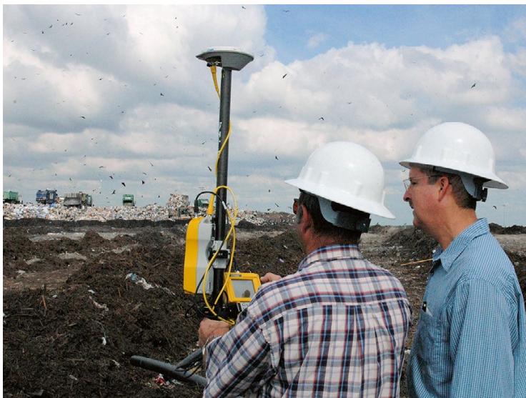
Fig. 16.11 Use of GPS technology to measure surface elevation and location
