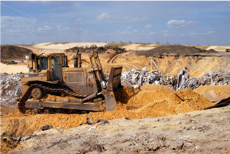
Fig. 1.6 Cover soil application at sanitary landfills aids in reducing odor, vectors, fires and helps in the control of storm water and leachate
