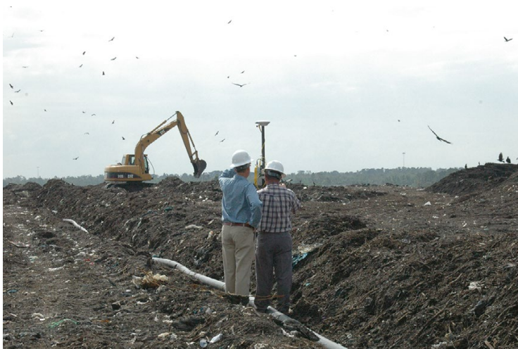
Fig. 15.1 Operator inspecting and observing construction of a liquids addition device
