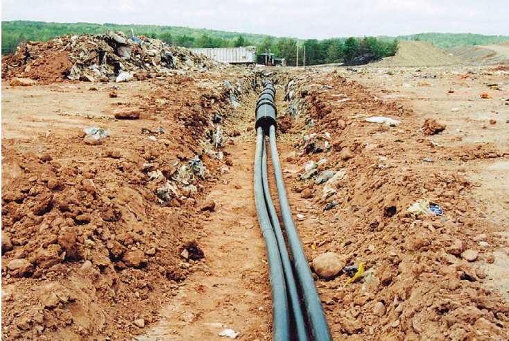
Fig. 14.17 VSA trench under construction (Photo courtesy of David Hansen)
