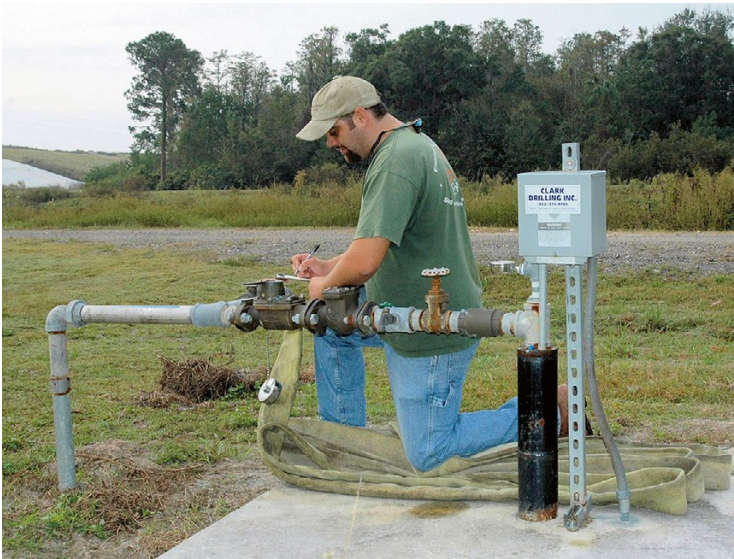
Fig. 6.2 Groundwater well used for extracting fresh water to mix with leachate before recirculating to a landfill
