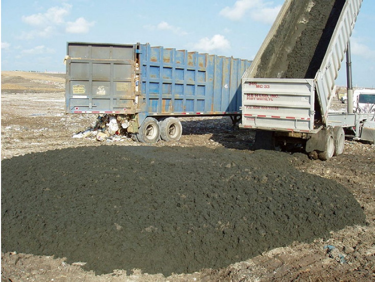
Fig. 6.3 A truck load of biosolids unloaded at the working face of a landfill
