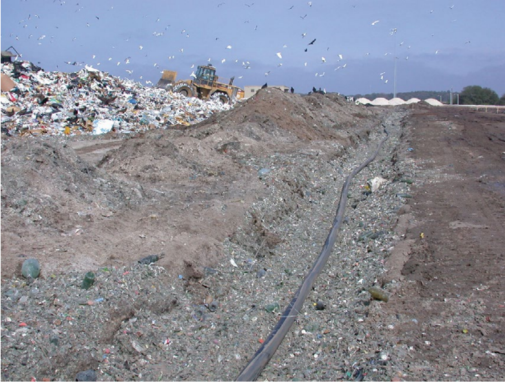
Fig. 9.6 HDPE liquids distribution pipe in the process of being placed on top of a bottom bedding layer of crushed glass in a horizontal trench
