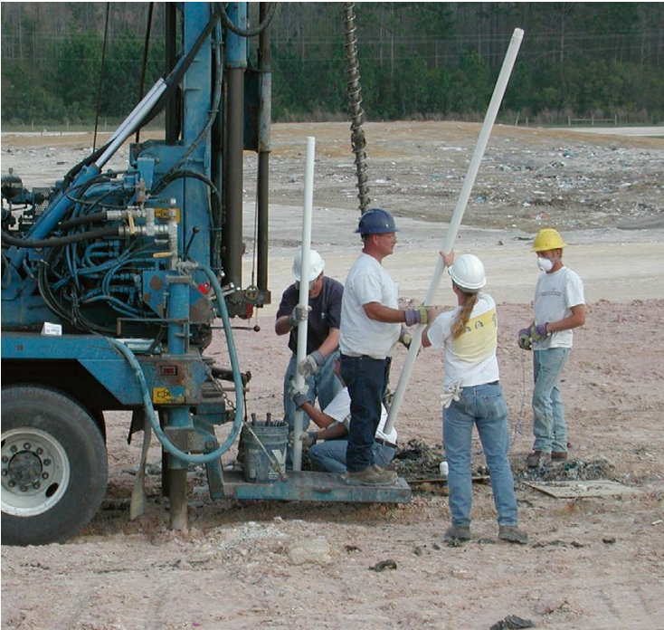
Fig. 8.8 Construction of small diameter liquids addition wells
