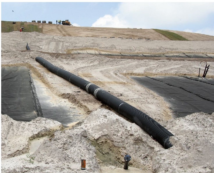
Fig. 17.2 Barrier layer final cover system under construction
