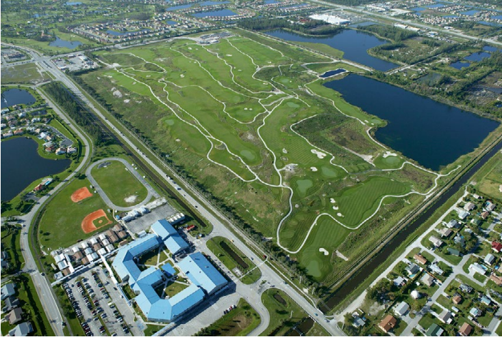
Fig. 17.14 Golf course constructed on a closed MSW landfill (Photo courtesy of CDM-Smith)
