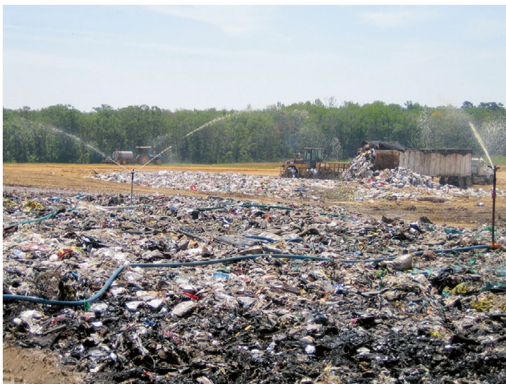
Fig. 7.3 Spray irrigation at the landfill surface prior to cover soil placement using portable spray heads
