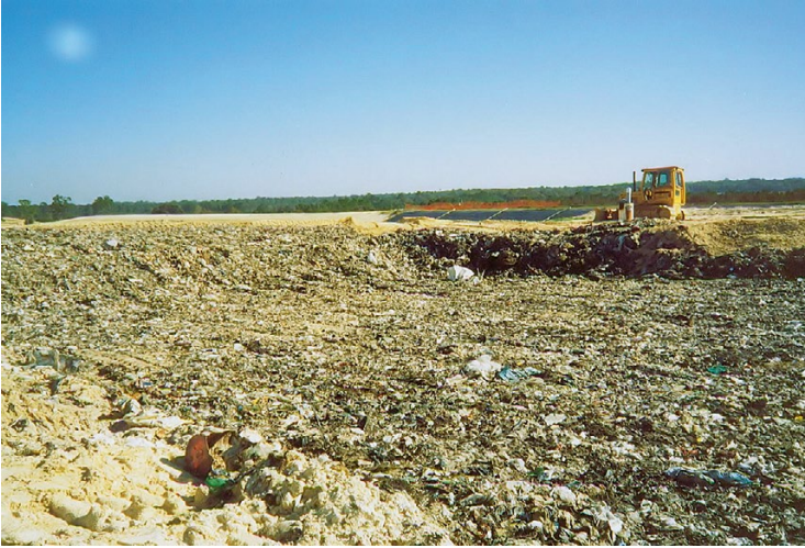
Fig. 4.3 Excavation of surface infiltration pond at ACSWL
