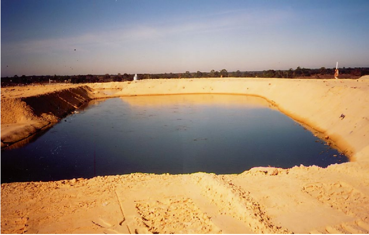
Fig. 7.5 Leachate infiltration pond at the landfill surface
