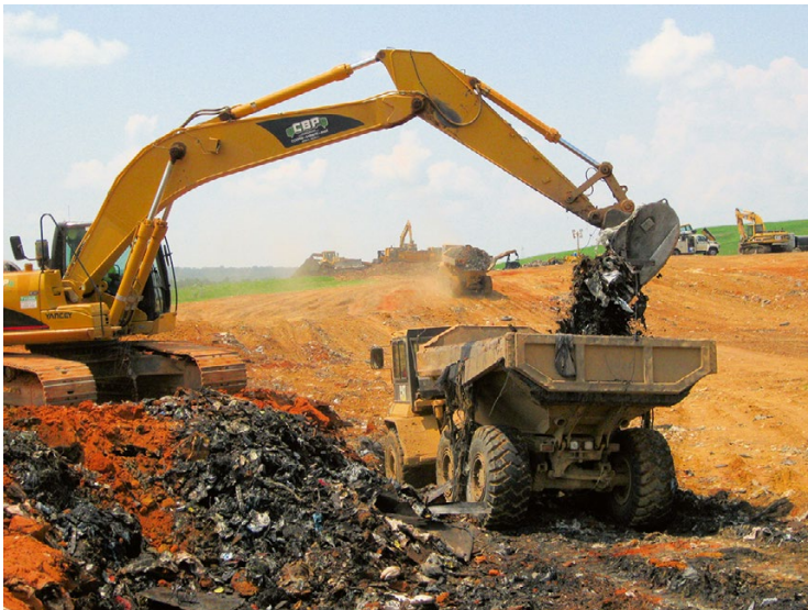
Fig. 17.10 Landfilled material reclaimed using excavation technique
