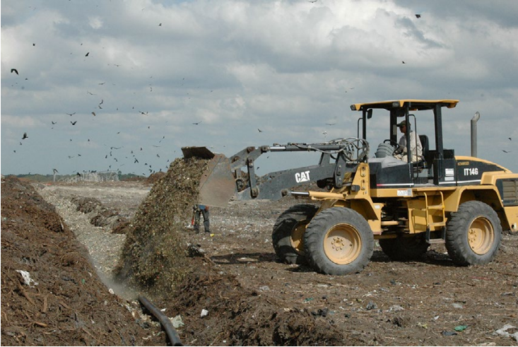
Fig. 9.7 Placement of crushed glass on top of HDPE liquids distribution pipe in horizontal trench
