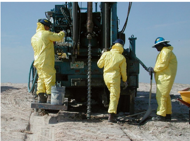
Fig. 8.4 Solid shaft open flight auger for drilling vertical wells in landfilled waste
