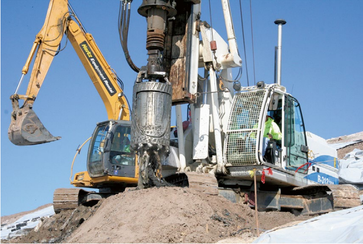
Fig. 13.3 Bucket auger rig for excavating borehole for LFG well
