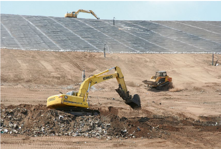
Fig. 2.9 Construction of a closure system at a landfill site
