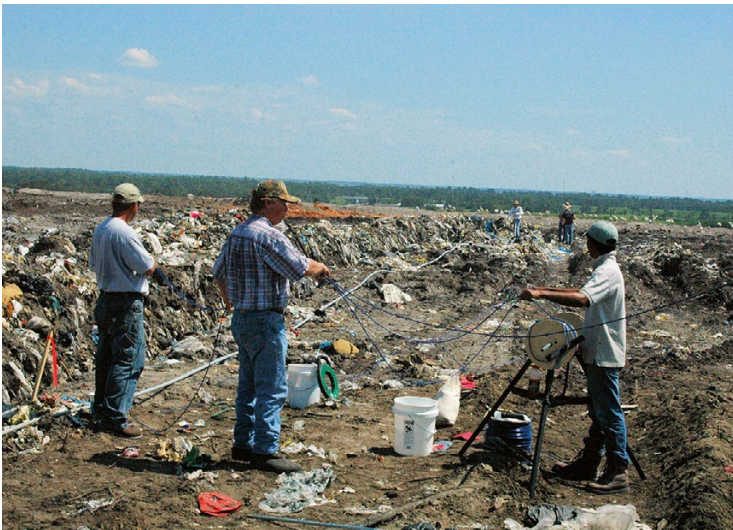
Fig. 4.24 Installation of buried pore water pressure transducers surrounding horizontal injection lines
