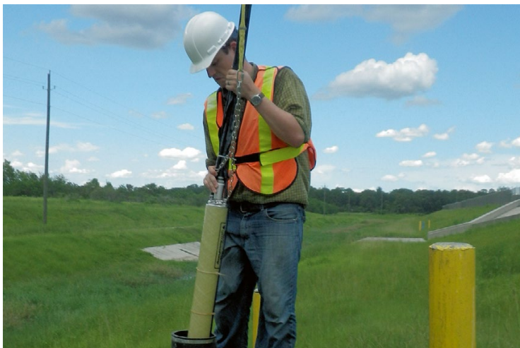
Fig. 13.13 Leachate pumps in gas collection wells
