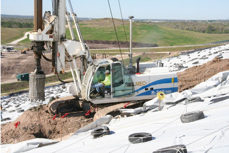
Fig. 8.2 Bucket auger rig for drilling vertical wells in landfill waste
