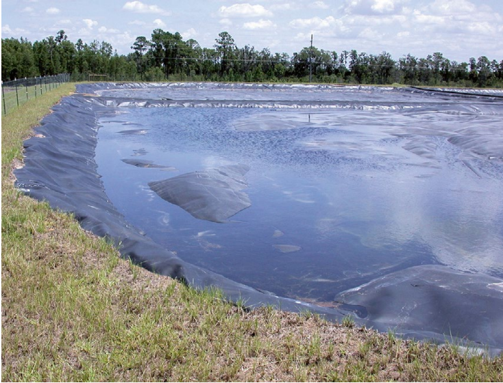
Fig. 11.14 HDPE lined leachate storage pond equipped with surface rain cover
