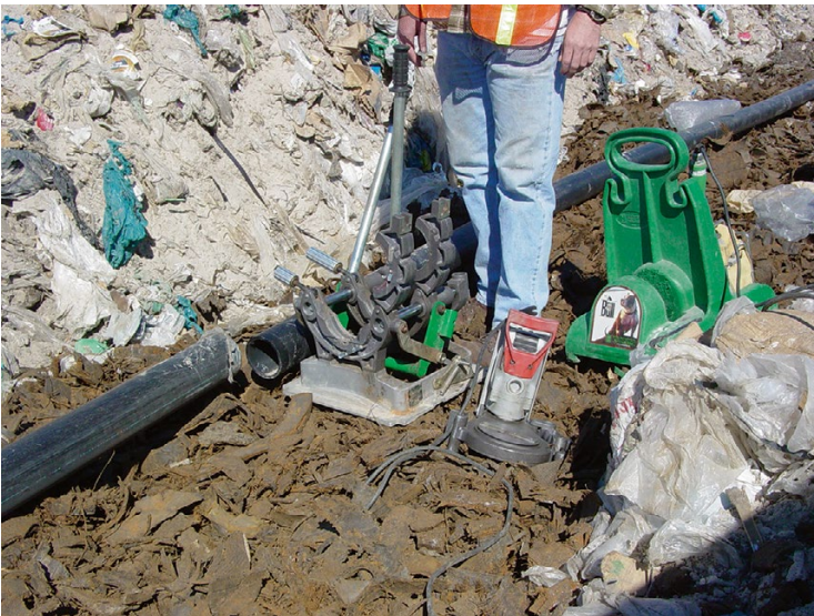
Fig. 9.8 Welding HDPE pipe in trench during construction
