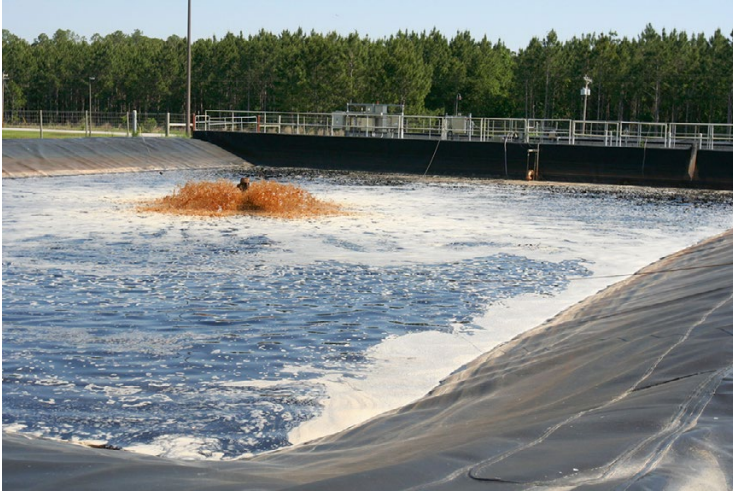
Fig. 6.1 Leachate storage and aeration pond equipped with a pump for recirculating leachate to the landfill
