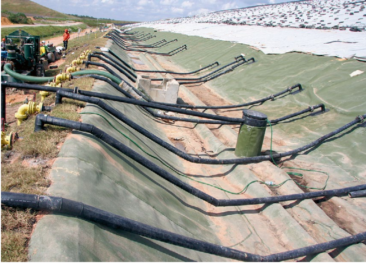
Fig. 4.26 Toe drain beneath liner at the base of the PCNCL
