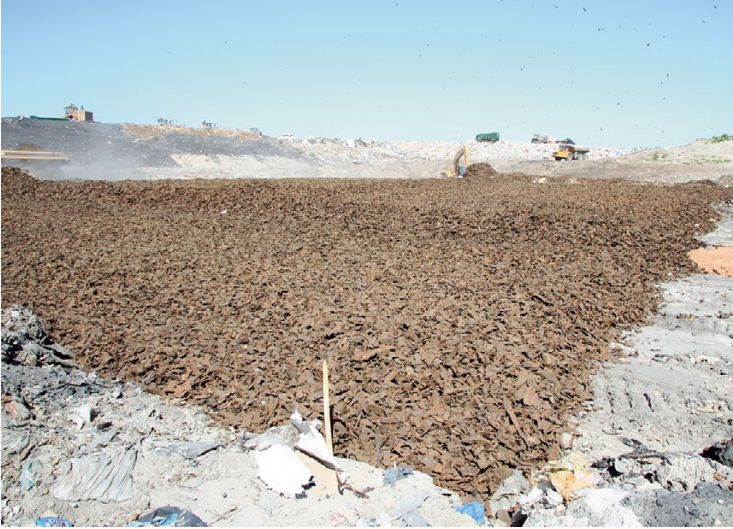
Fig. 4.25 Permeable blanket of shredded tires used for liquids addition (under construction)
