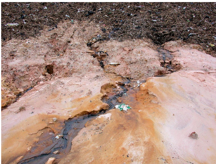
Fig. 11.1 Seep emergence from side slope of landfill
