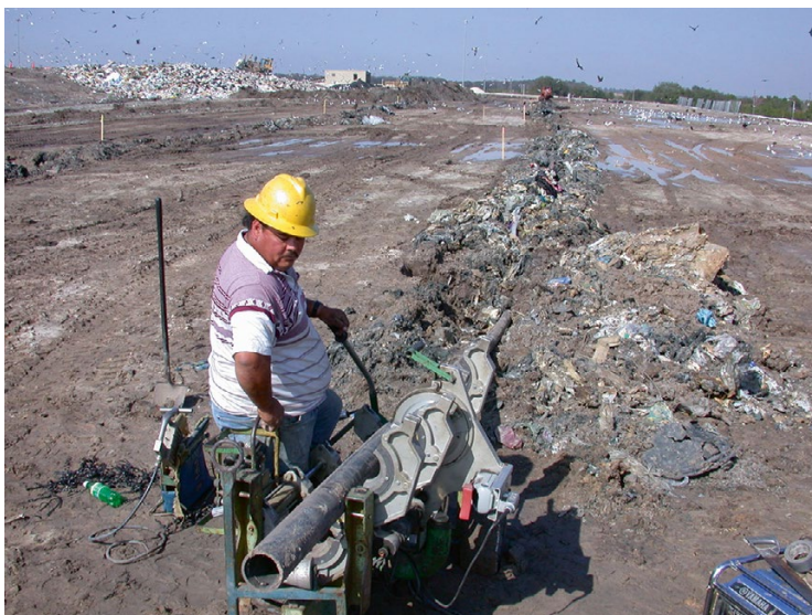
Fig. 9.14 Perforated HDPE injection pipe installed using a trenching device
