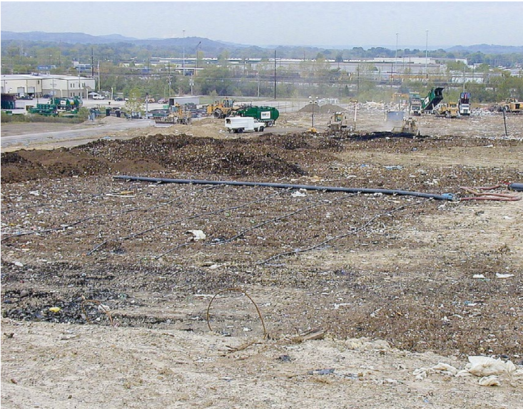
Fig. 4.28 Surface drip liquids addition system at Outer Loop landfill (Photo courtesy of Waste Management Inc.)
