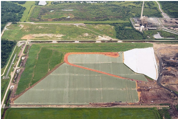
Fig. 17.5 Exposed geomembranes cap used as final cover (Photo courtesy of Jones Edmunds)
