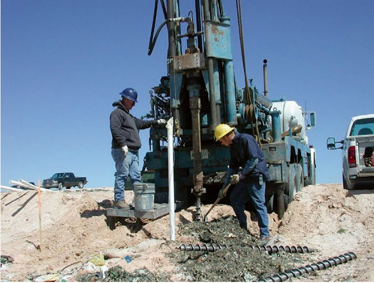
Fig. 8.7 Drilling small diameter liquid addition wells in a landfill
