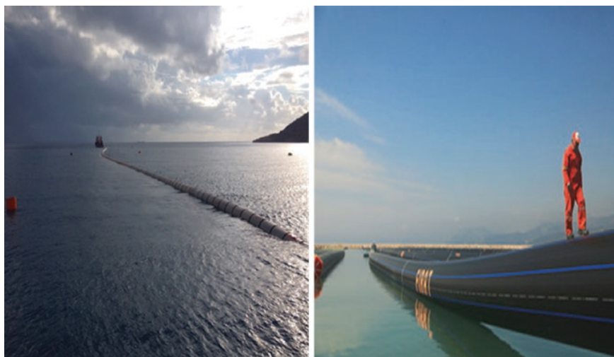
Fig. 13 The HDPE pipes used in the project
