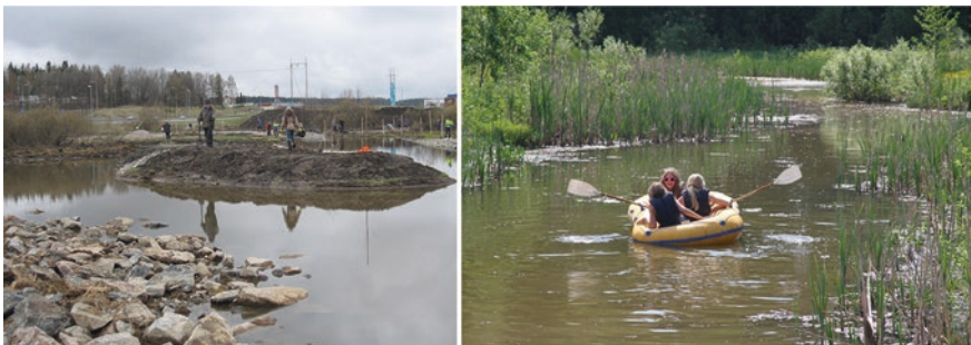
Fig. 10 The Nummela Gateway wetland park was constructed in 2010 by wintertime dry excavation, with some native trees planted on the site by an engaging volunteer event in May (left). In June 2013, the first children's summer camp was held at the site (right). Photograph Salminen (2010, 2013)
