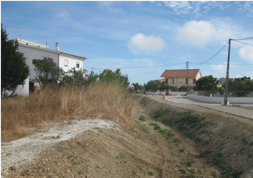
Fig. 7 The measures implemented 2013 for flood protection in the Sassoeiros stream. Without any other measures, e.g., settling adequate plants, the water flow will wash the banks away in the next rain. Photograph Smaniotto (2013)
