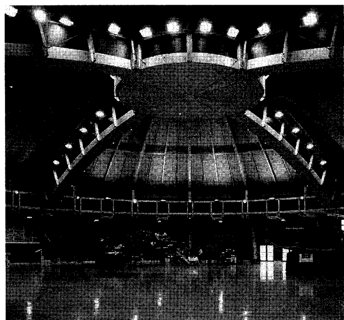
Fig 35. A glued laminated timber dome, Bournemouth International Centre
