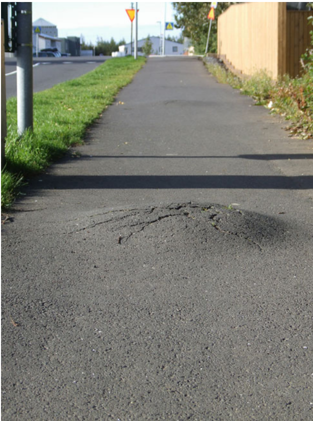
Fig. 10.26 It is necessary to place frost-free materials below concrete and buildings. Failure to use proper materials causes frost damage like seen on this asphalt path
