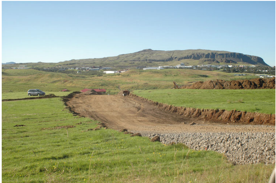
Fig. 2.11 Urbanization—road construction destroying valuable agricultural soil
