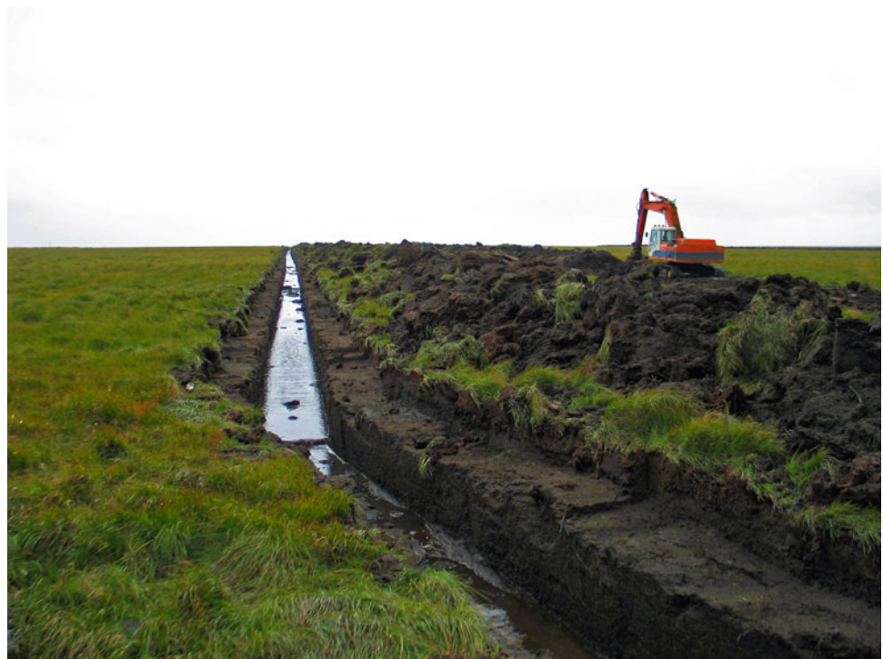
Fig. 12.20 Drainage ditch being put in a wetland in the South. The ecosystem changes towards a grassland, but a large amount of CO 2 is released by oxidation of the organic rich wetlands. Photo © Hlynur Oskarsson, AUI
