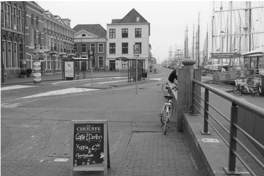
Fig. 25.6 Placeholder for demountable barriers (in the pillar, fence will be replaced by wooden boards) at the riverside quay in Kampen. In the pavement a hidden piston embankment can be seen (highlighted for better visibility)
