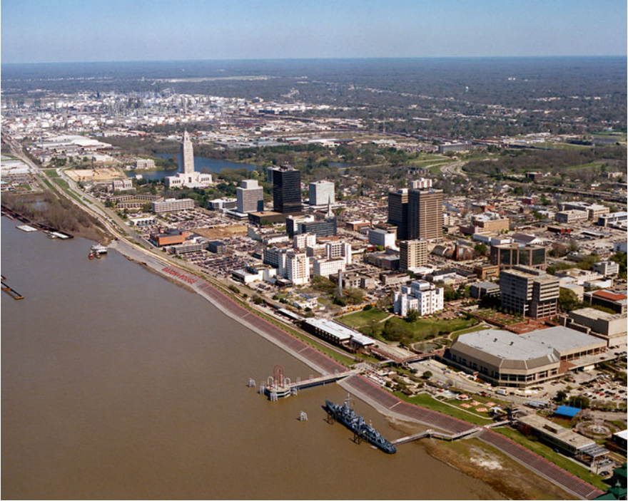
Fig. 4.14 Aerial view of the riverfront area of Baton Rouge USA (1990) with the Mississippi River in the foreground. The Exxon Mobile refinery and other industrial land uses can be seen in top left corner. The river between Baton Rouge and New Orleans has numerous oil refineries and petrochemical plants ( http://commons.wikimedia.org/wiki/File:Baton_Rouge_Louisiana_waterfront_aerial_view.jpg , By Michael Maples, U.S. Army Corps of Engineers, [Public domain], via Wikimedia Commons)
