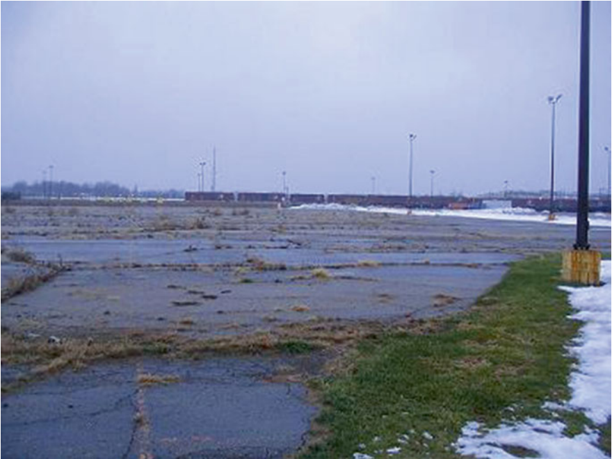
Fig. 4.5 Flint's 235-acre complex known as Buick City was in operation from 1904 until 1999. The facility was recently demolished. According to Wikipedia ( http://commons.wikimedia.org/wiki/File:Buickcityflint ) (Photograph by user Blueskiesfalling (Own work) [Public domain], via Wikimedia Commons)
