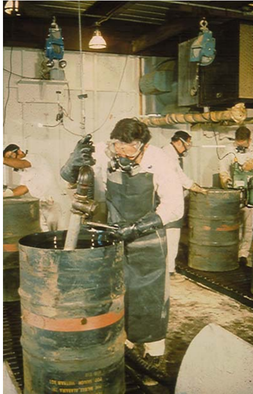
Fig. 4.25 Removing drum lids and contents (Agent Orange) being removed by a suction wand, Operation PACER HO, Naval Construction Battalion Center, Gulfport, Mississippi 24 May–10 June 1977 (Photograph courtesy of USAF Occupational and Environmental Health Laboratory, Brooks AFB, Texas)
