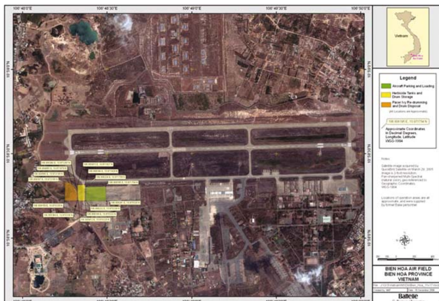
Fig. 8.4 A Satellite Image Map of Bien Hoa Air Base showing the location of the December 1966–February 1970 RANCH HAND Operations (Green and Yellow) the site of PACER IVY Operations April 1970–March 1972 ( Brown ). (Photograph courtesy of Battelle Memorial Institute)
