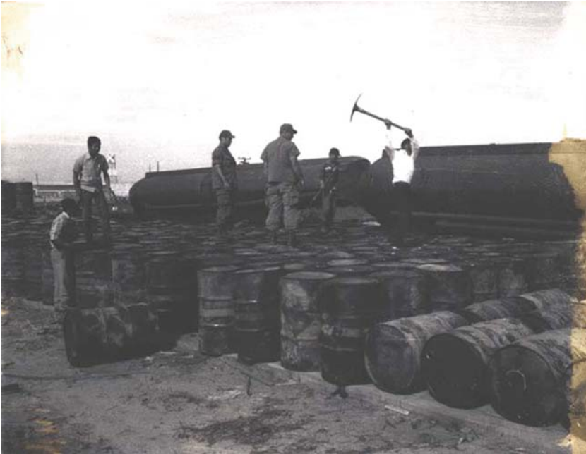
Fig. 4.9 Empty Agent Orange drums identified as non-reusable were further damaged by punching holes in the tops and bottoms, and then disposed of in a local landfill, Operation PACER IVY, Da Nang Air Field, 18 January 1972 (Carmichael Journal 1972)
