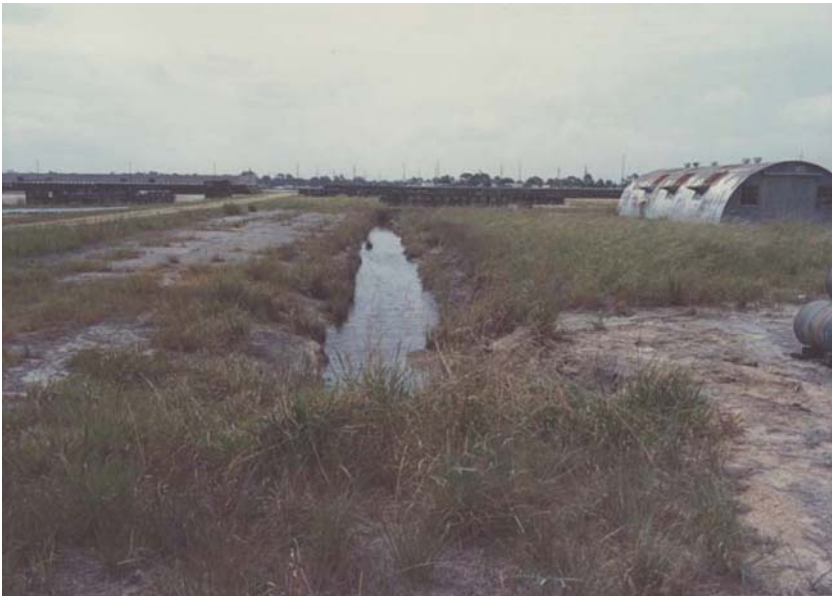
Fig. 7.6 A June 1975 photograph of part of the drainage system on the NCBC Herbicide Orange Storage Site. Herbicide residues were not found in the silt in the ditches or on the banks of the ditches (Photograph courtesy of A.L. Young)
