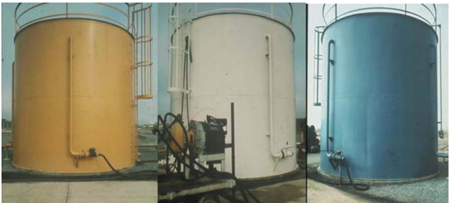
Fig. 3.14 Photographs of the 30,000-g (113,550-l) above ground tanks constructed at Bien Hoa Air Base in December 1969 for the temporary storage of Agents Orange, White, and Blue, respectively. Each tank was color-coded to identify the herbicide contained. (Photographs courtesy of J. Ray Frank, Frederick, Maryland)
