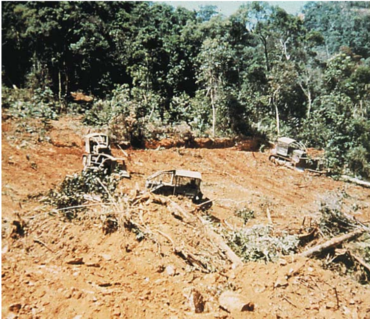
Fig. 3.27 A photograph of US Army Corps of Engineers using Rome plows to clear vegetation in III Corps, Vietnam (Photograph courtesy of J. Ray Frank, Frederick, Maryland)
