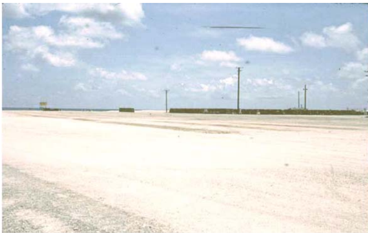
Fig. 4.39 A Photograph of the Johnston Island Agent Orange Storage Site taken on 1 September 1977 After completion of Operation PACER HO; In the background are the approximately 35,000 crushed drums prepared for shipment to a smelter; a residue monitoring program for the site was initiated on 25 August, 1977 (Photograph courtesy of USAF Occupational and Environmental Health Laboratory, Brooks AFB, Texas)
