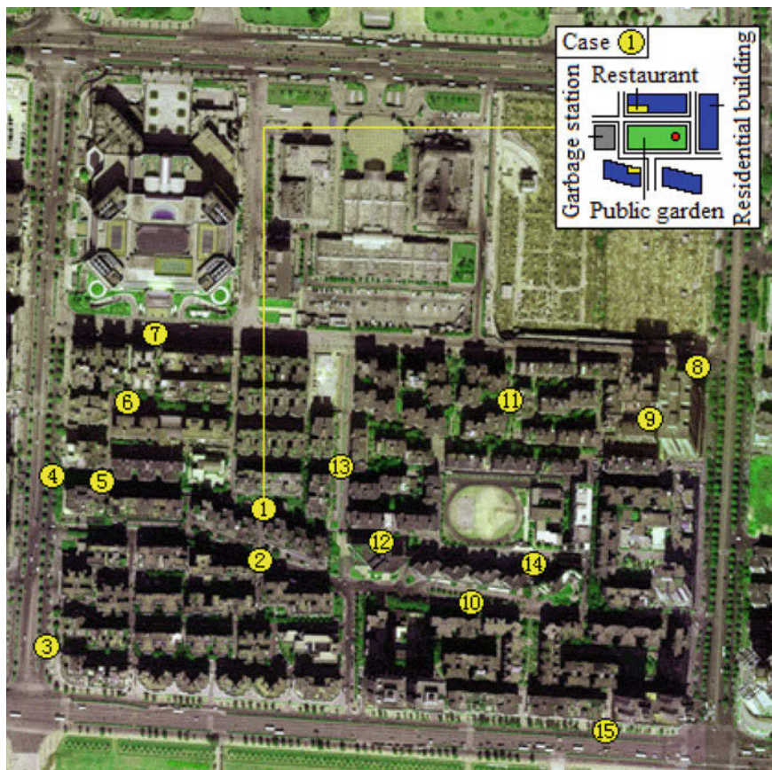
Fig. 19.1 Aerial view of the Tian-He-Nan residential area and the organization way of sound spaces (take case 1 as example)
