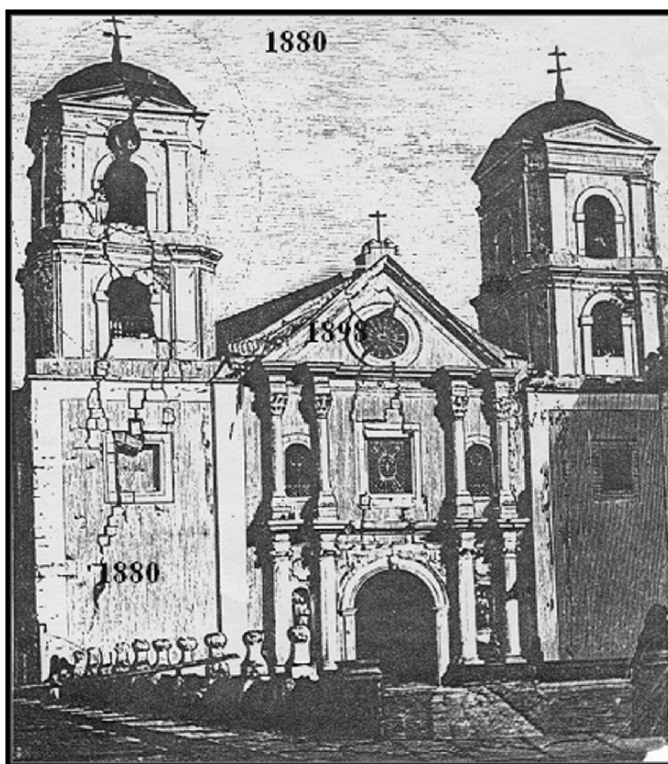
(b) past damage condition
