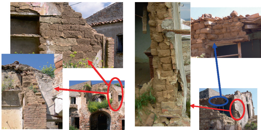
Fig. 4.5.6 Examples of adobe walls
