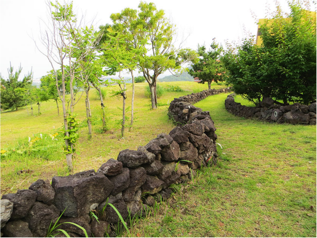
Fig. 2.29 Batdam (stone walls built from basaltic scoria boulders removed from adjacent soils) winding through the landscape of Jeju
