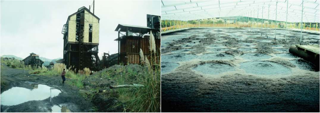
Fig. 9.22 An example of a contaminated site cleanup. Left: an abandoned industrial site in New Zealand with extensive hydrocarbon contamination. Right: biodegradation was enhanced by adding nutrients and oxygen to the material until a safe inert product was formed that could be incorporated into the soil at the site. The site is now a protected “historic place” due to its industrial history
