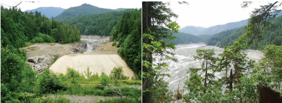
Fig. 3.24 The Elwha River in Western Washington State after dams were removed. Left: Site during removal of one of the dams in about 2012. Right: View of some of the sediments remaining after the dam was removed. An area of nearly 3 km 2 of new lake sediments was left after the dams were removed
