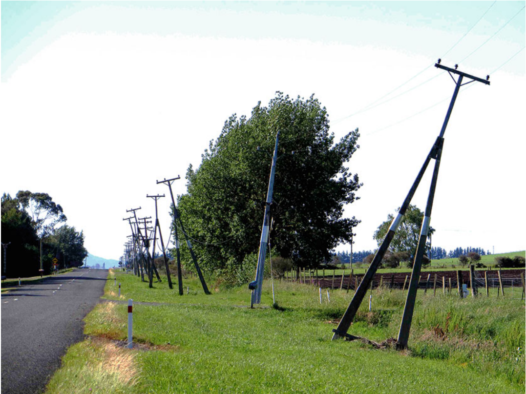
Fig. 3.21 Keeping power poles upright on peat soils is challenging. Even with extra support, the lack of coherence in the underlying organic soil material is evident to all
