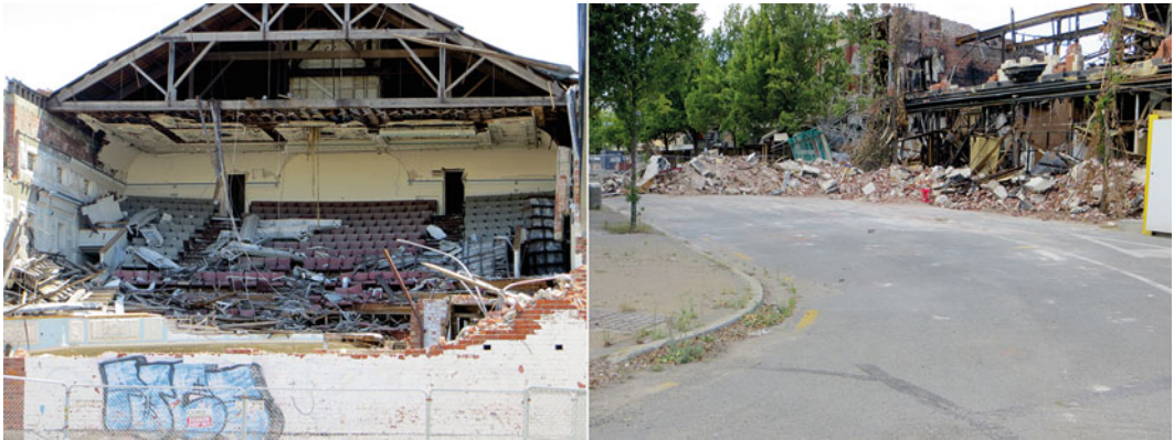
Fig. 7.7 Damage to buildings in Christchurch, New Zealand, caused by an earthquake in 2011
