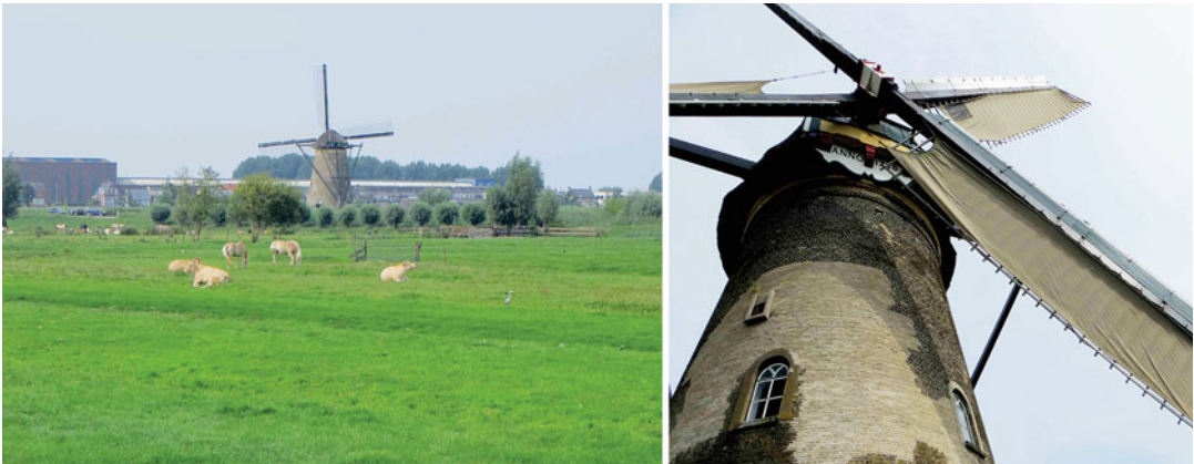
Fig. 9.27 Cows and horses graze pasture near Kinderdijk in the Netherlands where drainage works commenced about 800 years ago. Pumping water out over the dikes (using windmills from about 1740 until the mid-twentieth century) continues today
