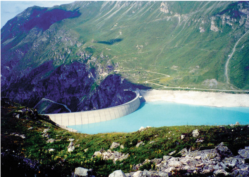
Fig. 3.23 A dam in the Swiss Alps. The pearly color of the water is due to the refraction of light by the high silt content of the water. Some of the silt will settle out and accumulate as sediment in the bottom of the dam
