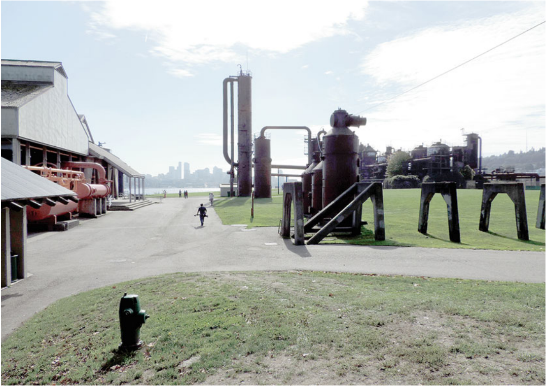
Fig. 8.31 Gas Works Park in Seattle, WA, USA, is an example of a contaminated soil on a site that was used to manufacture natural gas from coal and crude oil. Portions of the manufacturing plant remain in what is now a popular park. The contaminated soil has continued to be a problem and is being removed from the park
