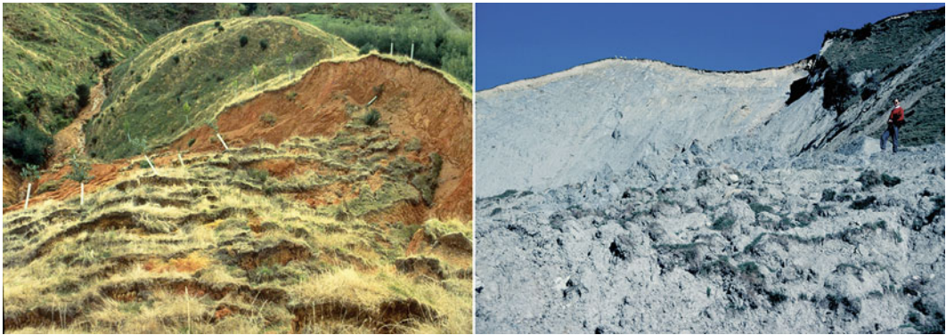
Fig. 7.15 Two examples of exposed shear planes from which the overlying material has slid. Mobilized, saturated soil flowed down to the streams far below
