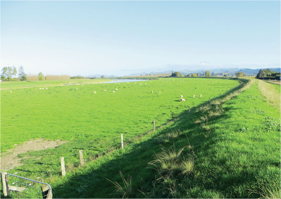
Fig. 3.10 Flood stopbanks protect farmland and other infrastructures on the floodplain of the Waipaoa River in New Zealand. Sheep graze the unprotected area inside the stopbank but can be readily moved if flooding is imminent. The protected area outside the flood stopbank is used for more intensive development such as cropping, vineyards, and housing
