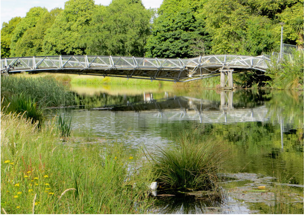
Fig. 7.9 The twisted remains of a footbridge after the 2011 Christchurch earthquake. The unsupported riverbanks collapsed inward as a result of the shaking damaging many bridges and water and sewer pipes
