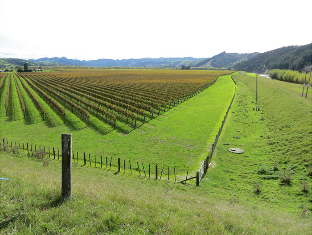
Fig. 3.31 A vineyard established on the floodplain of the Waipaoa River in New Zealand is protected by a flood stop bank. Twenty-five years earlier, a major cyclone deposited over 1 m of silt across this land surface
