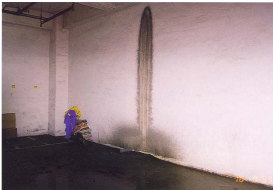
Fig. 2.2 Smear left on a building wall created by ejected sand during the 1999 M 7.5 Chi-Chi earthquake in Taiwan. Motorcycle at lower left shows scale (From Su et al., 2000)
