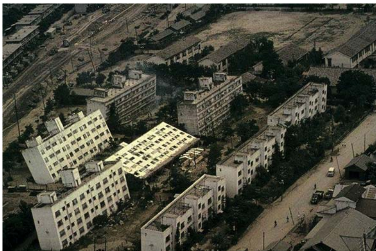
Fig. 2.4 Tilted apartment buildings after the Niigata earthquake. Despite the extreme tilting, the buildings themselves suffered remarkably little structural damage (From the Earthquake Engineering Research Center Library, University of California at Berkeley)
