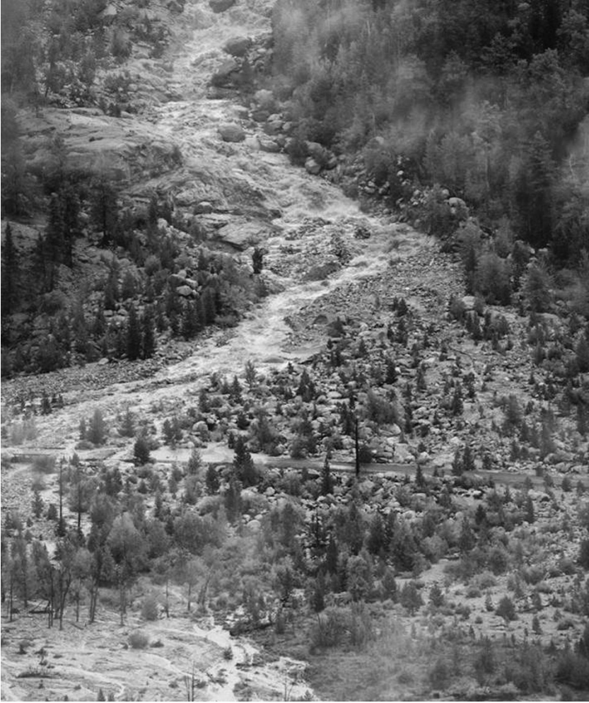
FIGURE 14-2 The September 2013 flood caused damage to roads, buildings, and other infrastructure in Rocky Mountain National Park. The road shown in this photo has since been replaced, with a large culvert now added that should withstand future flooding. (Photo from the Rocky Mountain National Park digital photo library, August 27, 2014.)
