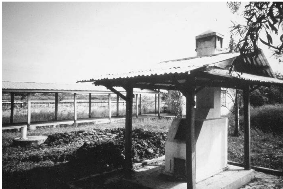
Fig. 8.3 Single-chamber incinerator
