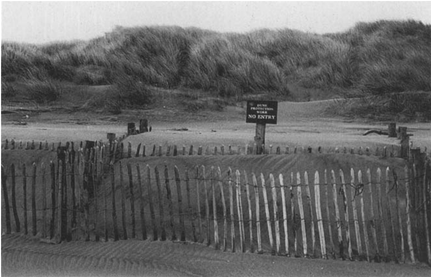
Fig. 9.14 Grid arrangement of chestnut paling fences, Sefton Coast, Merseyside, UK.
