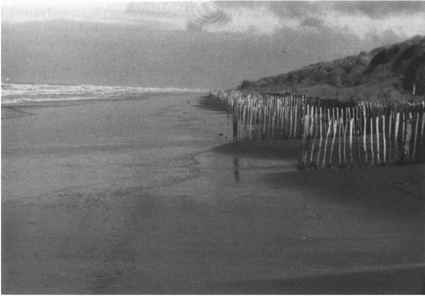
Fig. 9.13 Transverse slat-type fence and spur fences constructed of chestnut palings, Formby, Merseyside, UK
