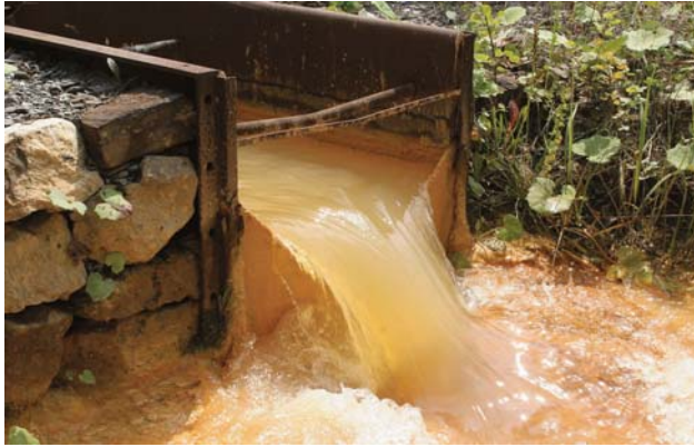
Fig. 49. V-notch weir measuring the flow of the Straßberg/Harz/Germany mine water treatment plant. Ochre precipitates are regularly removed from the weir plates.
