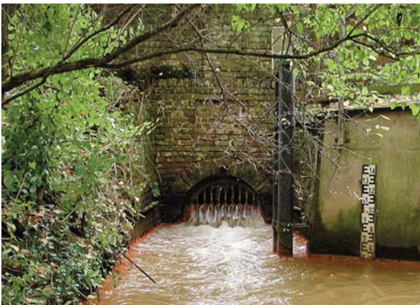
Fig. 11. The portal of the 7.5 km long German Burgfey/Eifel mine water adit discharging 15–19 m 3 min -1 of polluted mine water of the abandoned Mechernich mining area into the Veybach stream.
