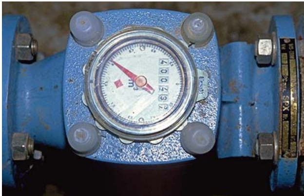
Fig. 59. Mechanical, propeller based water meter at the abandoned Dienststelle Marienthal bunker near Marienthal/Germany.
