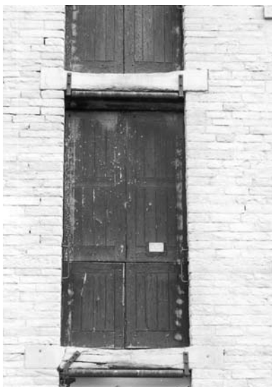
Figure 4.1 F Mill, Dean Clough, Halifax, 1858. Differential settlement to the front elevation is apparent in the form of cracks to the stone lintels across the full height loading bay doors. Note also the damage caused by the corrosion and expansion of iron fixings. (Stuart Millns)
