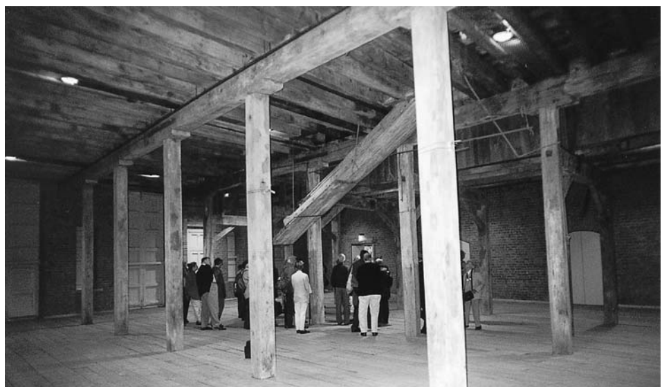
Figure 2.1 Liverpool Road Railway Station warehouse, Manchester. Built in 1830 and now a grade I listed building.
