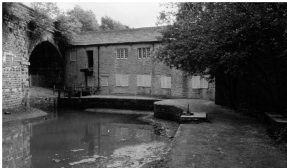
Figure 2.3 Higher Mill, Helmshore. Although built in 1790, the stone exterior, small windows and low rise of this mill are typical of pre industrial revolution water-powered mills.
