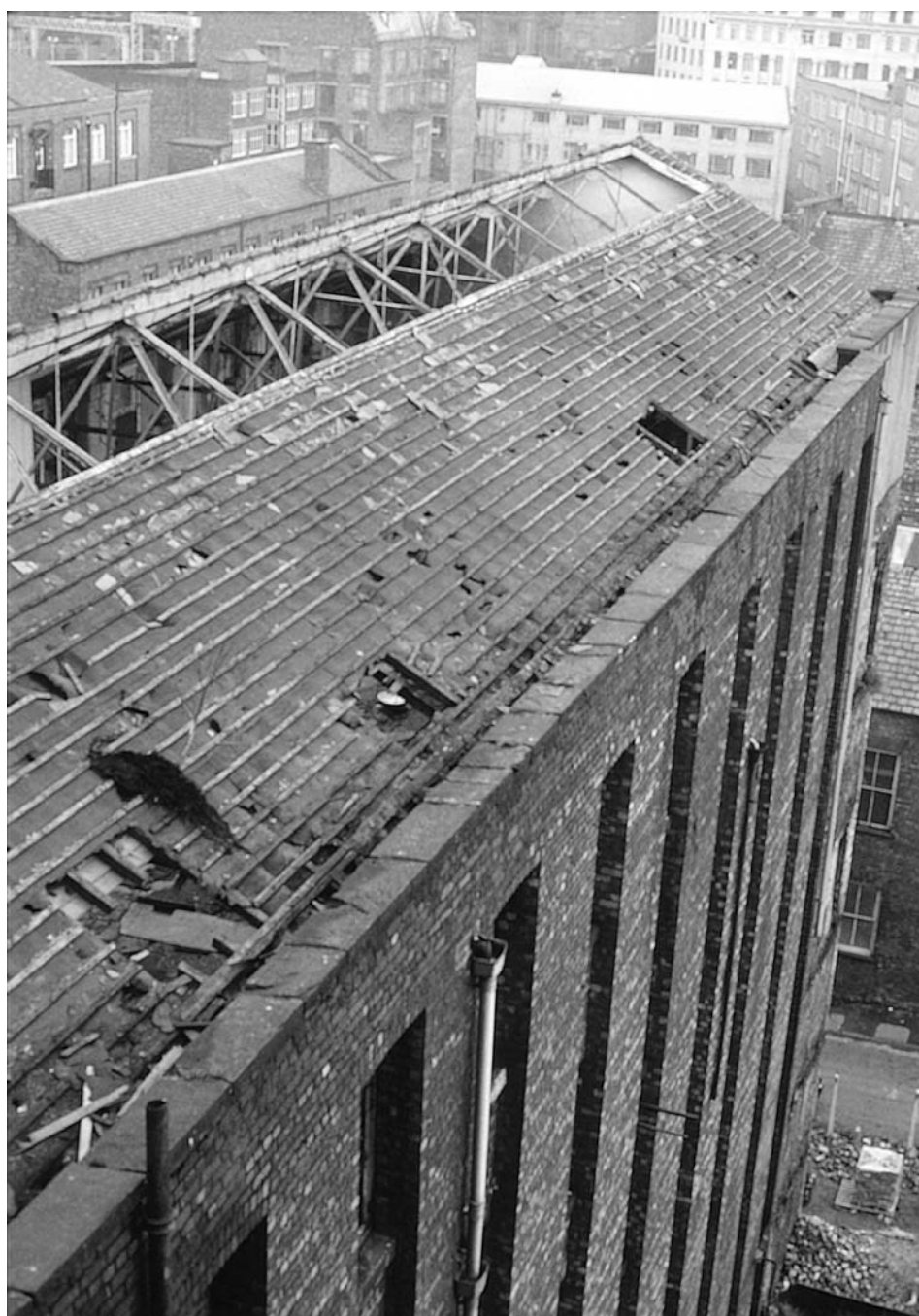
Figure 2.40 Chorlton Mills, Manchester. Built in c. 1803, the outer leaf to the mill is probably a late nineteenth-century addition.
