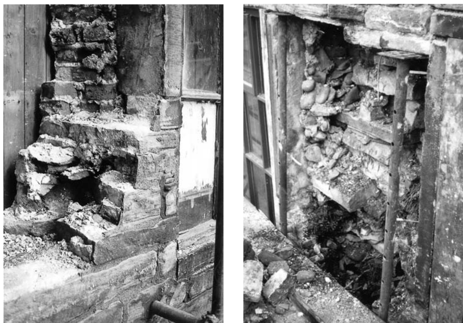
Figure 2.11 Cavity wall with rubble infill. Greenup's Worsted Mill, as previous figure. Cavity wall construction and window elongation. Note through-stones and part throughs with loose cavity rubble. Single leaf internal brickwork returns to stone jambs at window reveals. (Stuart Millns)
