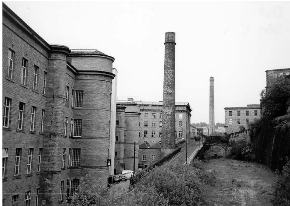
Figure 2.12 A Yorkshire industrial landscape – Dean Clough, Halifax. In the foreground is Bowling Mill, built c. 1840. The external stair and toilet towers maximize the floor space available for spinning machinery. Note the double stone lintels and good quality Yorkshire sandstone. (Stuart Milns)
