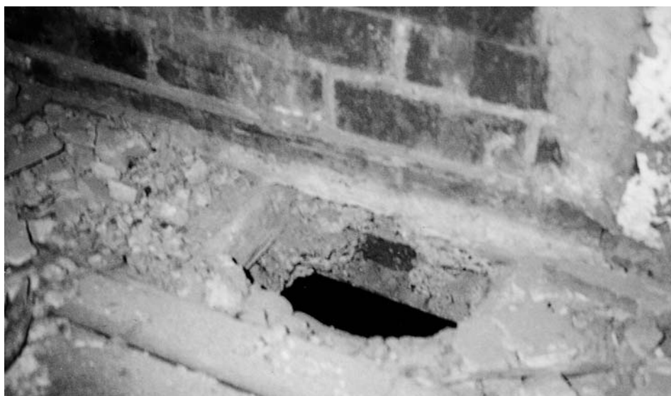
Figure 4.10 A 4 m brick wall built directly off a filler joist floor in the c. 1908 Rugby Mill, Chadderton, Oldham. The continuous wall arches between the primary steel beams. (Stuart Millns)
