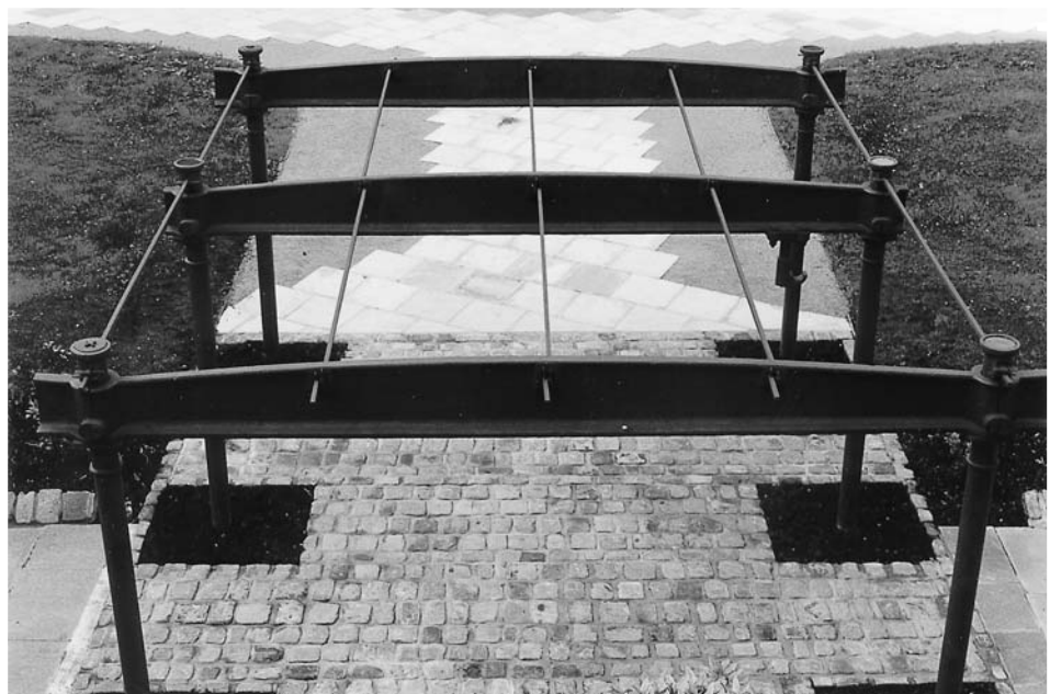
Figure 2.22 Havelock Cotton Mill iron framing (1845). As re-erected on the UMIST campus in 1997.
