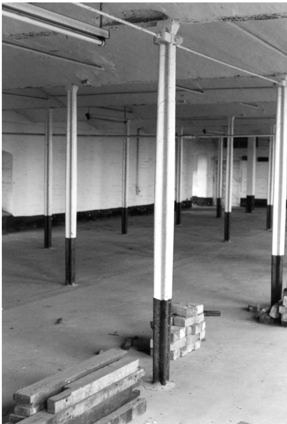
Figure 2.13 Cruciform column. in the 1797 Marshall, Benyon & Bage Flax Mill, Shrewsbury.
