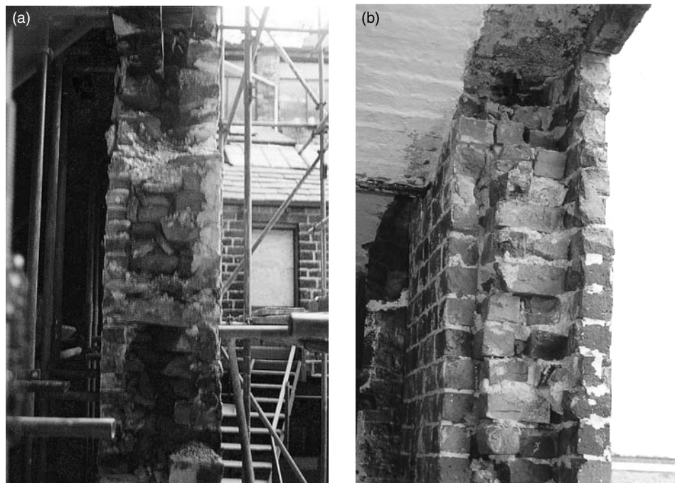
Figure 2.10 (a) Stone wall section, built c. 1791. Greenup's Worsted Mill, Sowerby Bridge Mills, is five storeys high with internal timber framing. (b) Brick wall section. (Stuart Millns)
