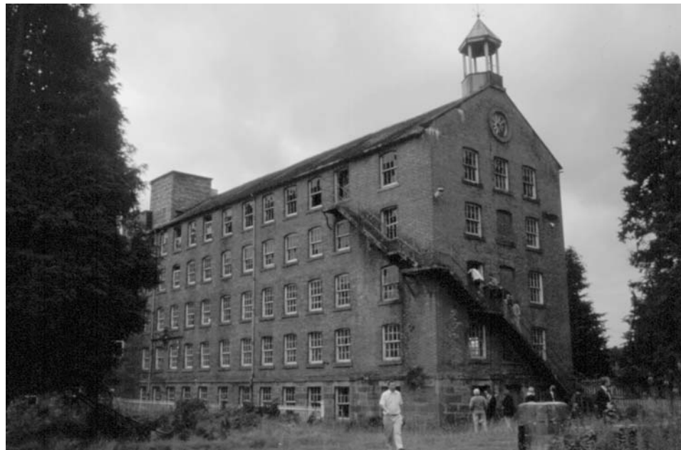
Figure 2.2 Bell Mill, Stanley, near Perth. Built c. 1787, a brick-built mill that exemplifies the long narrow floor plan of early Arkwright-type mills.
