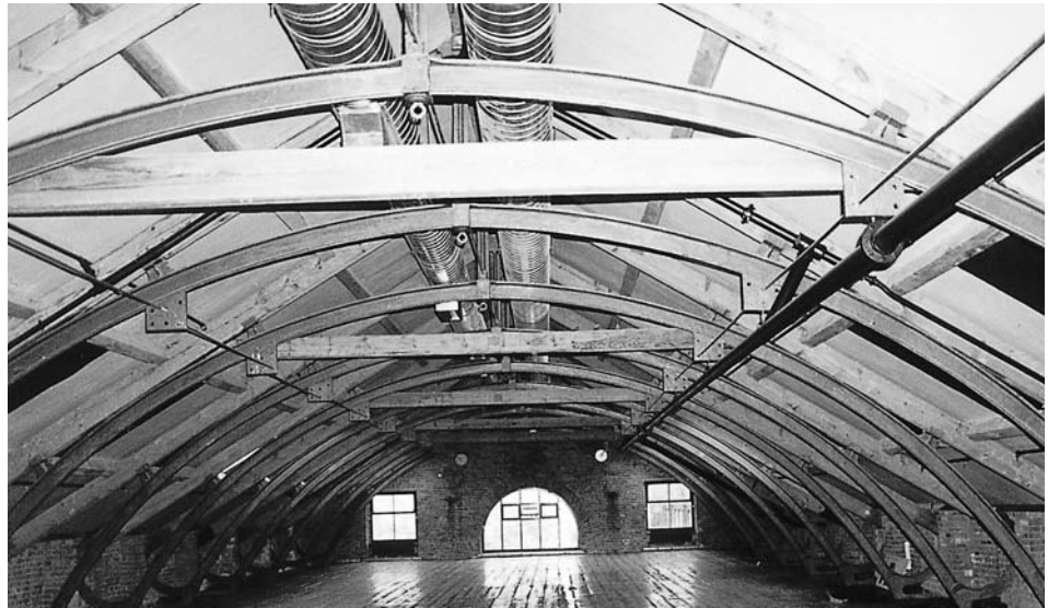
Figure 2.29 Cast-iron arched roof to part of Beehive Mill, Manchester (1825).
