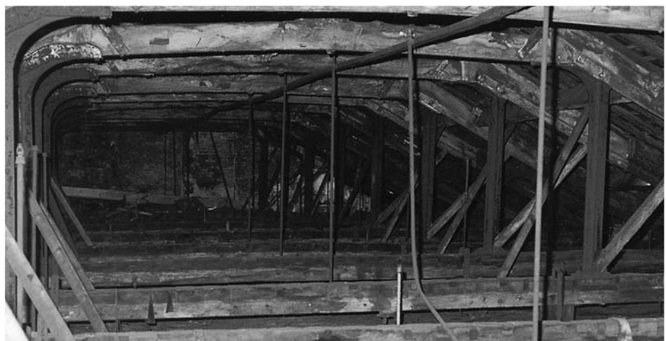
Figure 2.38 Floor removal in Bell Mill, Stanley, near Perth. Built in c. 1787 a complete floor removed about 100 years later.
