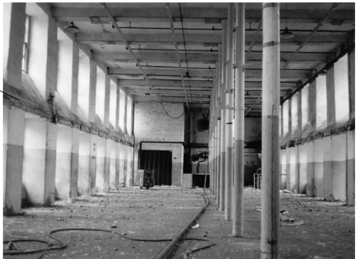
Figure 2.38 Floor removal in Bell Mill, Stanley, near Perth. Built in c. 1787 a complete floor removed about 100 years later.
