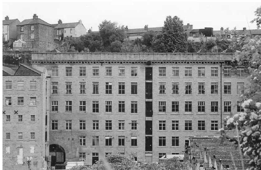
Figure 4.1 F Mill, Dean Clough, Halifax, 1858. Differential settlement to the front elevation is apparent in the form of cracks to the stone lintels across the full height loading bay doors. Note also the damage caused by the corrosion and expansion of iron fixings. (Stuart Millns)
