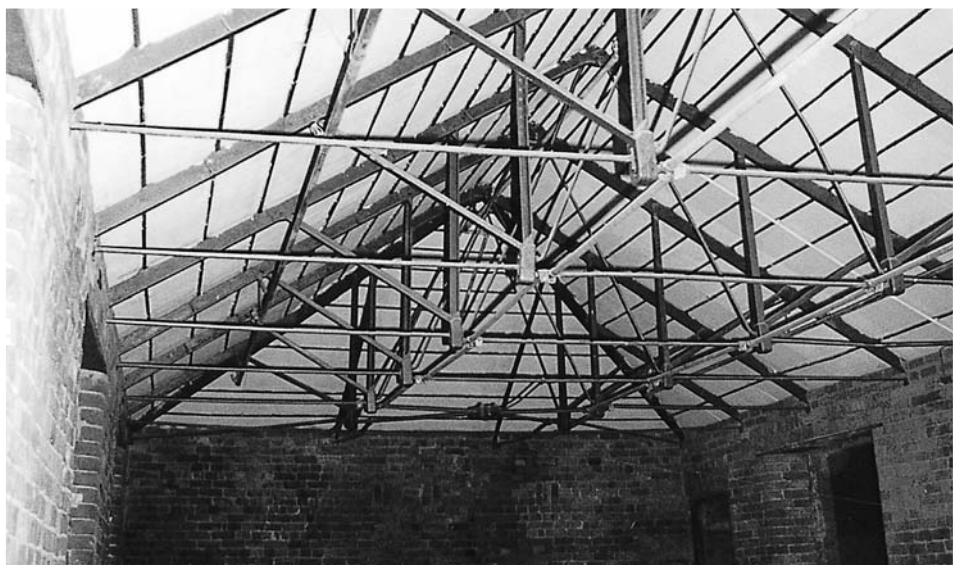
Figure 2.31 Trussed iron roof to part of Beehive Mill, Manchester (1824).
