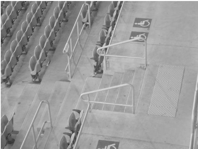
Figure 7.2 Integrated wheelchair seating and tactile ground surface indicators at Stadium Australia, the main stadium for the Sydney 2000 Olympic Stadium
