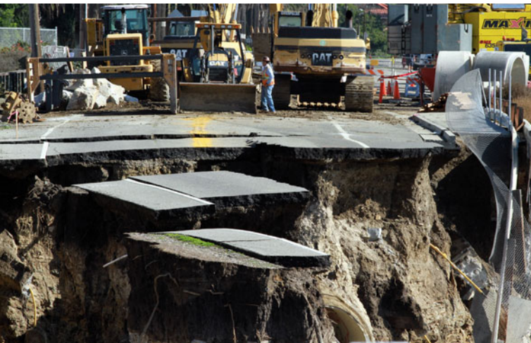
Fig. 1.2 Nov. 21, 2011—San Pedro, California, U.S.—A view of the scene after heavy weekend rains caused a portion of the cliffside and roadway on Paseo del Mar into collapse into the ocean in San Pedro, California. No one was hurt and no structures were damaged as a result of the slide. (Imaginechina)
