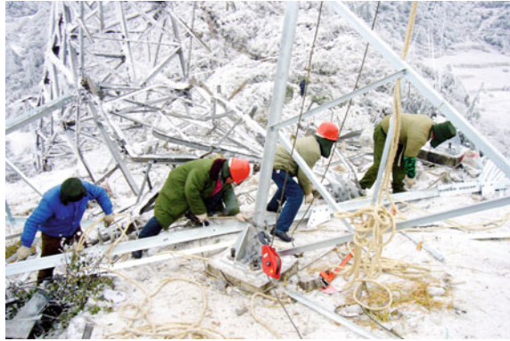
Fig. 11.1 Emergency repair of power grids collapsed in the snowstorm (Changmin Liu/Imaginechina)
