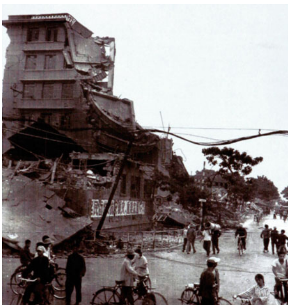
Fig. 10.2 Building collapse in the Tangshan Earthquake (Imaginechina)
