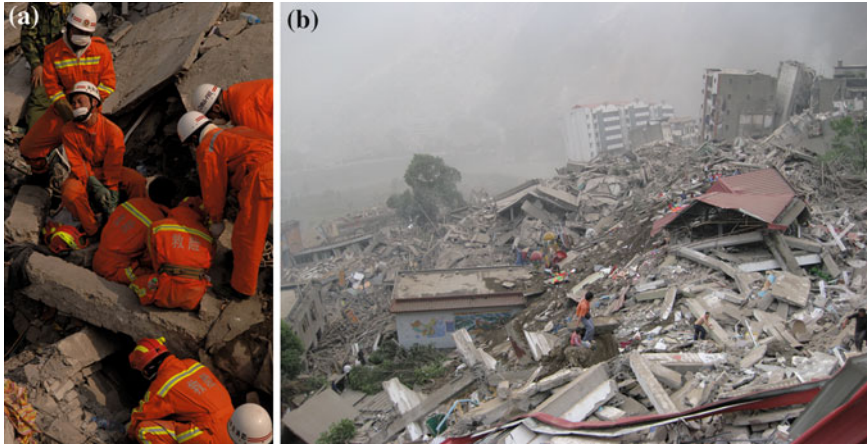
Fig. 6.1 Disaster scene of wenchuan earthquake. a Chinese firefighters search for quake survivors and victims in the rubble of collapsed houses after the May 12 earthquake in Yingxiu town, Wenchuan county, Aba Tibetan and Qiang Autonomous prefecture, southwest Chinas Sichuan province, 16 May 2008. (Chuanming Wu/Imaginechina) b Mess around Beichuan Earthquake area in the Wenchuan Earthquake. (Imaginechina)
