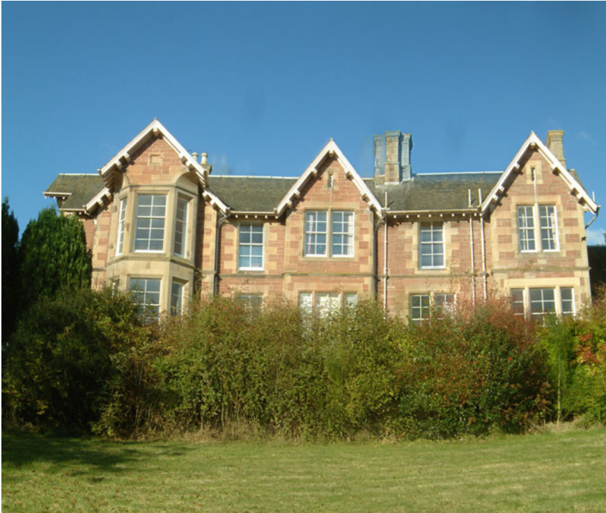
Fig. 5 Energy efficiency improvements on the nineteenth century mansion house in Alyth, Perth and Kinross [7]
