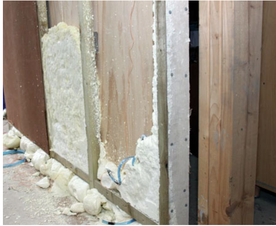
Fig. 8.5 Test installation of Icynene [4]
