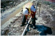
Photo 5 Injection pipe construction
