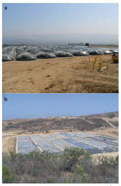
Figure 11.5. Full-scale *ex situ* soil bioremediation in (a) Ag-Bag<sup>®</sup> and (b) concrete containment cells (reprinted from Evans et al., 2008).
