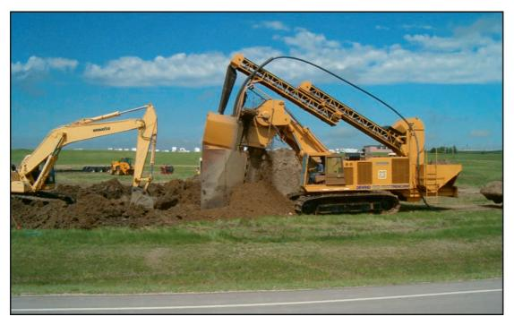
Figure 9.2. Continuous one-pass trencher in operation at Ellsworth Air Force Base, South Dakota (from AFCEE, 2008)
