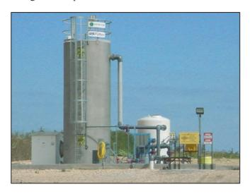
Figure 9.3 Ex situ bioreactor at NWIRP McGregor, McGregor, Texas (Photo courtesy of NAVFAC Southeast)
