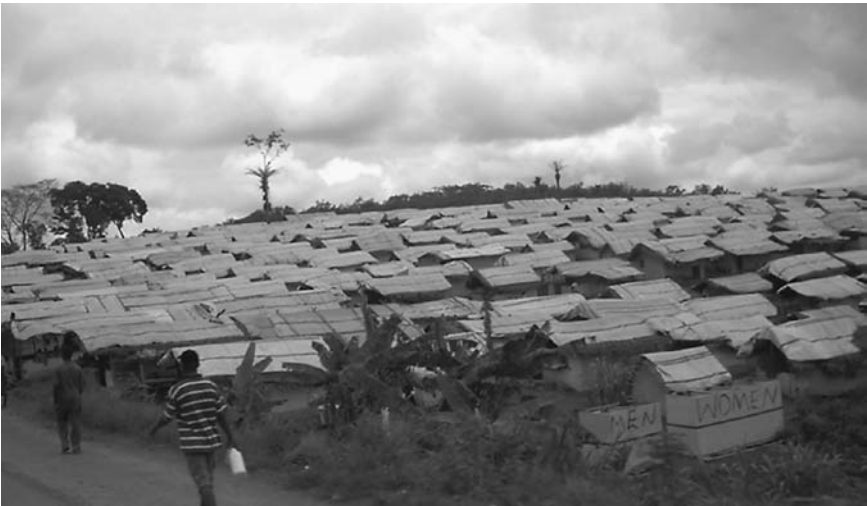
FIGURE 19-12 Physical design and spatial location of shelters in IDP camps, Salala District, Bong County, Liberia.
