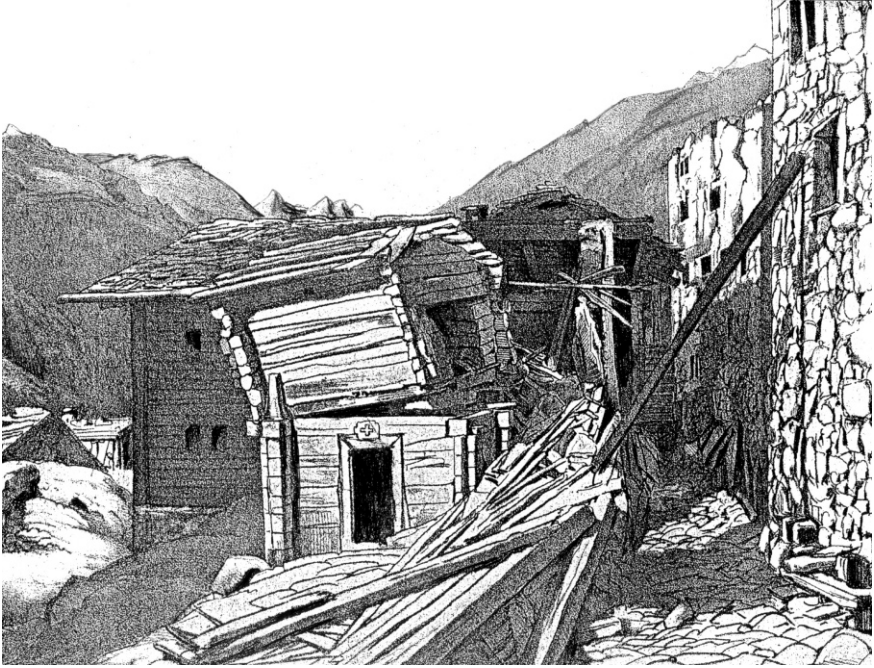
Fig. 3 Lithographic illustration showing heavily damaged stone house and timber structure in the Visp Valley. Heusser, 1856, ETHZ RARA: Geol P 173: 58 (1856)
