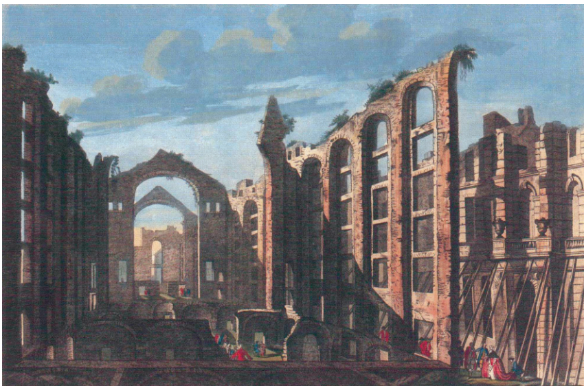
Fig. 16 Structure with slender walls without falling (Opera House or Real Theater) denoting damage caused essentially by the fire
