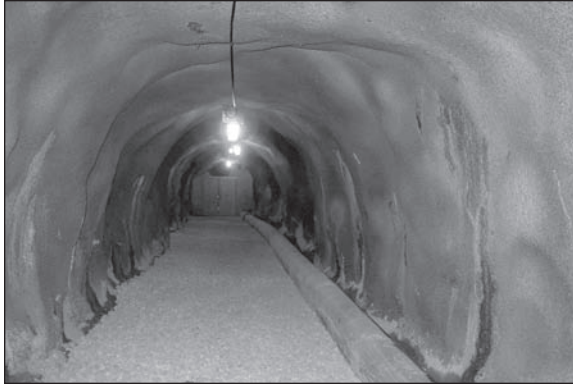
Figure 7. The finished Richmond Adit
