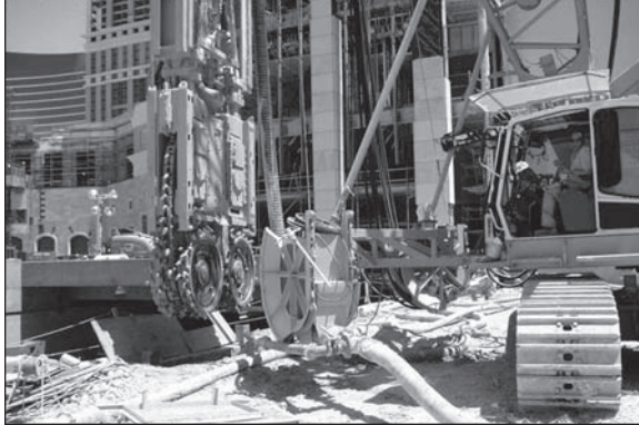
Figure 5. Typical slurry wall hydromill rig
