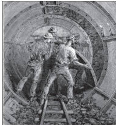
Erecting the Segments
