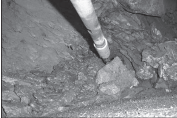
Figure 14. Picture of the drilling rods from the cavity on top of the shield
