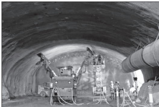
Figure 4. Tamrock Minimatic two boom jumbo drill in action
