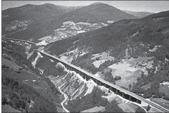
Figure 1. Liesertal Bridge on A10
