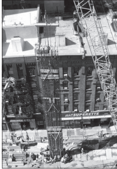
Figure 3. Slurry wall reinforcement cage lift
