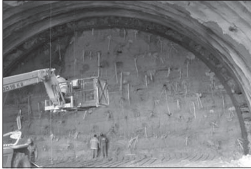
Figure 36. Cassia 1 tunnel: Jet-grouting columns in the core reinforced with fiberglass elements
