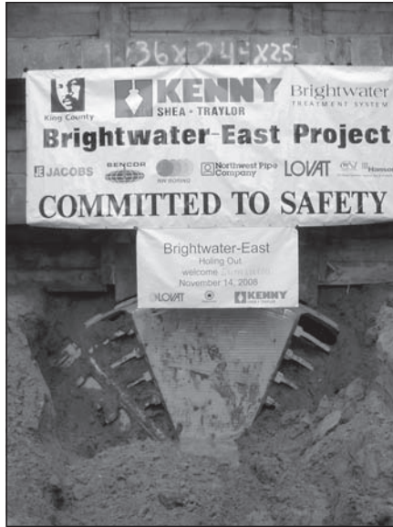
Figure 9. TBM holing-out at the TPP shaft
