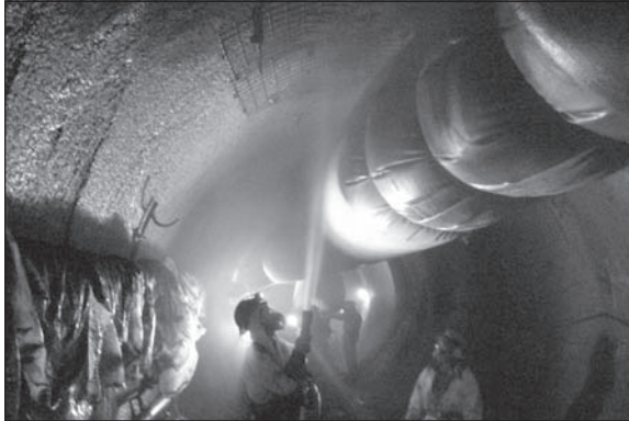
Figure 9. Final support as shotcreting
