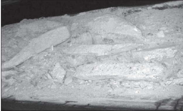
Figure 27. TBM excavation material from the Piora
