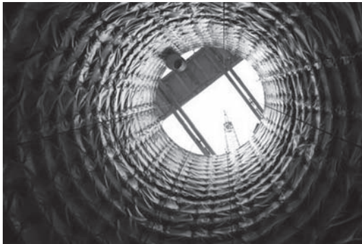
Figure 8. Installed PVC liner
