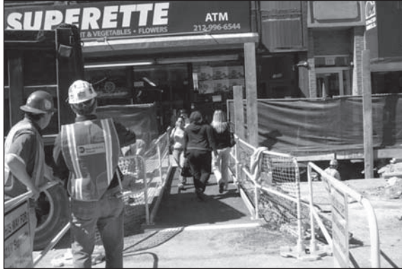
Figure 4. Maintaining access to businesses and pedestrians
