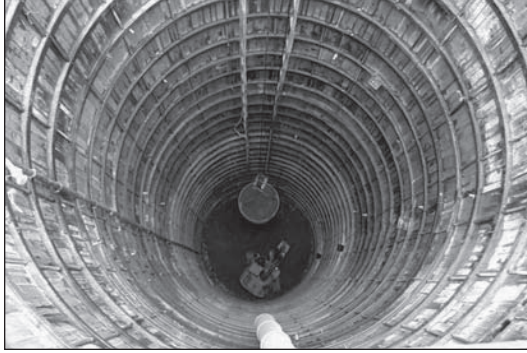
Figure 7. Deep excavation underway within the steel set liner
