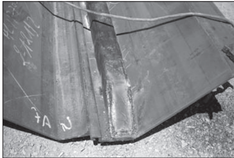
Figure 4. Outer inclinometer casing prior to sheet pile installation
