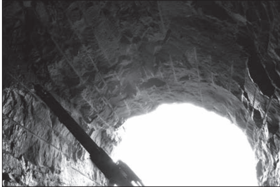
Figure 5. Photo of rock in the portal entrance
