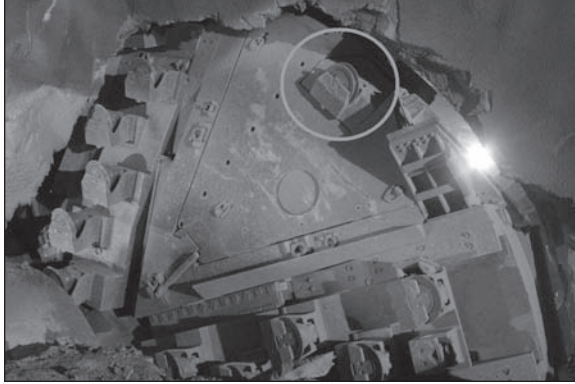
Figure 19. Overbreak roller bit on the TBE cutterhead
