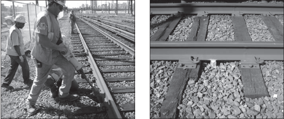
Figure 5. Field demonstration of installation of Track Dynamic Profile monitoring points
