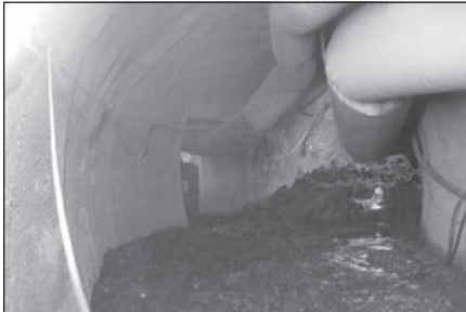
Figure 11. Extruding mud in the Exploratory Adit
