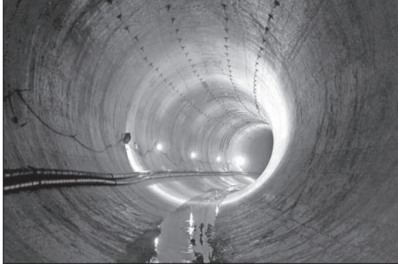
Figure 4. Thorn Creek diversion tunnel
