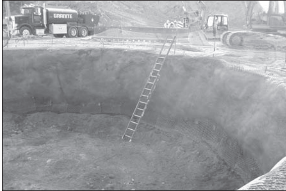
Figure 6. Initial excavation for shaft collar
