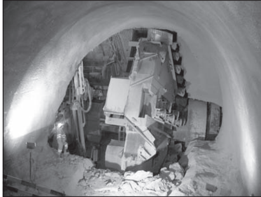
Figure 18. TBE-cutterhead passing an accessible cross-passage
