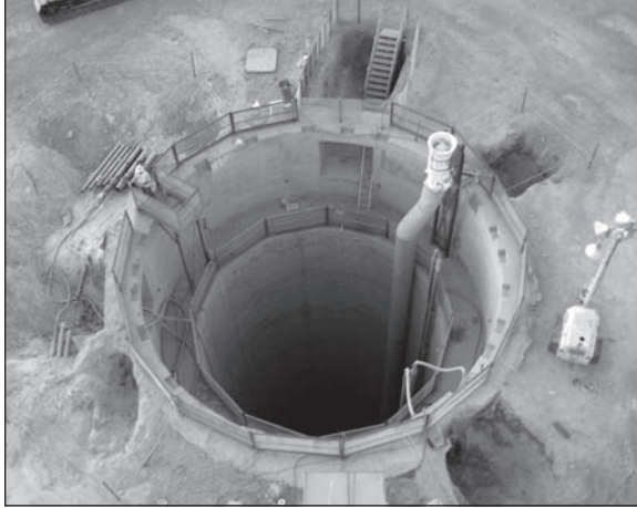
Figure 7. Completed shaft collar
