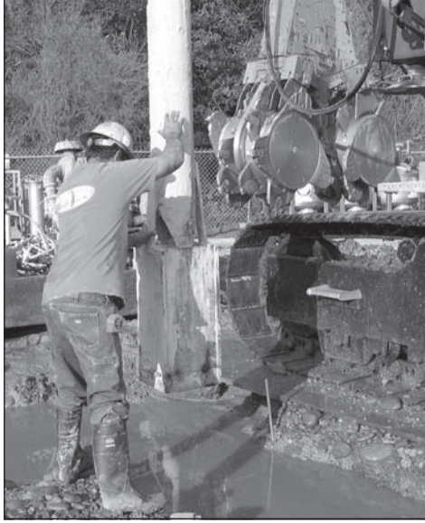
Figure 8. Drill Tech taking a sample from a CSM panel
