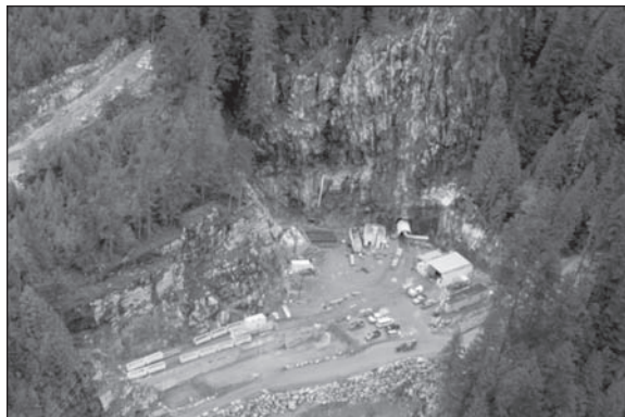
Figure 4. Portal rock stabilization
