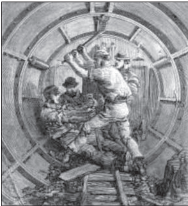
Advancing the Shield
