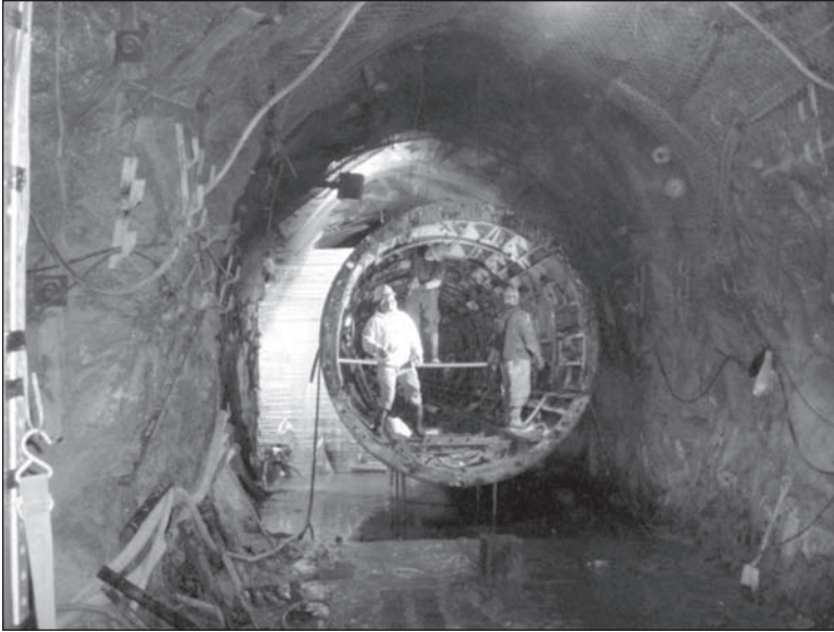
Figure 10. 3.05 meter (10 foot) diameter formwork in the East Starter Tunnel
