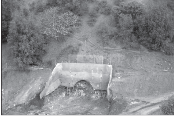
Figure 4. Development of tunnel portal
