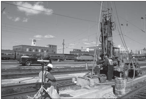
Figure 3. Subsurface exploration drilling in Sunnyside yard
