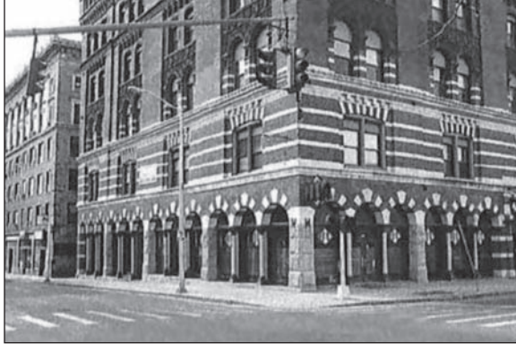
Figure 8. Historic buildings along alignment in downtown Hartford, Connecticut
