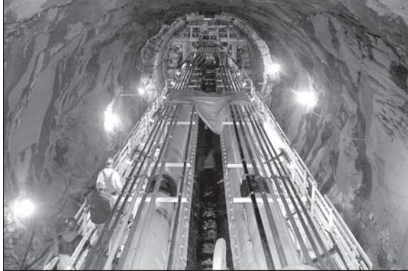
Figure 2. TBM in starter tunnel
