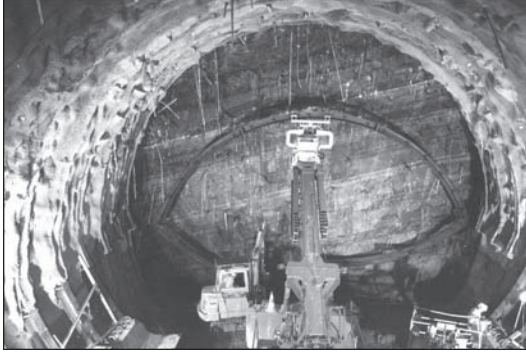
Figure 31. Tartaguille tunnel: Erection of a steel rib. After Lunardi (2008).
