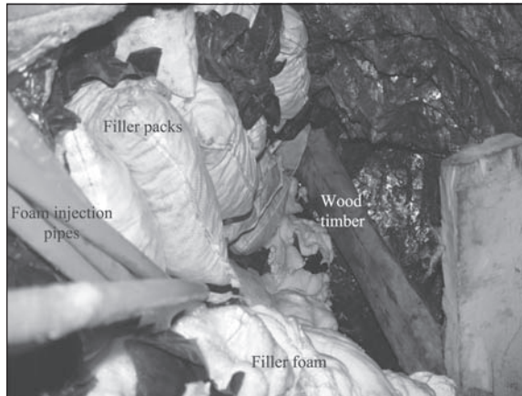
Figure 13. Filling cavities above the front shield by filler packs and foam
