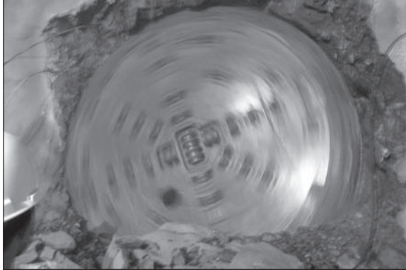
Figure 14. Breakthrough of the TBM
