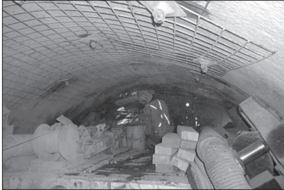
Figure 12. Typical tunnel support
