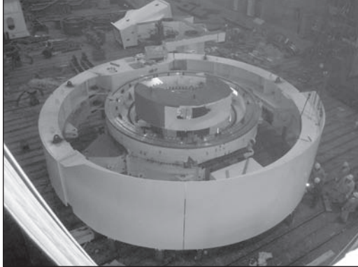
Figure 4. Partial shop assembly
