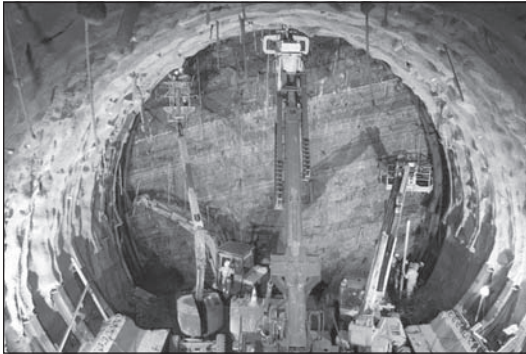
Figure 32. Tartaguille tunnel: The steel rib is erected. After Lunardi (2008).
