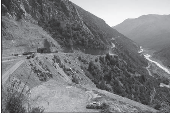
Figure 7. Intermediate access adit for long tunnel
