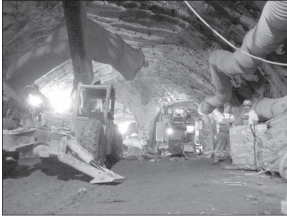
Figure 10. View showing GCT 3 Wye Cavern excavation
