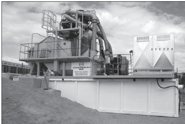
Figure 3. MTBM slurry separation plant
