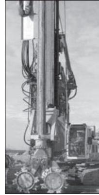
Figure 6. CDSM mixing rig
