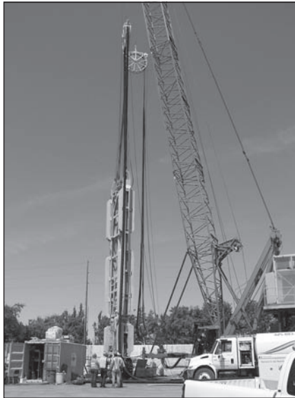
Figure 6. Start of the slurry wall operation at the IS shaft
