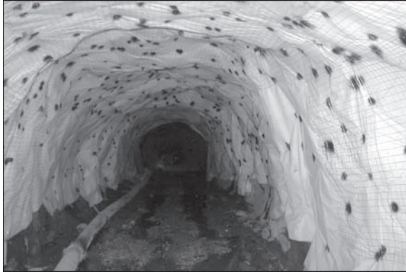
Figure 6. Drainage blanket
