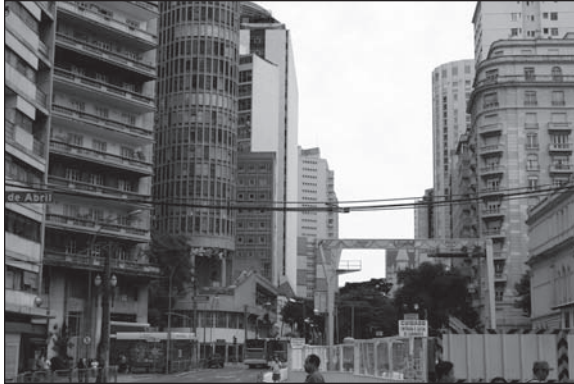
Figure 1. Dense populated area—view from site installation
