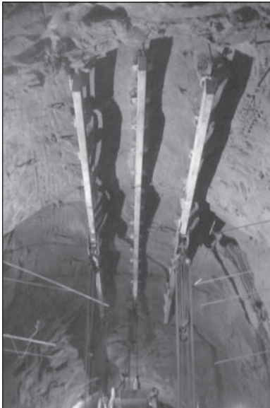
Figure 26. Monorails in the assembly chamber
