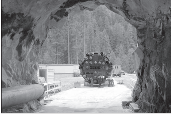
Figure 1. Small size TBM tunnel
