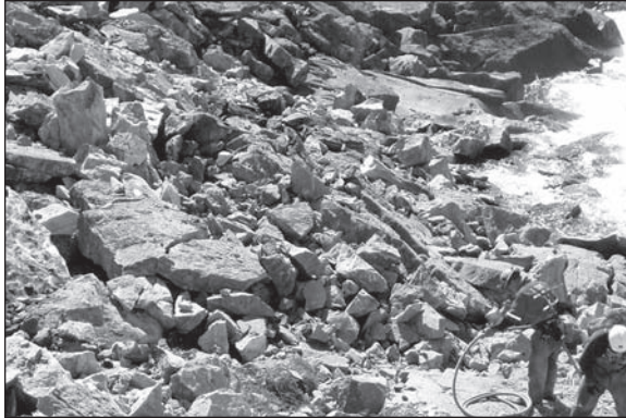
Figure 2. Clearing a landing site using handheld equipment
