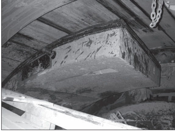
Figure 3. Segment being installed
