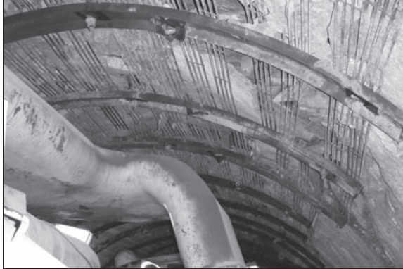
Figure 4. McNally TBM Support System™
