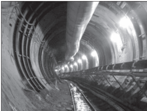
Figure 9. View Showing TBM mined tunnel
