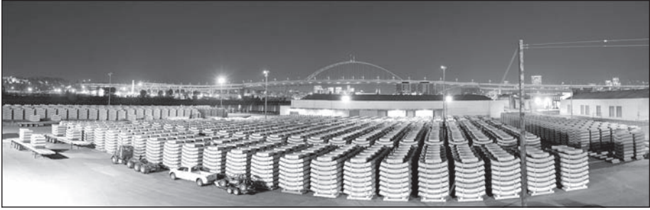
Figure 13. Segment storage of the ESCSO project
