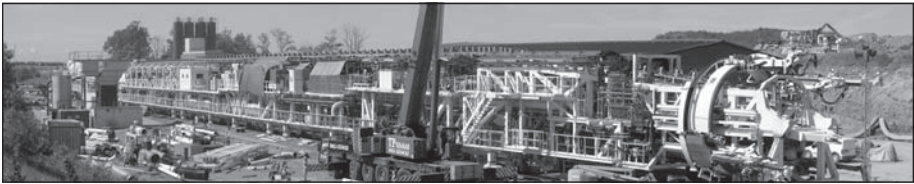
Figure 8. Trailing gear in front of the tunnel portal
