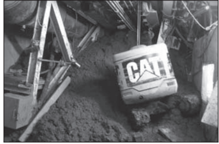
Figure 14. Extruding mud filling the Back-Up
