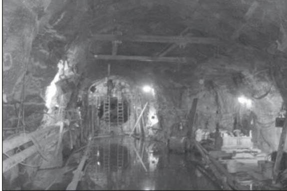
Figure 6. East starter tunnel with transformer pocket
