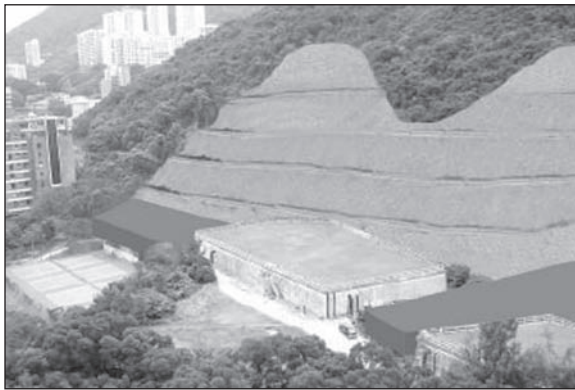
Figure 5. Photomontage showing general view of the open-cut alternative with large cut slopes and new water reservoirs (new water reservoirs highlighted for identification purposes only).
