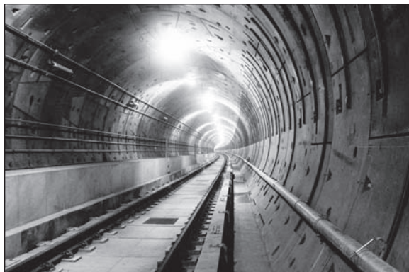
Figure 7. Tapered ring—Sheppard Subway
