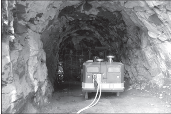
Figure 5. Drill and blast starter tunnel
