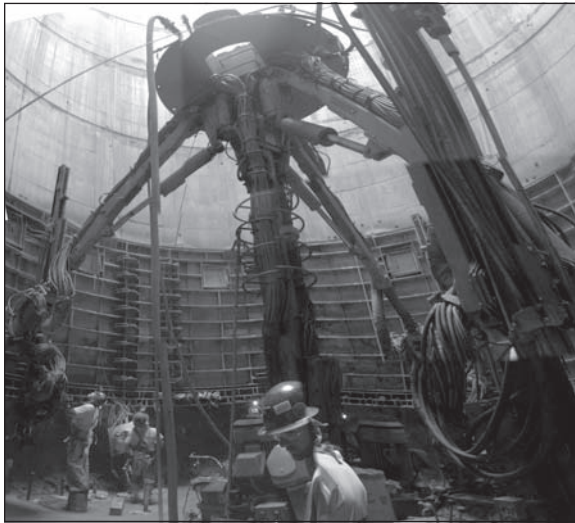
Figure 8. Tamrock Shaft Jumbo
