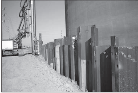
Figure 3. Progressive vibratory installation of sheet piles at the reservoir
