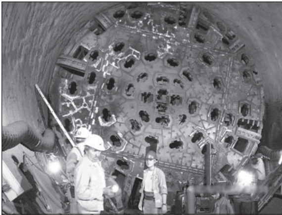
Figure 29. TBM cutterhead revision
