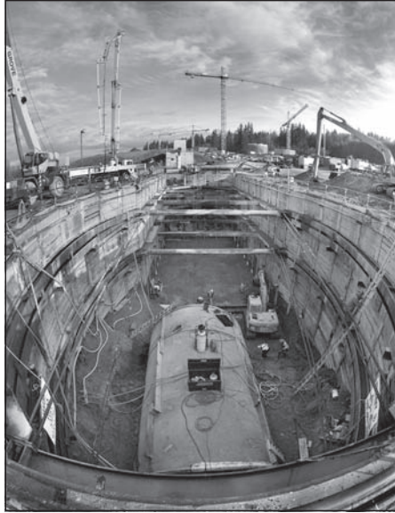
Figure 8. Treatment plant portal (TPP) shaft
