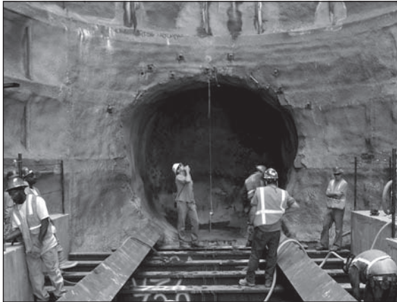
Figure 5. Central shaft excavation
