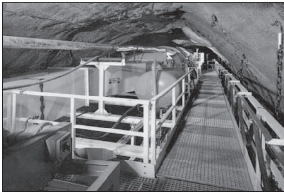
Figure 12. Hanging platform—bolt and chain supporting the rails to the right
