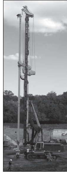
Figure 5. The Bauer CSM rig
