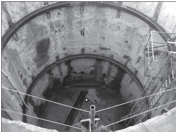
Figure 11. The completed south shaft
