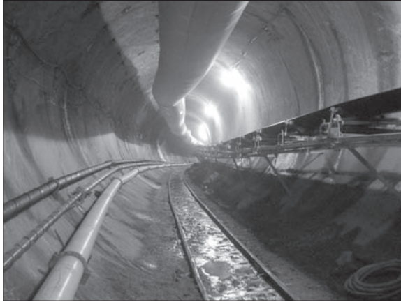
Figure 8. View showing TBM tunnel with ring steel ground support
