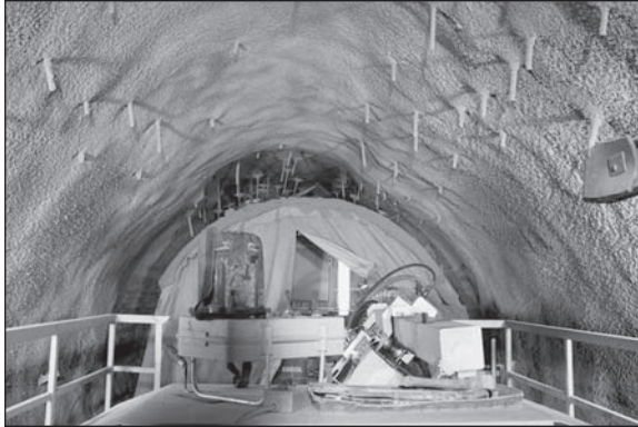
Figure 11. TBM-Excavation of the pilot tunnel
