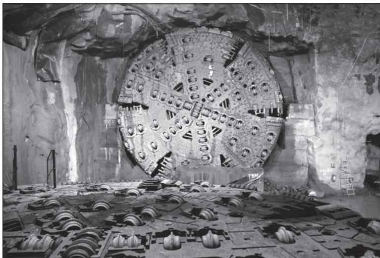
Figure 21. TBM arriving at mid-adit in April 2008 with the second cutterhead waiting in front
