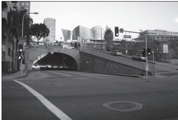
Figure 14. 2nd Street Tunnel, East Portal
