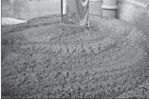
Figure 2. Conditioned muck at disposal area
