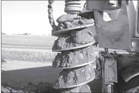
Figure 3. Large diameter flight auger in cobble laden ground
