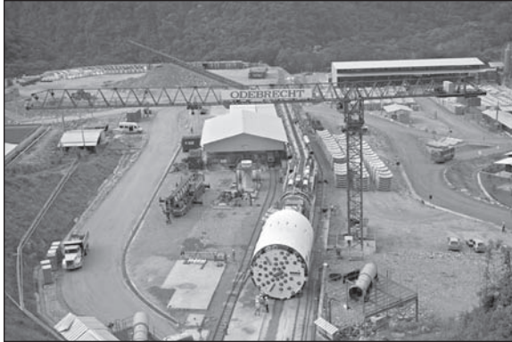
Figure 3. San Francisco TBM portal set up
