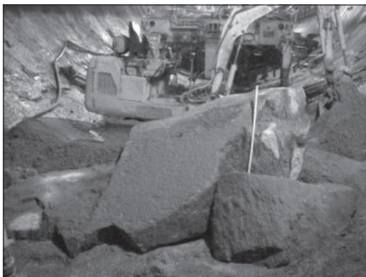
Figure 10. Caving in the L1*
