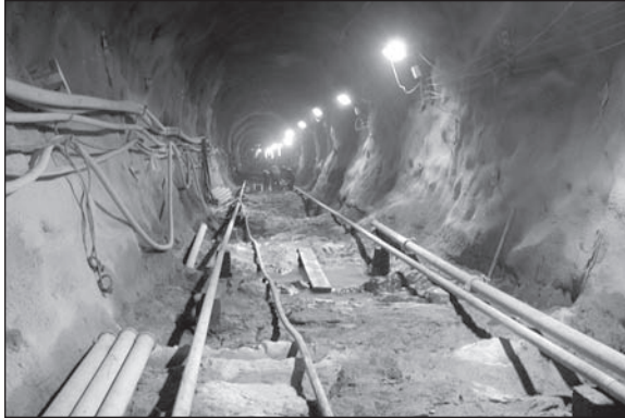
Figure 10. Concrete invert works for D&B tunnel
