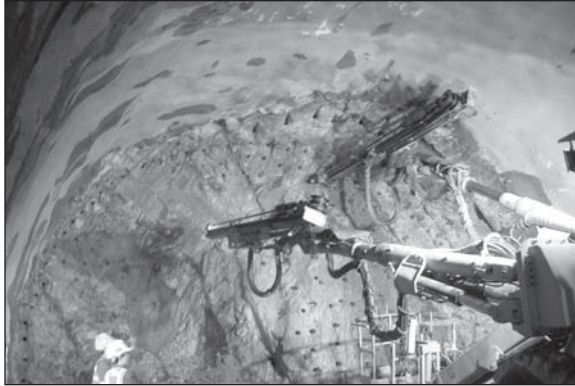
Figure 12. Drilling with the jumbo
