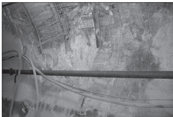
Figure 8. Fault F2 conditions
