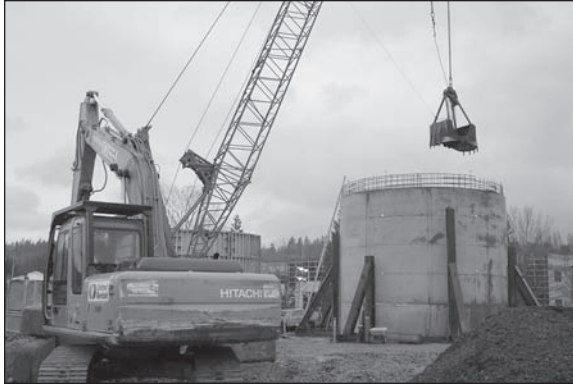
Figure 5. Manhole 1 caisson operation
