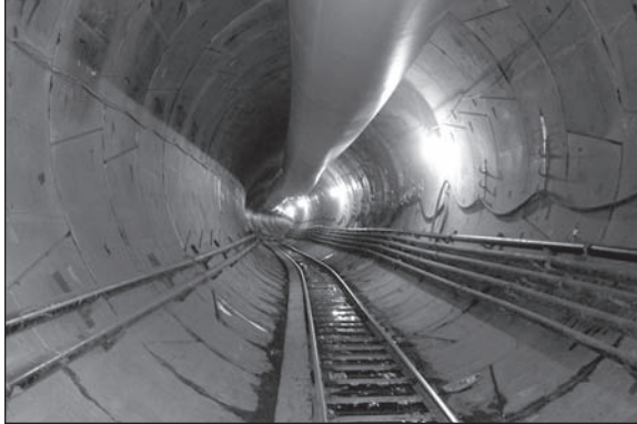
Figure 4. Segments installed in the tunnel
