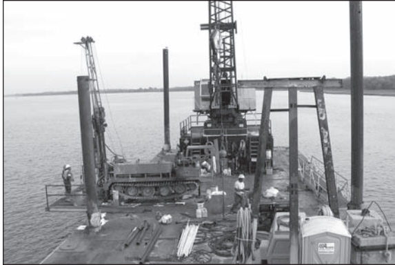
Figure 7. Photo of river boring from barge
