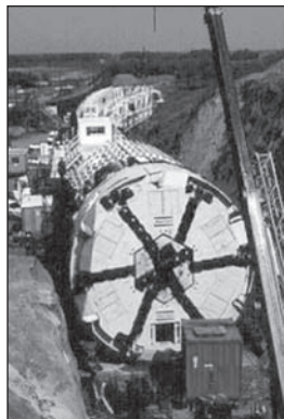
Figure 1. First attempt, grripper TBM “Hallborr” ready to go
