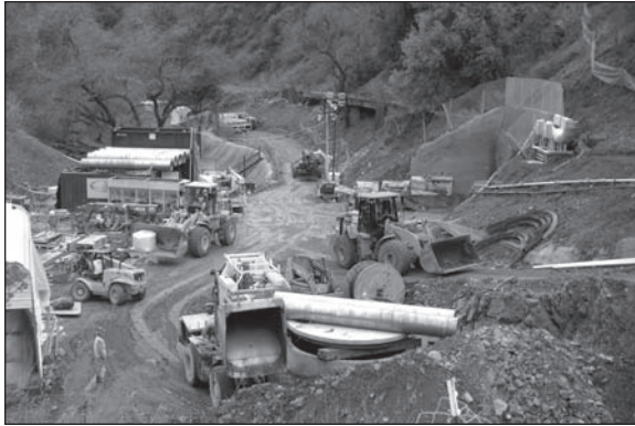
Figure 5. Portal area during mining activities
