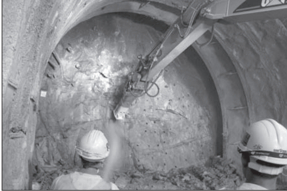
Figure 10. Excavation using mechanical breaker for the initial tunnel
