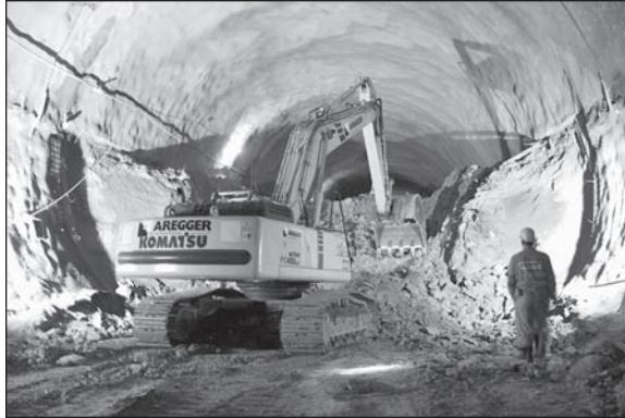
Figure 10. Excavation of the Eichholz molasse section
