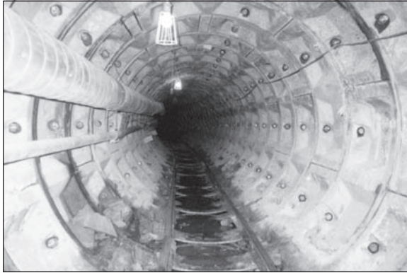
Figure 4. Standard bolted segmental liner
