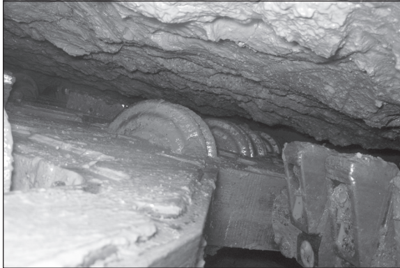
Figure 8. Mix-Shield cutter head tools during inspection stop
