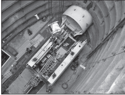
Figure 12. Shaft shield assembly
