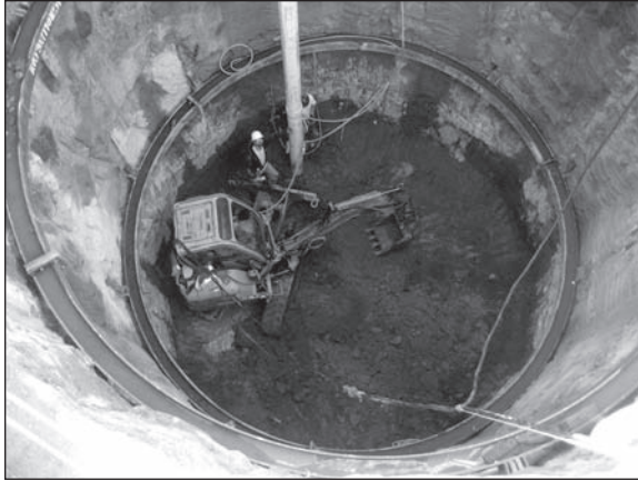
Figure 10. Excavation at the north shaft
