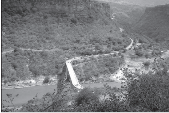
Figure 13. Nile bridge crossing
