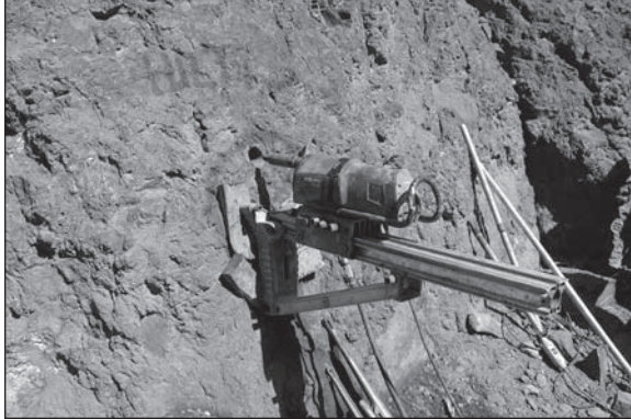
Figure 12. Hilti-drilling into outcrop
