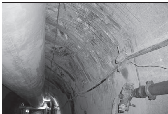
Figure 11. Support for overstressed conditions
