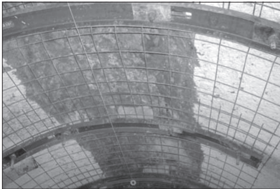
Figure 9. Modified ground support with channel
