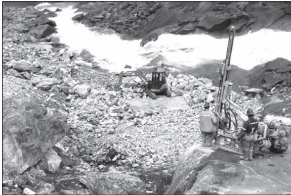
Figure 3. Small excavator and air track drill used to establish portal site
