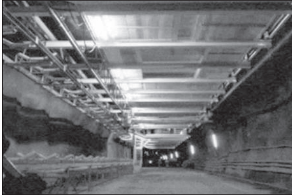
Figure 13. Platform from below—tunnel conveyor on the floor to the left
