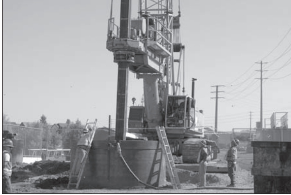
Figure 8. Shaft drilling setup
