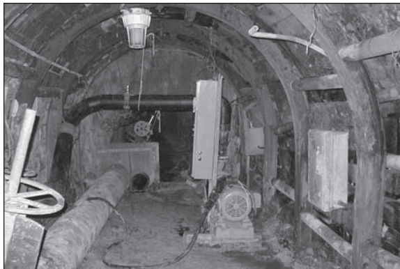
Figure 3. Scott Fault Bunker from the Richmond Adit
