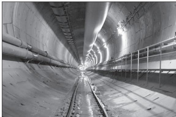
Figure 23. Lined tunnel
