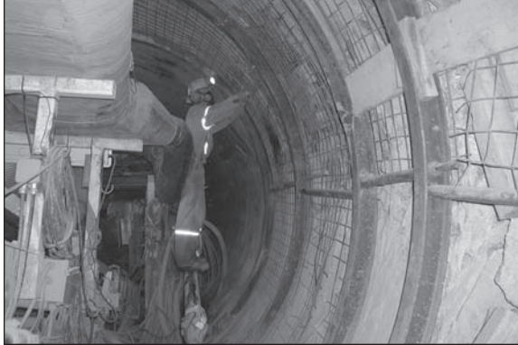
Figure 8. Support Installation in small TBM tunnel
