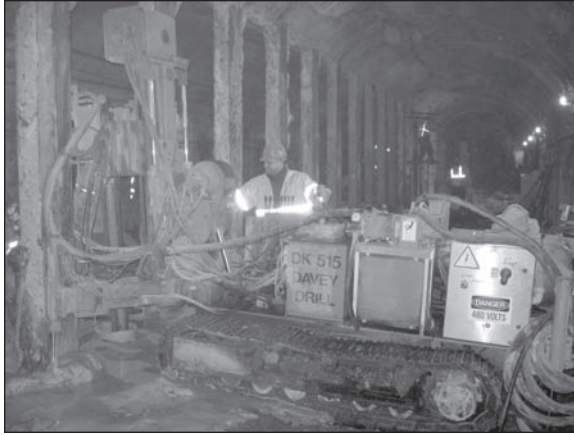
Figure 9. Installation of small diameter caissons with Davey DK 515 down-the-hole hammer
