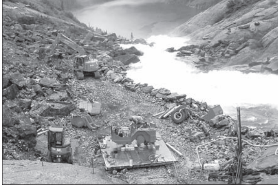
Figure 4. Larger equipment arriving to site
