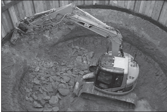
Figure 4. Excavation of frozen ground underway with hoe ram
