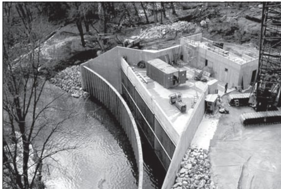
Figure 3. Thorn Creek diversion structure
