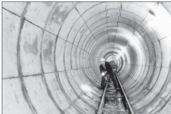
Figure 5. Wedge block liner
