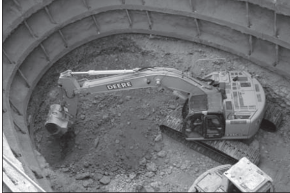
Figure 5. Central shaft excavation
