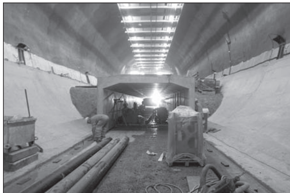
Figure 21. Service duct and backfilling behind the TBE
