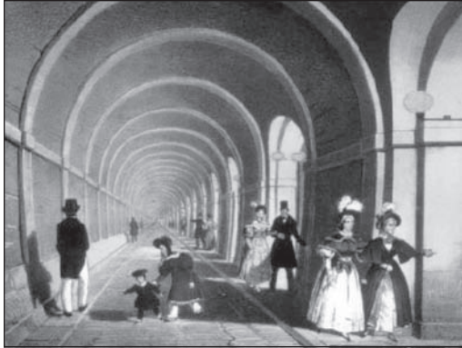
Figure 39. Opening of the tunnel under the Tames in the early 1800s, when sequential excavation was conceived
