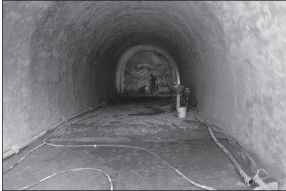
Figure 10. Tryon Street tunnel after spraying waterproofing on sides and arch
