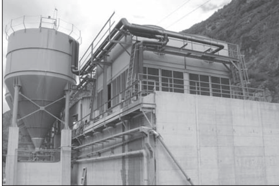
Figure 19. Construction site at Bodio, treatment of wastewater from the tunnel
