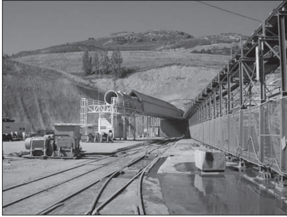
Figure 1. Access ramp tunnel portal
