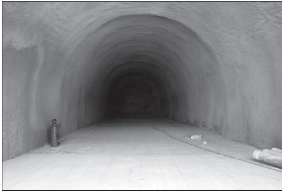
Figure 11. Tryon Street tunnel after pouring floor slab
