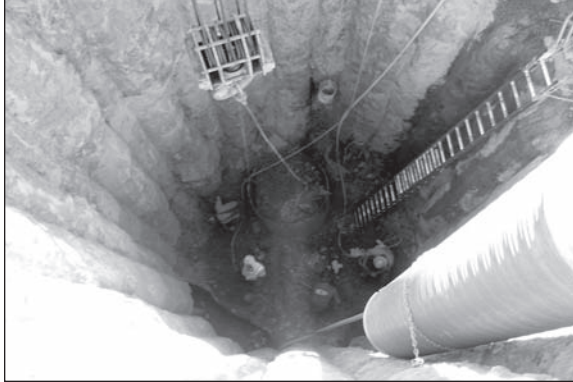
Figure 8. Shaft excavation by hand mining
