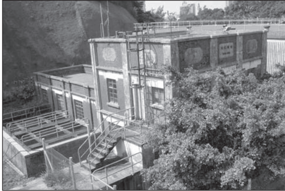
Figure 9. Elliot Treatment Works
