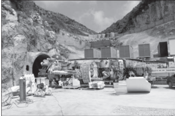
Figure 1. TBM assembly for launch
