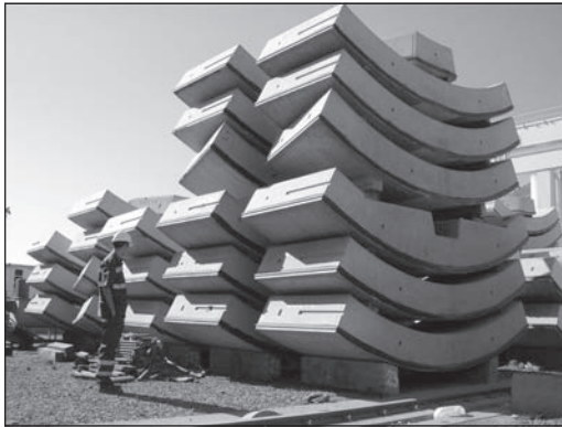
Figure 15. Pajares precast segments (500/ 600 mm thicknesses)
