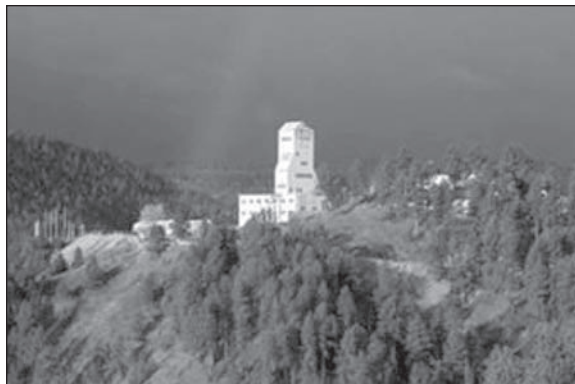
Figure 1. Homestake Shaft Head House
