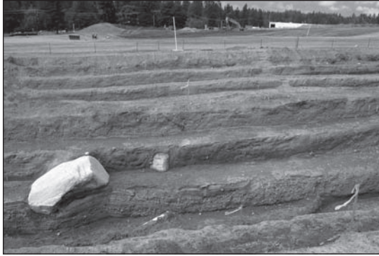
Figure 2. Glacial deposits exhibited in a trench excavated for seismic investigation of the treatment plant site
