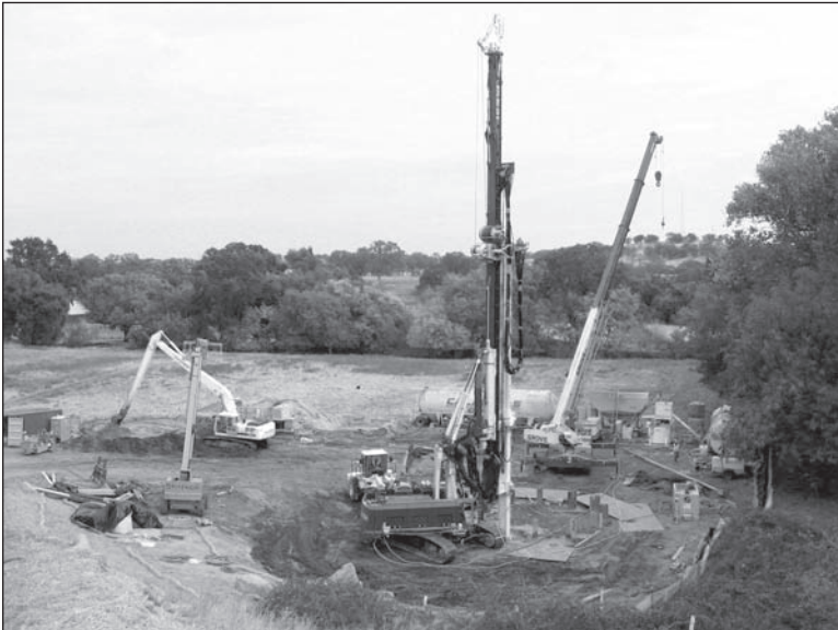
Figure 9. The north shaft site
