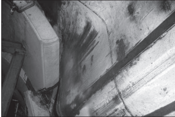
Figure 3. Tail TBM shield damaged and bent
