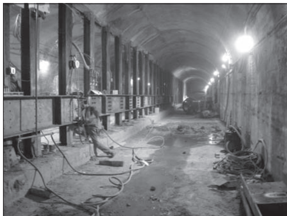
Figure 10. Installation of underpinning steel on existing center columns
