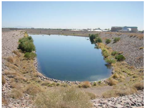
Fig. 4.4 Recharge basin located near a river channel that has high soil permeabilities. A wastewater treatment plant is located in the background, and treated wastewater flows into this recharge basin to supplement regional groundwater supplies
