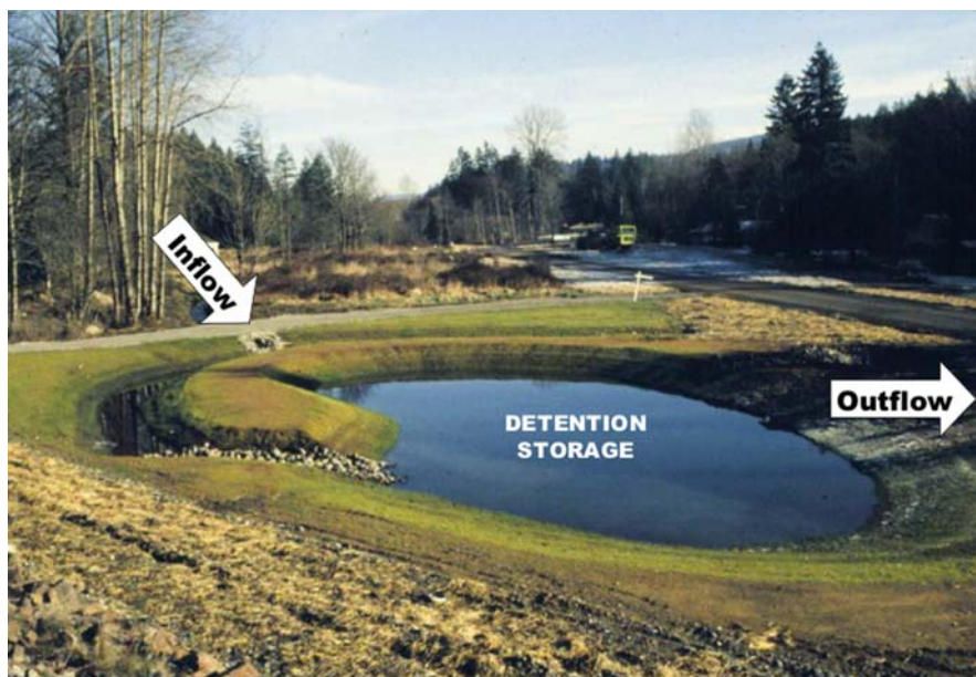
Fig. 6.6a A detention pond, designed to capture and temporarily store runoff from the adjacent residential development before releasing the water to the downstream channel (King County, Washington)
