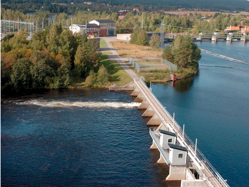
Fig. 1.3 The Dönje Hydropower plant. Source Unknown
