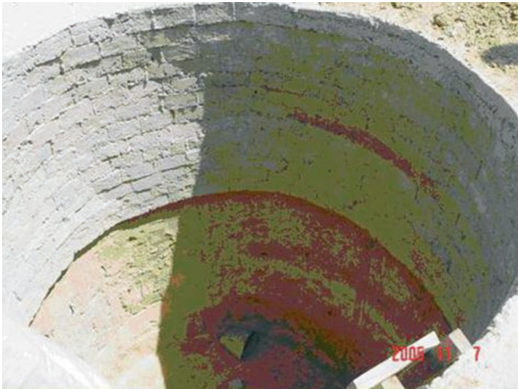
Fig. 4.9 Excavation and casting of concrete wall of water in unstable subsoil
