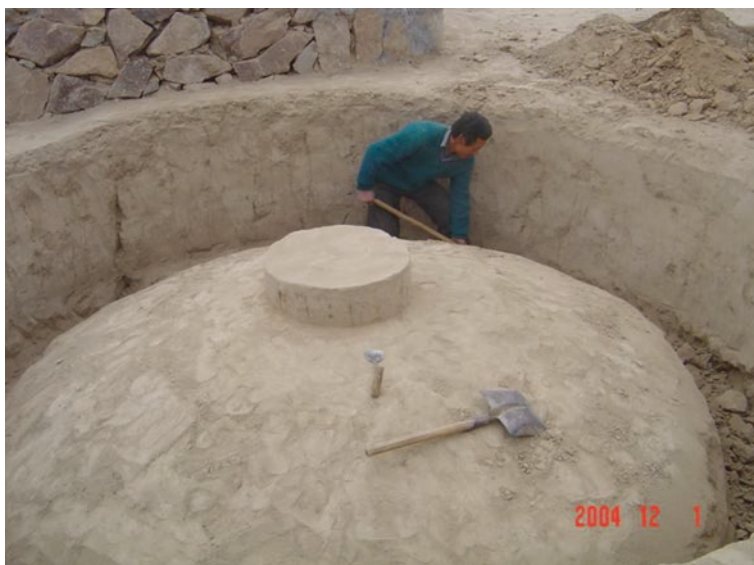
Fig. 4.5 Earth mold for casting concrete dome of water cellar
