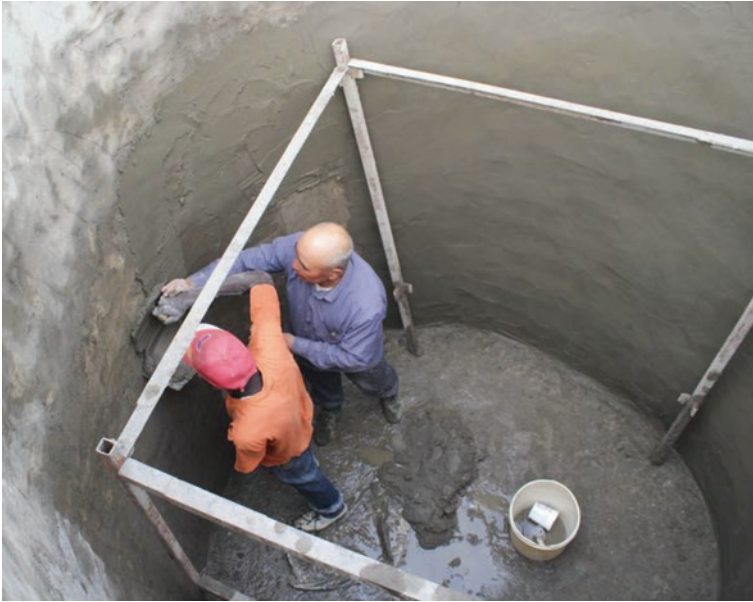
Fig. 4.8 Plastering the wall of the cellar with cement mortar
