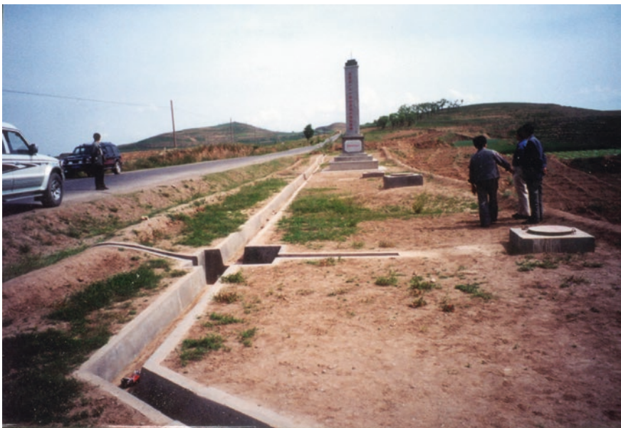
Fig. 3.7 Highway catchment for collecting rainwater for irrigation
