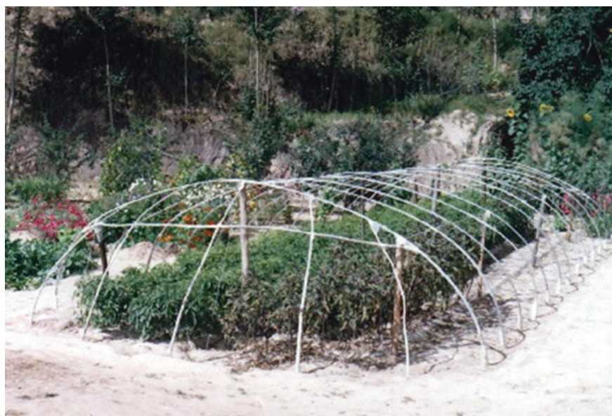
Fig. 1.5 RWH irrigation greenhouse built in 1991 in Beishan, Yuzhong County
