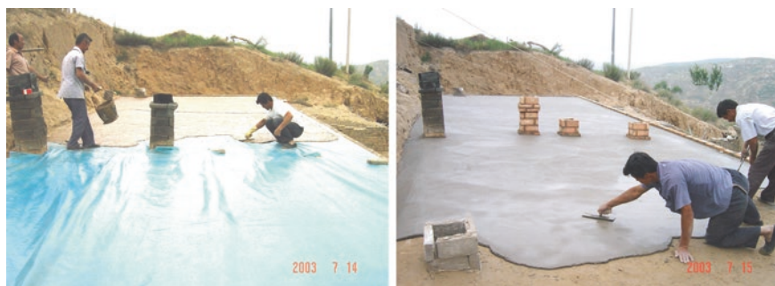
Fig. 3.6 A new type of roof structure for rainwater catchment Courtesy of M. Cheng of Inner Mongolia Research Institute for Water Resources
