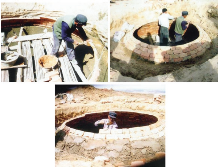
Fig. 4.6 Cost effective way for construction of brick dome of a water cellar. Source Zhu et al. (2012)
