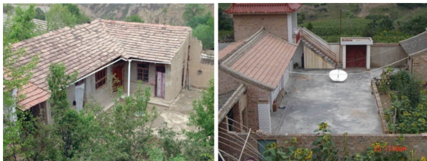
Fig. 3.5 Two kinds of collecting domestic water to the storage tank: with gutter and downpipe ( left ); without gutter and downpipe ( right )
