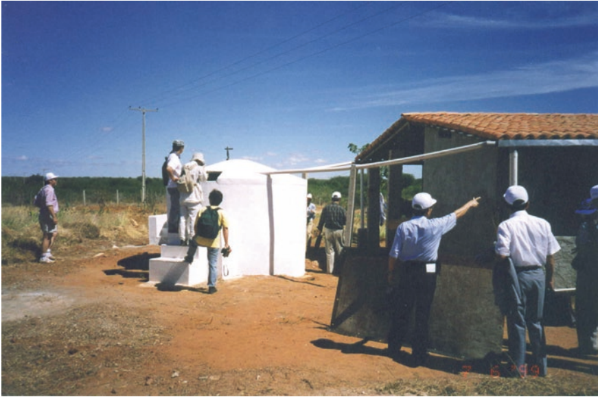
Fig. 7.1 A typical 16 m 3 Ferrocement Rainwater tank collecting runoff from a clay tile roof in Pernambuco State, Brazil (Photo: Courtesy Andrew Lo 1999)
