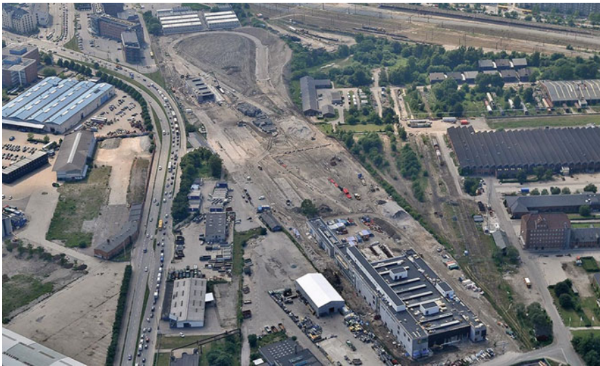
Fig. 3 Control and maintenance center site
