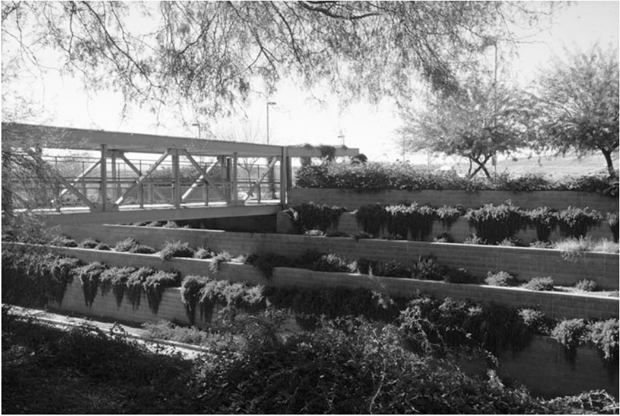
Fig. 9.15 27th Avenue Solid Waste Management Facility, Phoenix, design by Michael Singer and Linnea Glatt (Photograph by Frederick Steiner)
