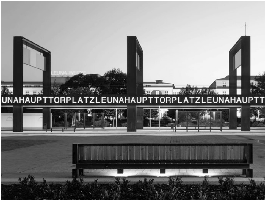
Fig. 10.4 Tramway stop by night detail
