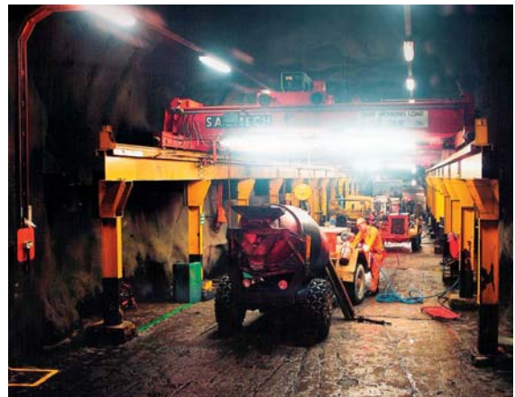
Fig. 335 Massive machinery is required to extract and transport of ore and overburden
