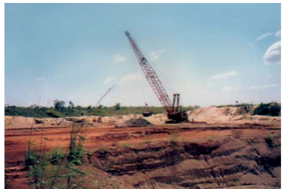
Fig. 159 Drag-line set-up of diamond bearing gravels in Banankaro in the Kerouane region
