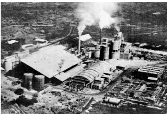
Fig. 301 The oldest cement factory in Africa at Bargny near Dakar, where Cretaceous limestone is quarried (1964)
