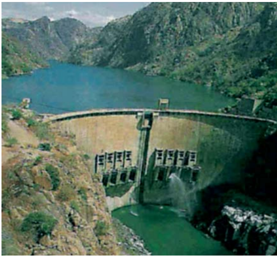
Fig. 253 The wall of the Cahora Bassa dam in central Mozambique.
