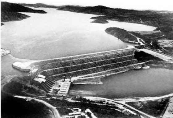
Fig. 151 The 113 m high rock-fill dam at Akosombo in the Volta Gorge of southern Ghana, holding back an artificial lake of 8482 km 2 (1964)
