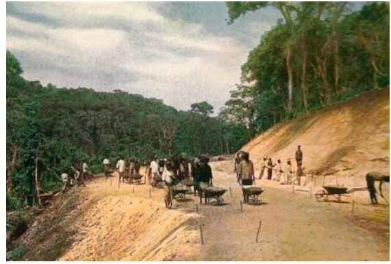
Fig. 376 Road construction work in southern Togo during German colonial times (about 1912)
