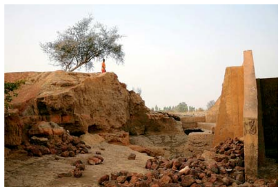
Fig. 47 Heavy rains and flooding in southern Burkina Faso caused this local dam to break-off
