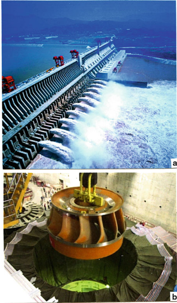
Fig. 13 Three Gorges Dam Project, Yangtze River, China (a) (Photo courtesy of nopic.com). (b) shows a 425 t Francis turbine runner being inserted into the turbine housing (Courtesy of Alstom Turbine Technology Center, France; the manufacturer)
