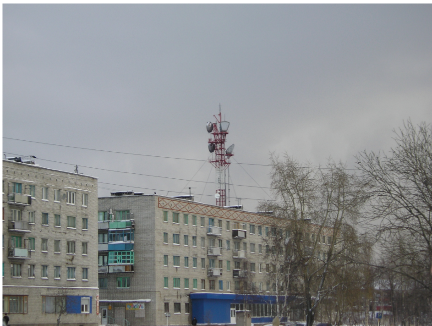
Figure 9 The Radio mast in the outskirts of the town Belomorsk where one of the CR-II seismic stations was installed. Due to the noise produced by the mast related activity and the proximity of the town infrastructure the operation of this station was a scientific failure
