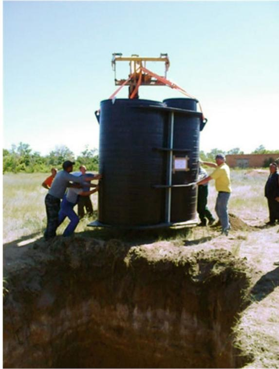
lysimeters is not affected before it reaches the filter layer. The composition of the filter layer was chosen to allow free drainage of seepage water. The vessels were transported to Poluyamki and positioned in the lysimeter station on load cells using a three-legged steel frame.
