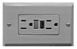
**FIGURE 18.5:** GFCI safety outlet found in one author's kitchen. The black is the TEST button; when pushed, it shuts off power if the device is working properly. The red is the RESET button; when pushed it returns the outlet to normal functioning after a test or if the GFCI has tripped the circuit. The smaller slot plug represents the hot side of the circuit; the larger slot, the neutral side. The circular hole connects the ground prong to the grounded circuit.
