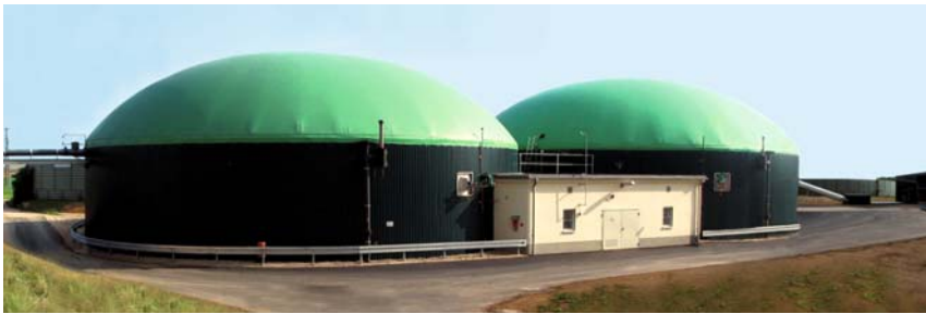
Figure 11.3 Biogas reactor with plastic cover for gas storage (Markert, 2008)
