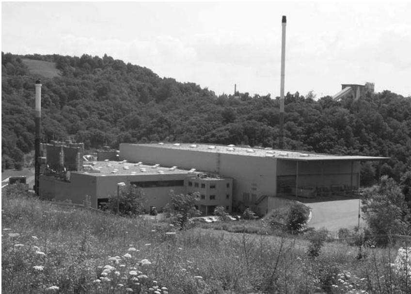
Figure 12.7 Total view of an industrial scale MBP facility in Germany
