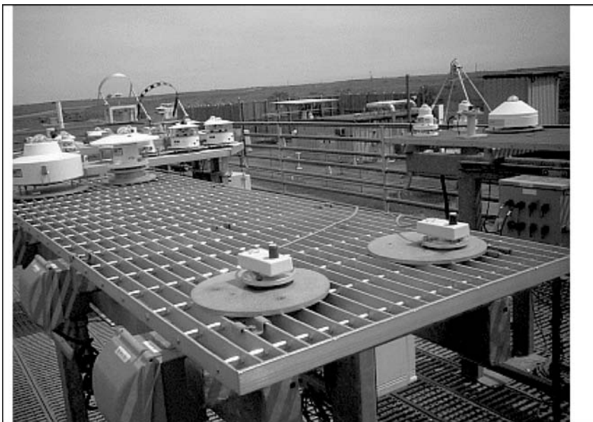
Figure 4.10. PDB-C139 SIPs being calibrated at NREL.
