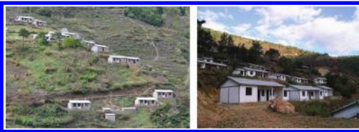
Figure 6. Concrete box houses.
