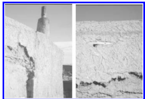
Figure 6. Exterior wall and roof of typical alkaline soil dwelling.
