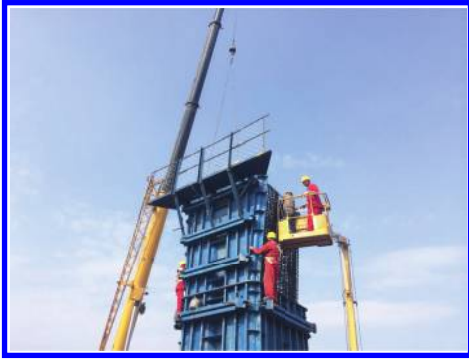
Figure 5. Installation of pier column formwork.
