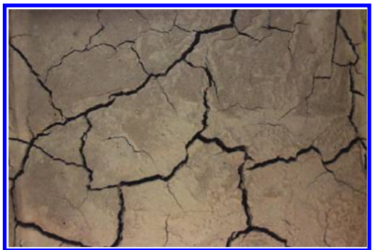
Figure 7. Original fracture of expansive soil.
