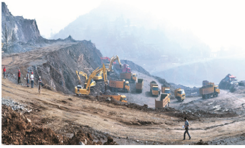
Figure 1. Bench blasting in Hongshuitai.
