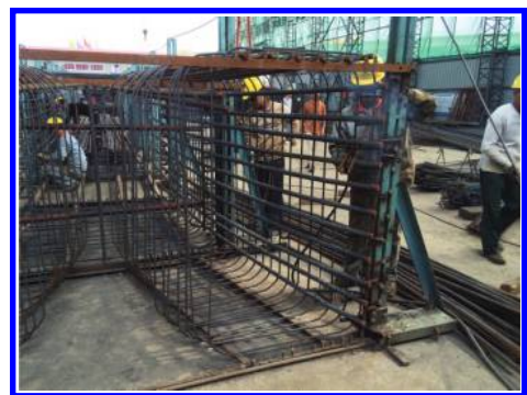
Figure 1. Processing of reinforcing cage.
