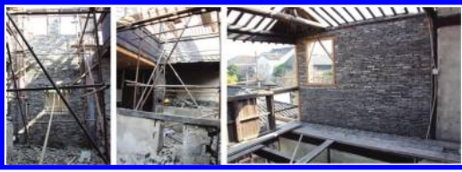
Figure 6. The transformation of traditional residence completely dismantled the internal structure.
