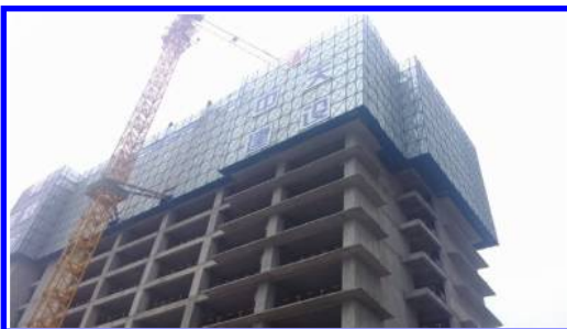
Figure 1. The adhesive integral-lift scaffold during the structure construction.
