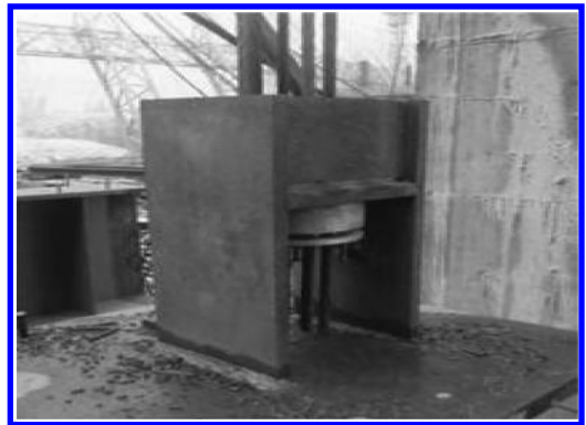
Figure 3. The spreaders arranged on the top chord.
