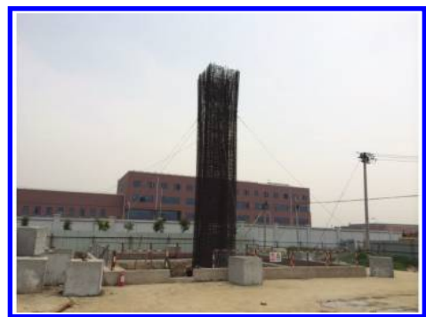
Figure 4. Fixed mooring rope and ground anchor.
