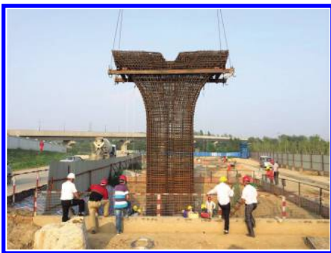
Figure 3. Lifting of reinforcing cage.
