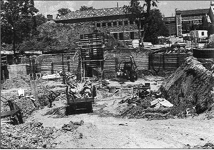
Figure 7-27. Foundation Work at Site 2
