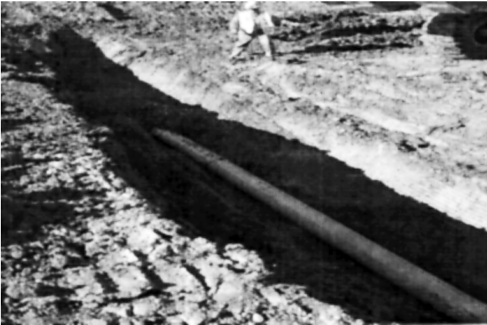
Figure 7-45. Backfilling around Pipe in Trench
