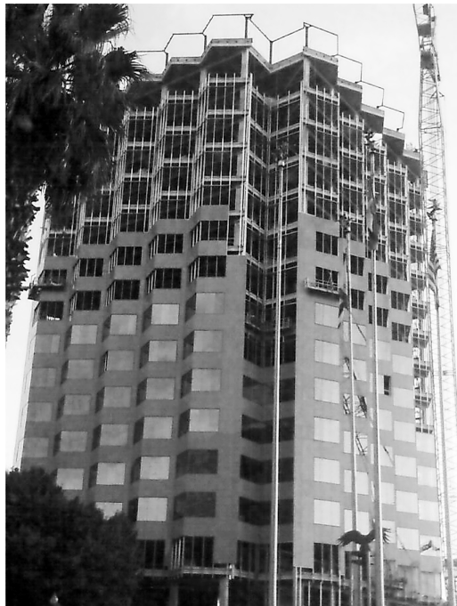
Figure A-3. Curtain-Wall System in Midcompletion
