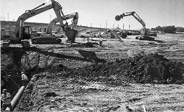
Figure 7-44. Worker Connecting Pipe while in Trench
