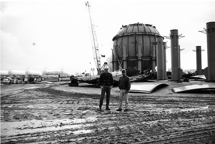
Figure 4-3. Tank Construction Project with Management Personnel Wearing Hard Hats
