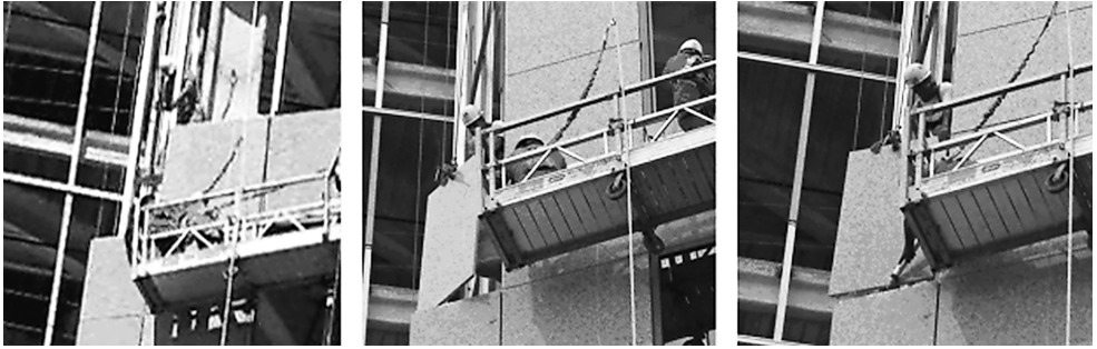
Figure A-34. Worker 3 Reaching Over Edge of Platform to Perform Work
