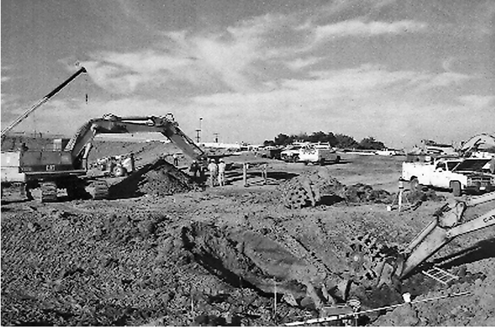
Figure 7-41. Excavating Trench for Pipe Installation
