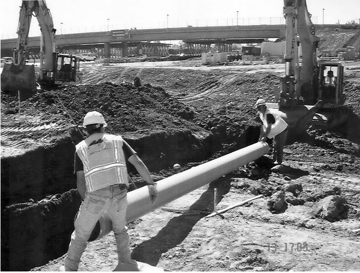
Figure 7-42. Installing Pipe in Trench
