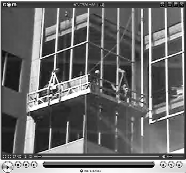
Figure A-16. Installation of Stone Panel Type 1
