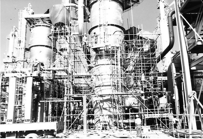
Figure 4-1. Construction of Liquefied Natural Gas Plant in Bontang, Indonesia
