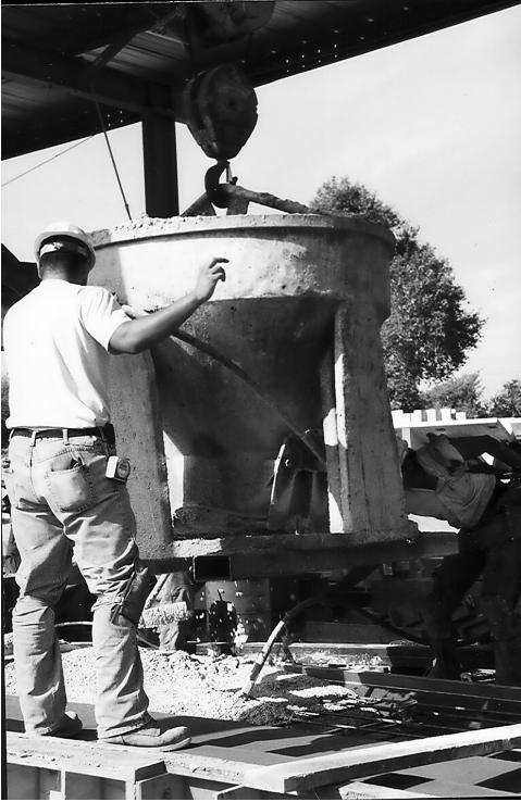
Figure 4-2. Concrete Placement with Worker Wearing Steel-Toed Boots
