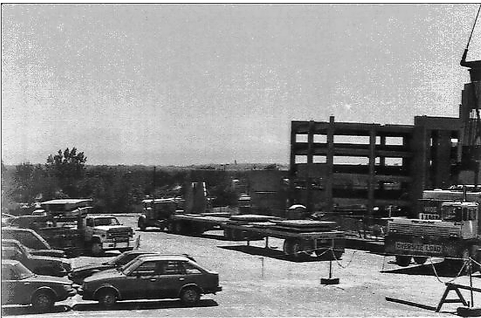
Figure 7-22. Limited Parking Area for Trucks Unloading Precast Members
