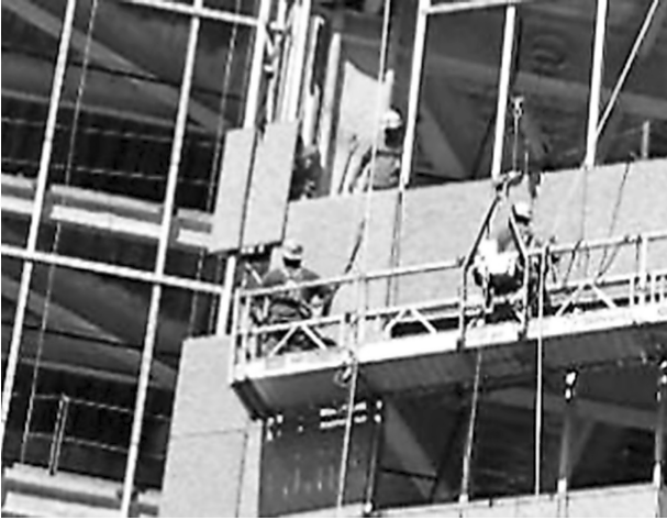
Figure A-33. Worker 3 Idle
