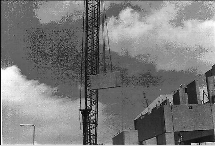
Figure 7-23. Lifting Precast Concrete Member by Crane
