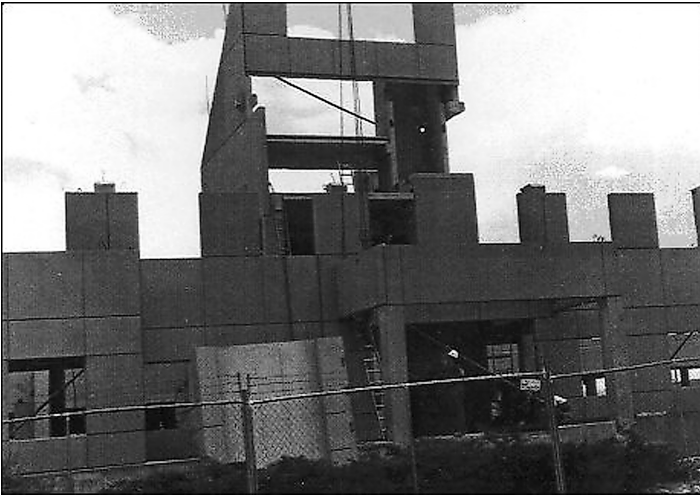
Figure 7-24. Fixing Precast Concrete Member
