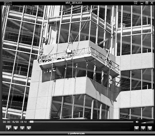
Figure A-17. Installation of Stone Panel Type 6
