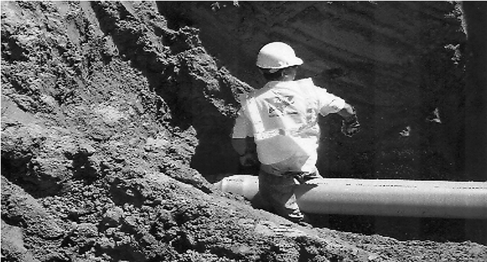
Figure 7-43. Pipe Installed in Trench
