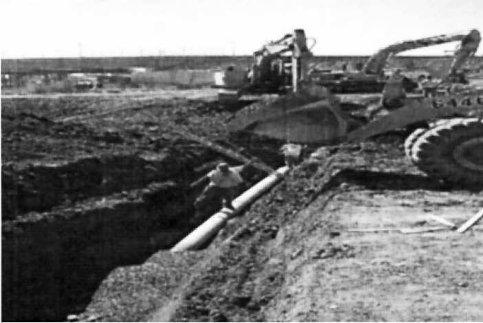
Figure 7-46. Backfilling over Pipe in Trench
