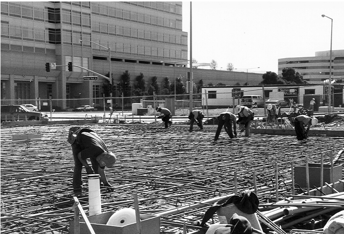
Figure 4-6. Intricate Rebar-Tying Operation for Concrete Slab
