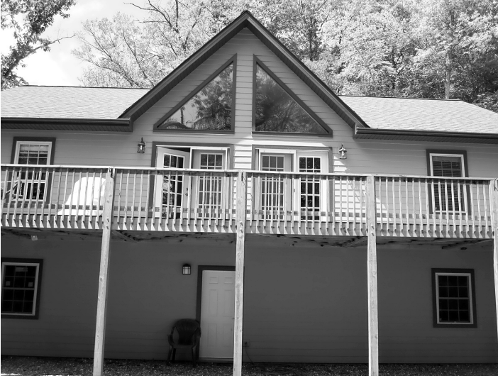
Figure 13-3. Home with Hardie Board Siding
