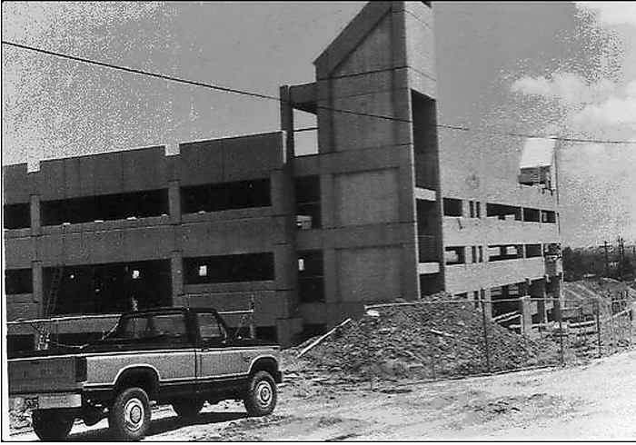
Figure 7-19. Site 1 Car Parking Structure
