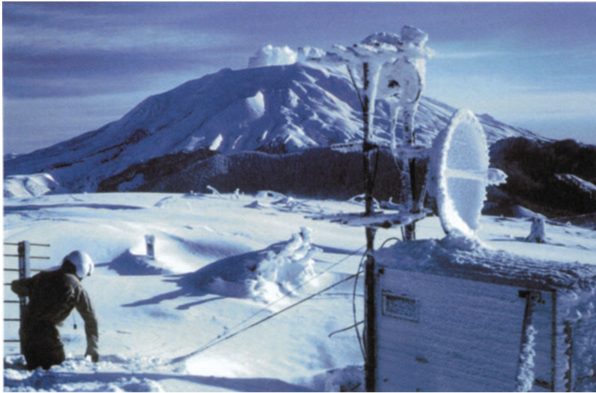
Figure 2.7. Flat Top radio repeater station near Mount St. Helens in January 1982. Harsh winter conditions can hamper volcano-monitoring efforts, but such difficulties can be overcome through experience, ingenuity, good planning, and hard work. USGS photograph by Daniel Dzurisin.
