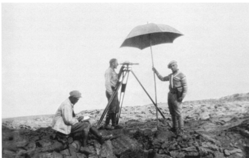
Figure 1.21. (top) US C&GS leveling crew beginning a spur line into Moku'āweoweo Crater near the summit of Mauna Loa Volcano, Hawai'i, in 1927. (bottom) The last set-up on the summit of Mauna Loa (elevation 4,169.7 m). The survey began two months earlier at a tide gauge in Hilo. Skip Theberge, NOAA Central Library, Silver Spring, Maryland kindly provided these images from Historic C&GS Catalog of Images, C&GS Season's Report Simmons 1927.
