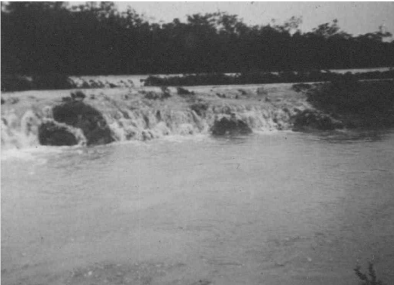
FIG. 5.25. High seas spilling over the sea wall at Tabucola on the northern coast of Vanua Levu island in Fiji, pushed up by storm surge associated with Tropical Cyclone Gavin on the afternoon of 7 March 1997. Photo courtesy of the Land and Water Management Division, Fiji Ministry of Agriculture.
