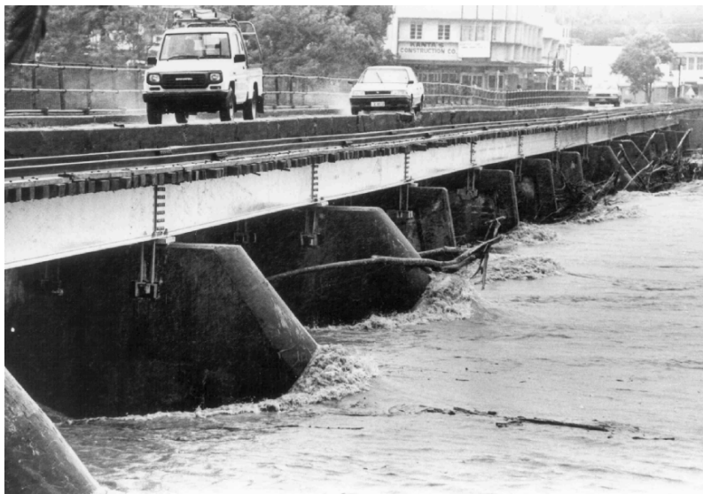
FIG. 9.4. View of the old main bridge over the Sigatoka River at Sigatoka town, southwest Viti Levu island in Fiji, during the flood produced by Tropical Cyclone Kina in December 1992. The water level is 10 m or more below the bridge at normal flow. Courtesy of the Fiji Times.
