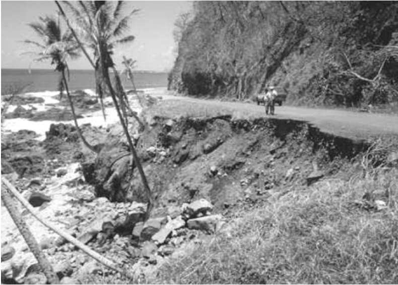
FIG. 7.7. Coastal erosion east of Apia on Upolu island in Samoa, caused by storm waves accompanying Tropical Cyclone Ofa in February 1990. Source: Rearic (1990).
