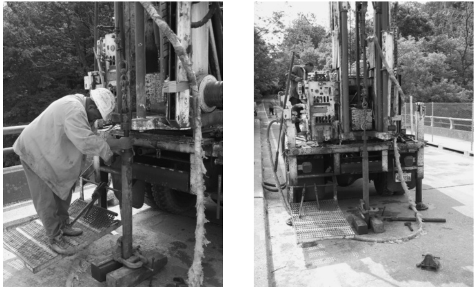
Figure 17.7 Drilling rod with split-spoon sampler lowered to the bottom of the borehole (Courtesy of Braja M. Das, Henderson, Nevada)
