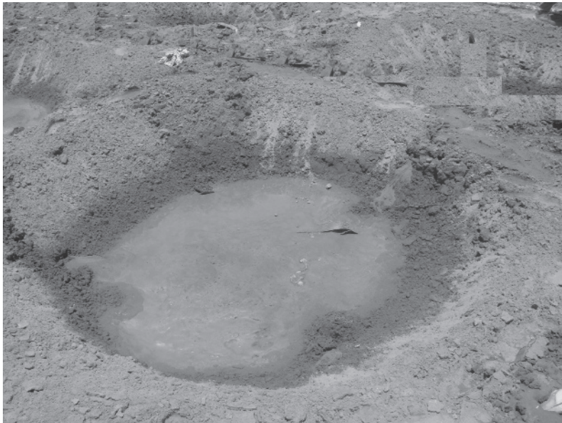
Figure 6.37 (a) Dynamic compaction in progress; (b) a site after completion of dynamic compaction (Courtesy of Khaled Sobhan, Florida Atlantic University, Boca Raton, Florida.)
