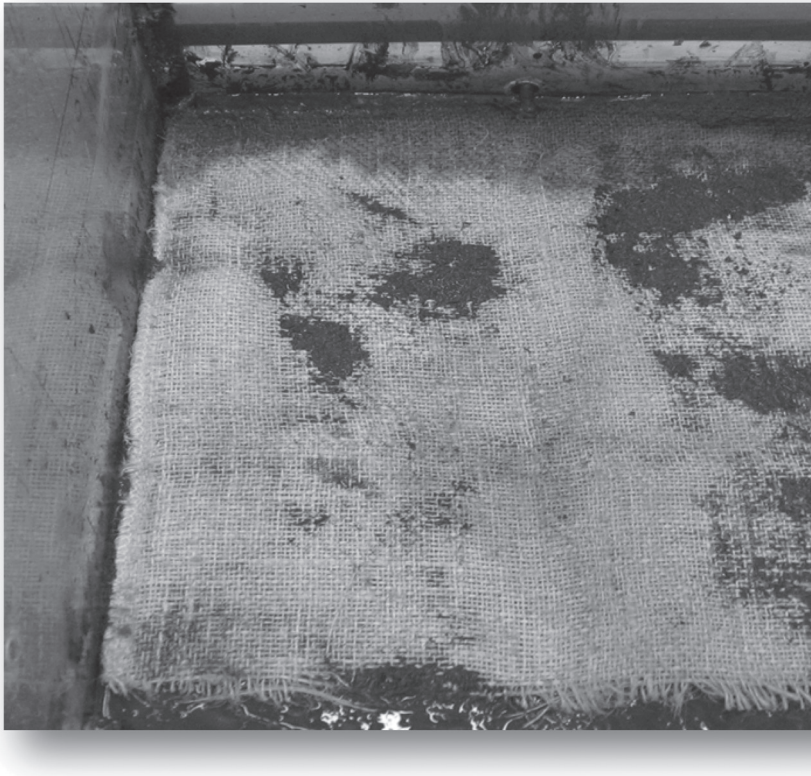
Figure 9.4 Layout of sisal geotextile over soft soil (before erection of embankment)
