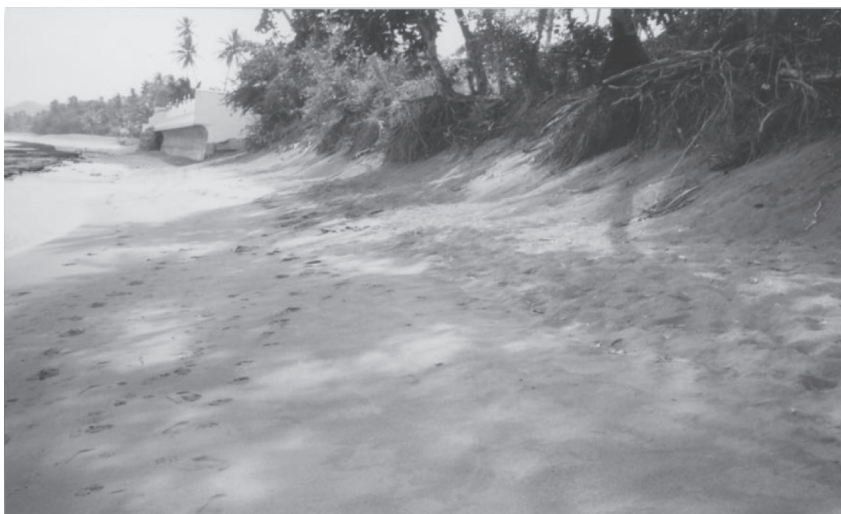
Figure 3.1 Extensive beach erosion in Tobago, Caribbean Islands
