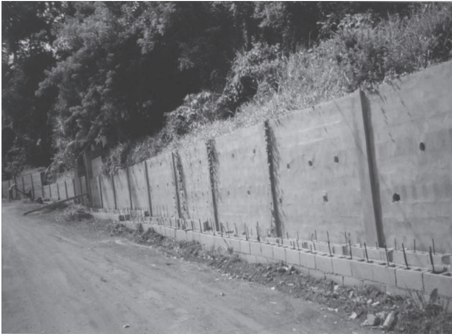
Figure 3.2 Using retaining wall to minimise soil erosion at Plymouth, Tobago
