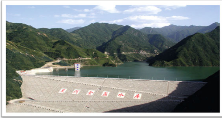
Fig. 1 Jinpen Reservoir in Shaanxi Province
