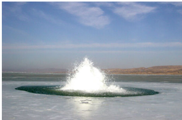
Fig. 3 The water-lifting aerator in operation
