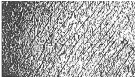
Figure 7.27: Crack pattern after 22,000 thermal shock cycles.
