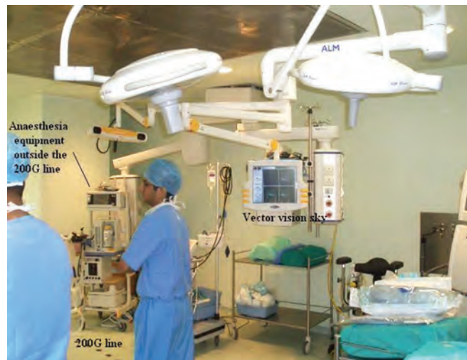
Fig. 17: Arrangement of equipment in the Brain suite
