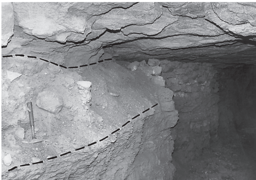
Fig. 5.25. Wadi Khalid, mine 42. This Early Bronze Age mine has been cut by a modern prospection tunnel of the Natural Resource Authority. It is difficult to localize the original mine as it has been almost systematically backfilled. The original height of the now backfilled mining chamber can be recognized with the help of the scale. The bottom and roof of the mine are marked by the hatched line . The lateral extension of the pit, constructed as a room and pillar mine, is roughly 30 × 50 m
