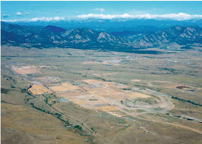
Fig. 10 Aerial photo of the remediated Rocky Flats site, October 2005
