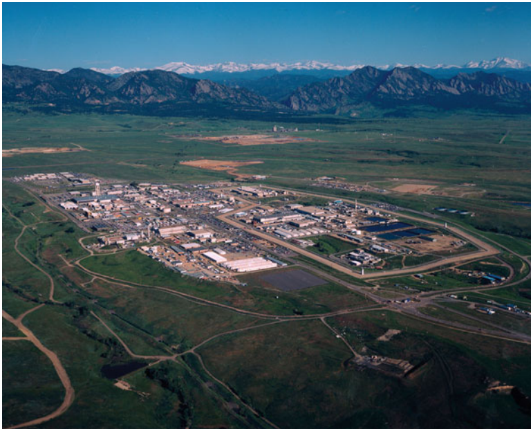
Fig. 1 A 1995 aerial photograph of the RFETS showing the industrial area
