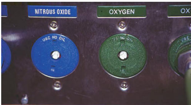
Fig. 6.9 Ohmeda “quick connect” gas outlets. These are gas specific within each manufacturer but not between manufacturers
