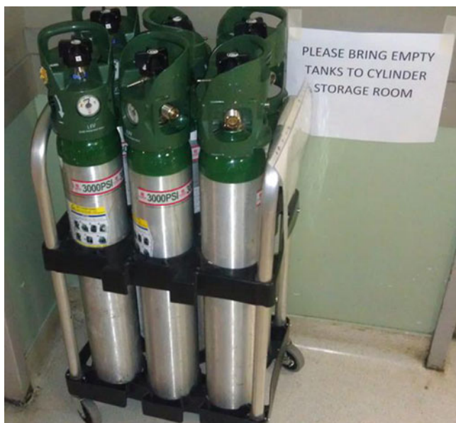
Fig. 6.6 Storage rack of full oxygen tanks. Empty tanks are stored elsewhere to avoid confusion
