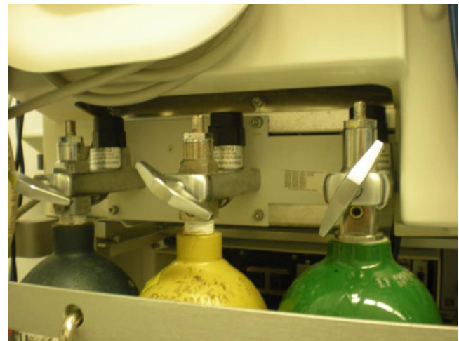
Fig. 6.3 Oxygen (green) and air (yellow) E cylinders in respective hanger yokes in rear of workstation
