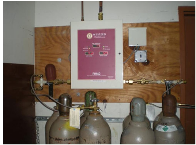
Fig. 6.2 Cylinder manifold arrangement for pipeline supply
