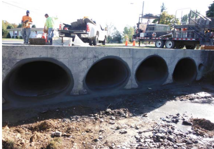
Figure 4: Four large parallel culverts
