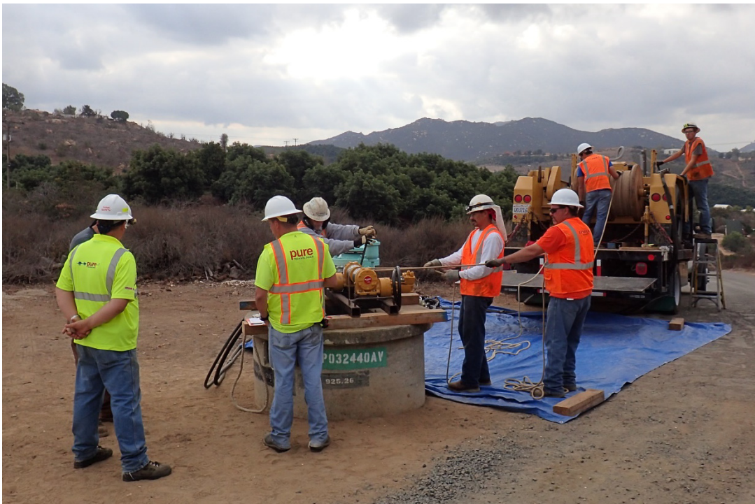
Figure 3. Winching of MFL tool
