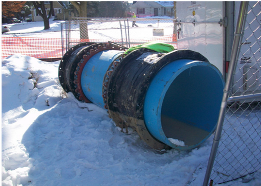
36" PVC pipe, used to combine sections of lined pipe.
