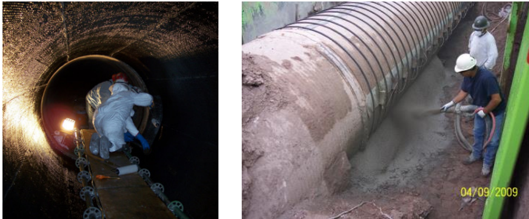
Figure 5. Typical internal CFRP and external post-tensioning repairs.
