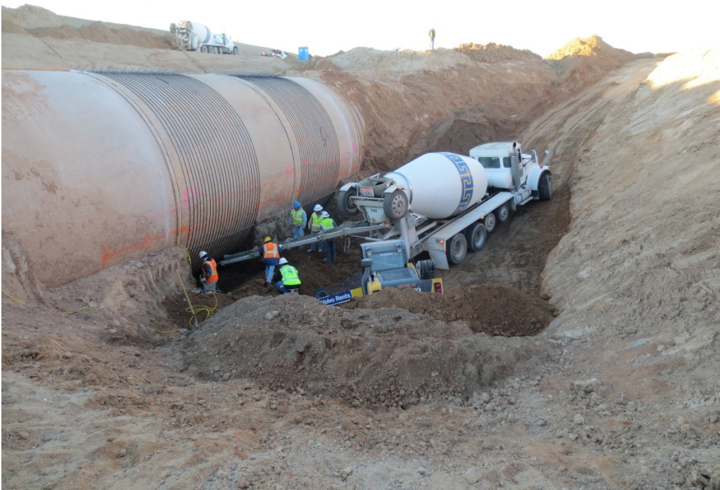
Figure 4 - Placing CLSM Beneath Pipe
