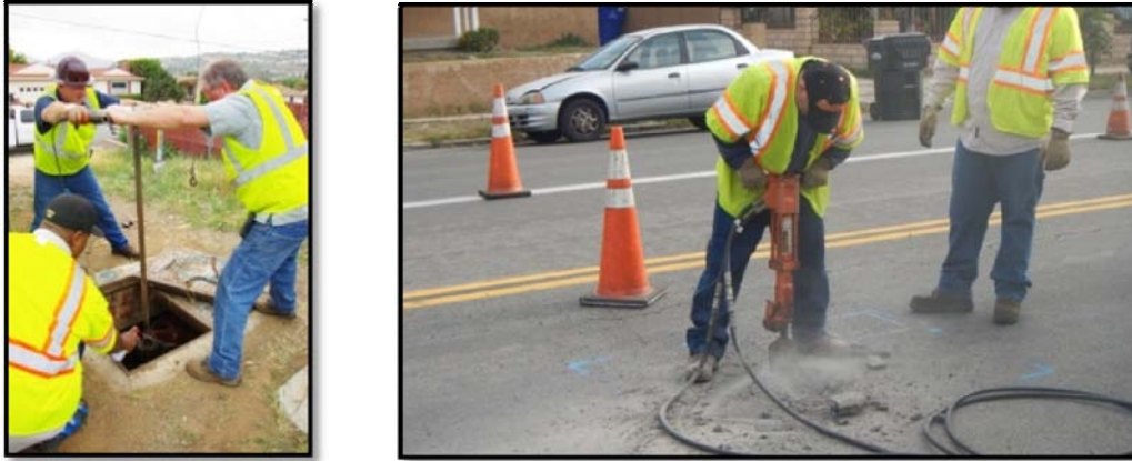
Figure 14. Left: Exercising an in-line valve with the help of City crews. Right: Uncovering a paved-over-in-line valve.
