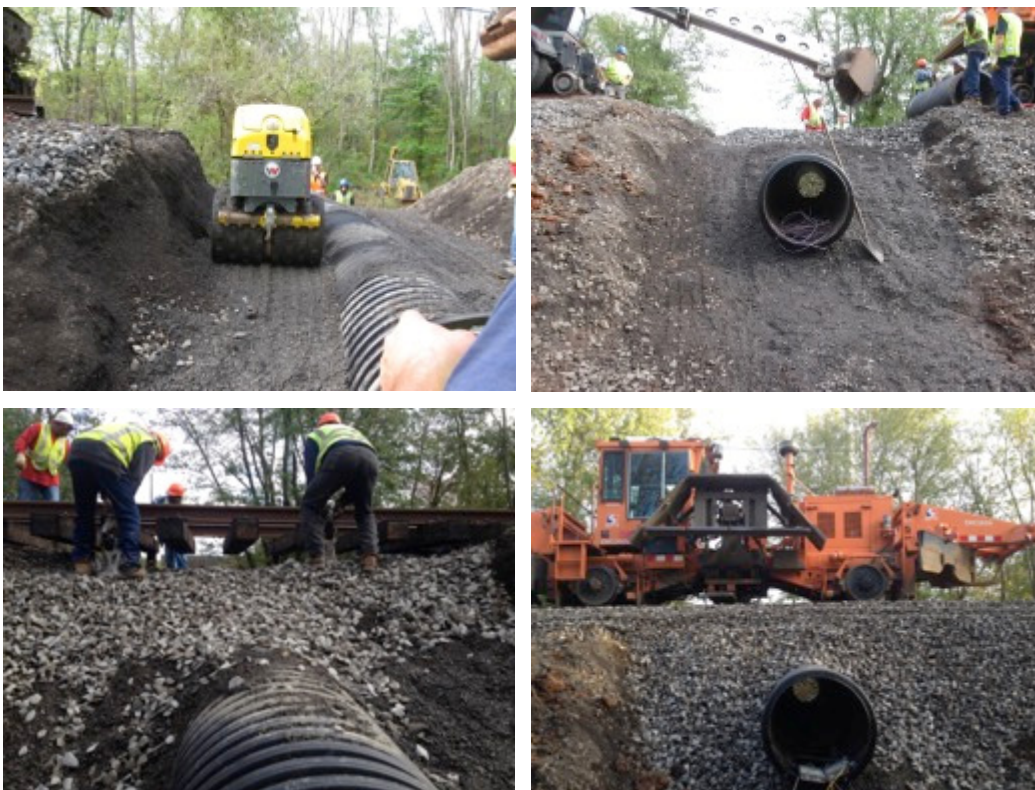
Figure 5: Installation of pipe and railroad track
