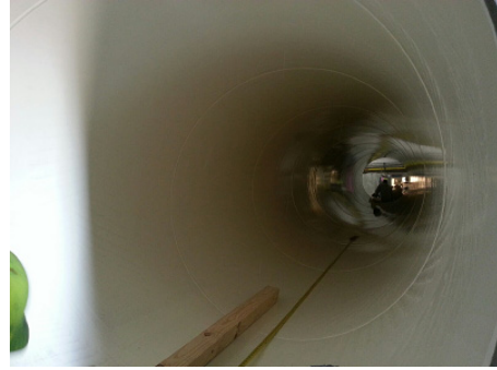
Figure 6: The location of the inside stull is determined
