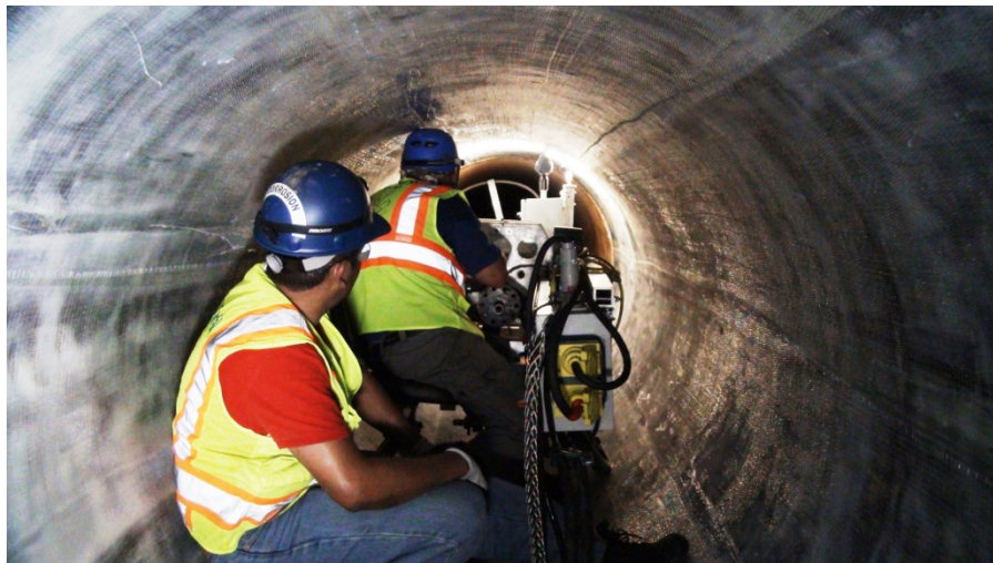
Figure 6 – Hybrid FRP System – Steel reinforcement installation
