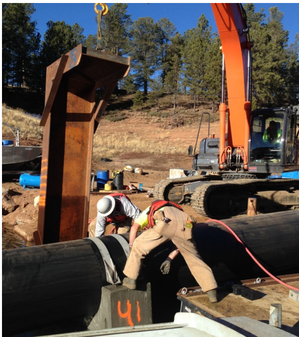
Figure 7 - Ballast block installation.
