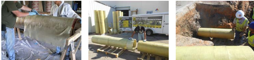
Figure 1. Honeycomb-FRP pipe being made on a mandrel for repair of culvert.
