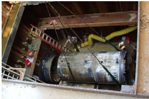
Figure 4. MTBM Received at Shaft 5
