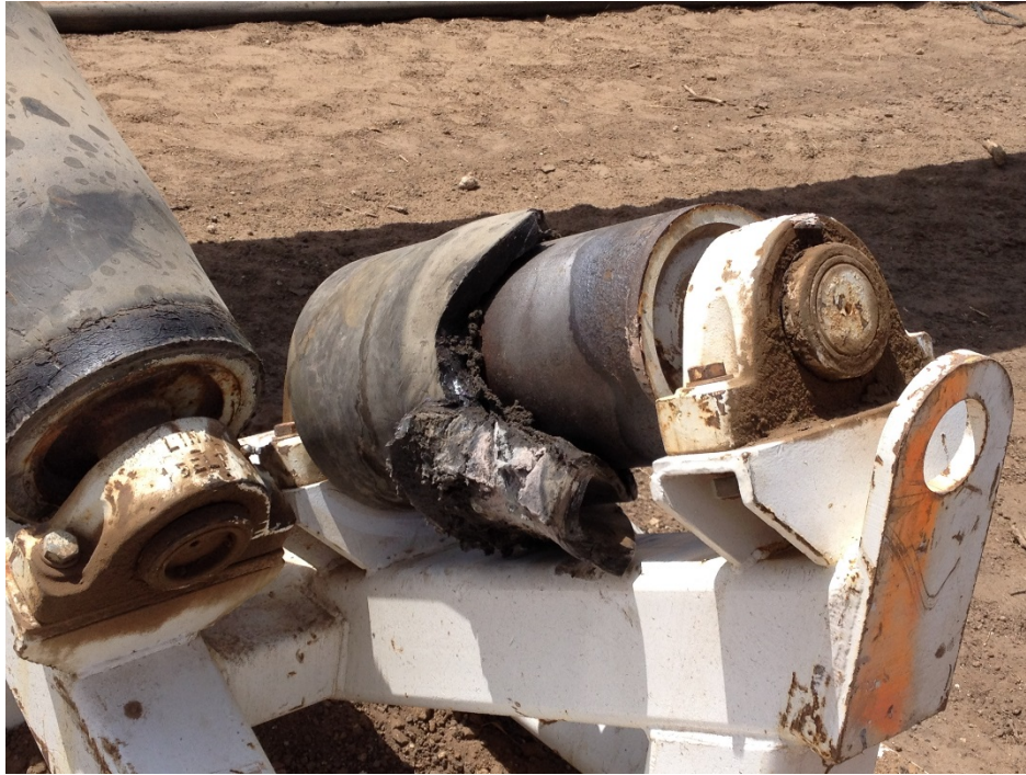
Figure 6: Broken Roller Support
