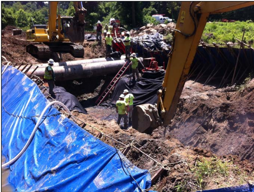
Figure 6: Open cut river crossing using PortaDam and flume bypass
