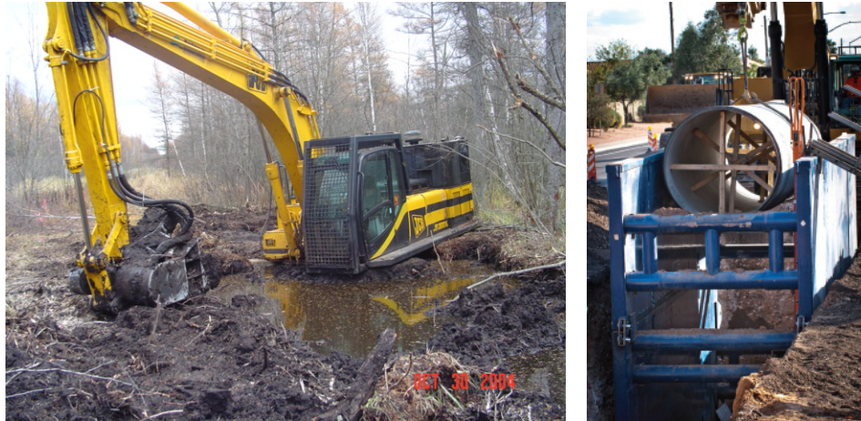
Figure 16 – High Water Table and Trench Box
