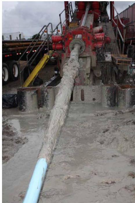
Figure 4. Completed 4-inch FPVCP conduit installation by HDD.
