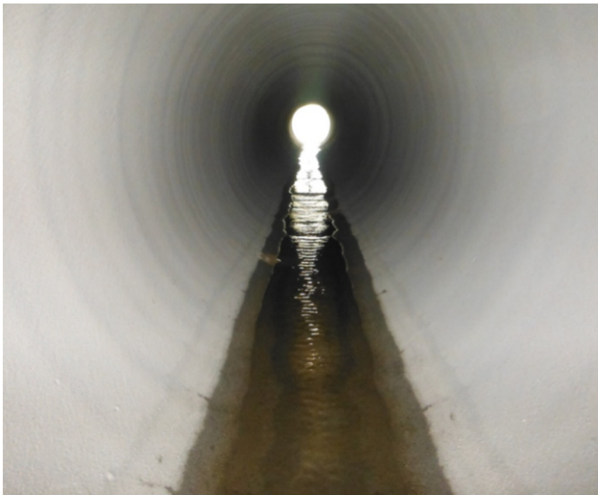
Figure 14. After CCCP rehabilitation.
