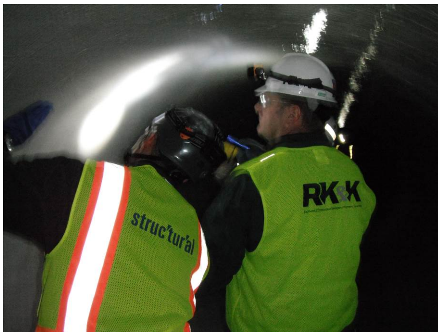
Figure 4. Inspection of top coat
