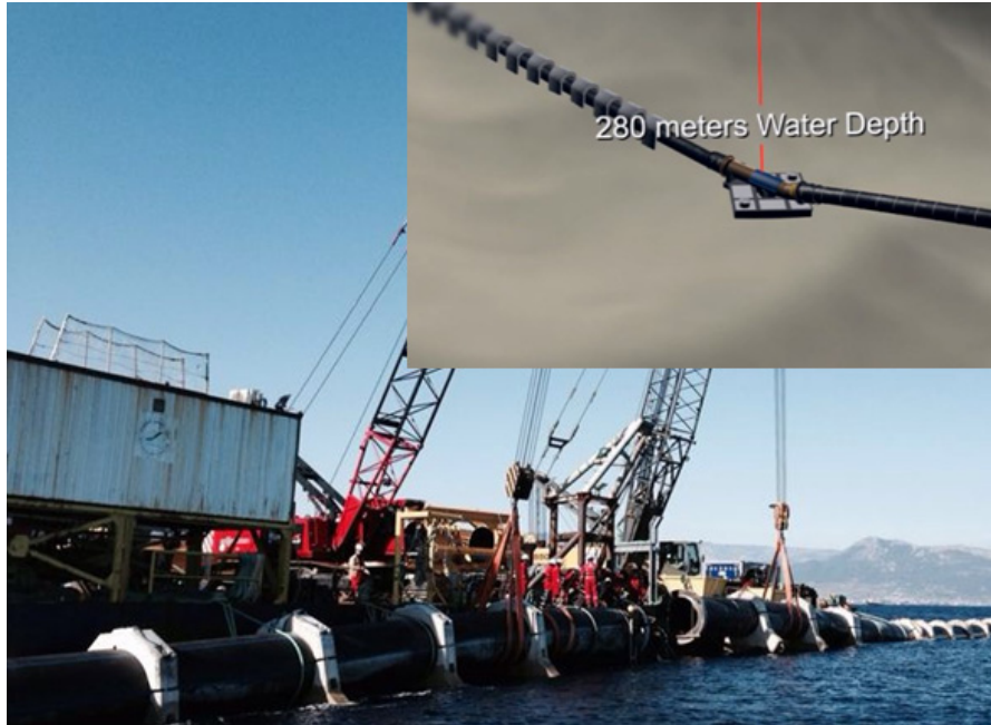
Figure 6: PE 100 Pipe with Concrete Blocks
