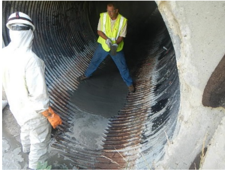
Figure 4. CMP invert repair.
