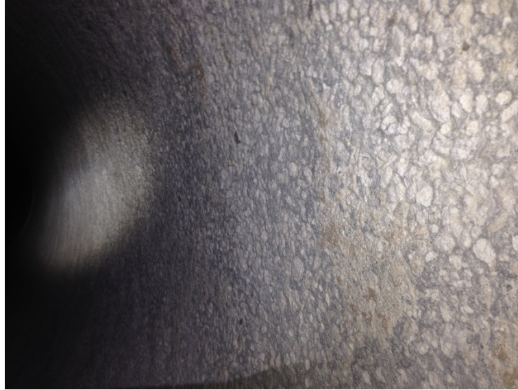
Figure 5 – Prepared concrete substrate – MDWASD 54-inch PCCP
