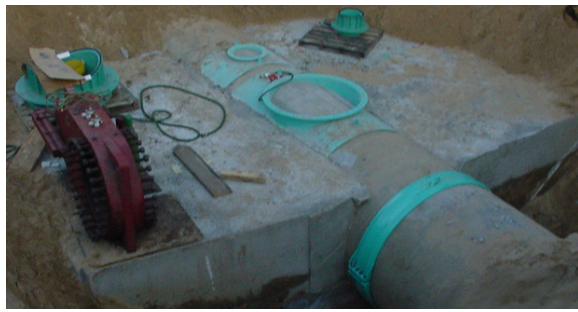
Figure 17 Tapping fittings and thrust block
