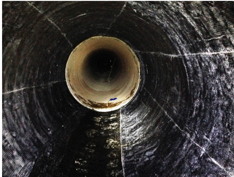
Figure 2 – Typical FRP installation
