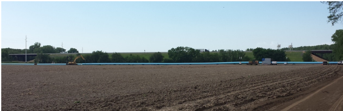
Figure 5 – Kansas River Bore Pipe String
