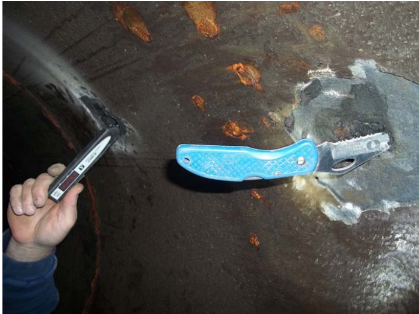
Figure 8. Verification of Remaining Wall Thickness
