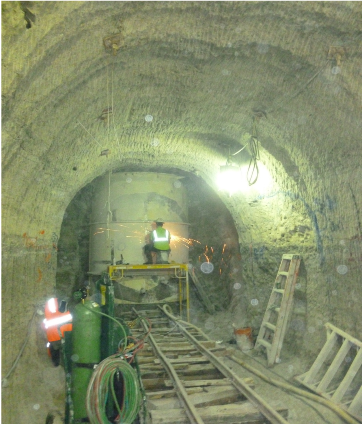
Figure 2. Field Cut-In Outlet Location around Elevation 450 feet.
