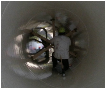
Figure 9: The final leg is placed, supporting the full circumference of the cylinder
