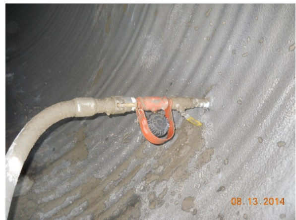
Figure 8. Grout pumping.
