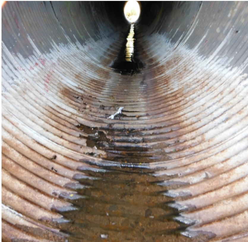
Figure 13. Before CCCP rehabilitation.
