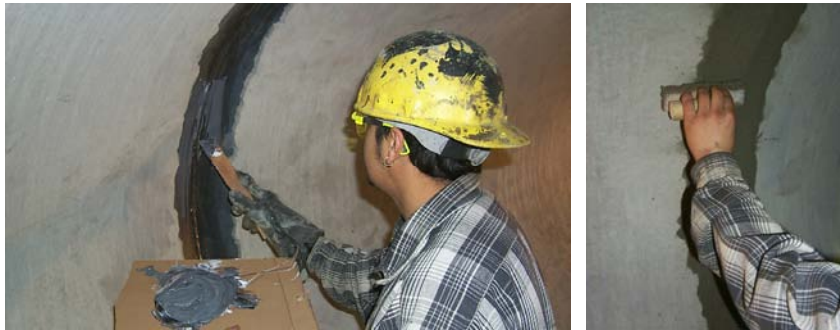
Figure 15 – Interior Joint Grout
