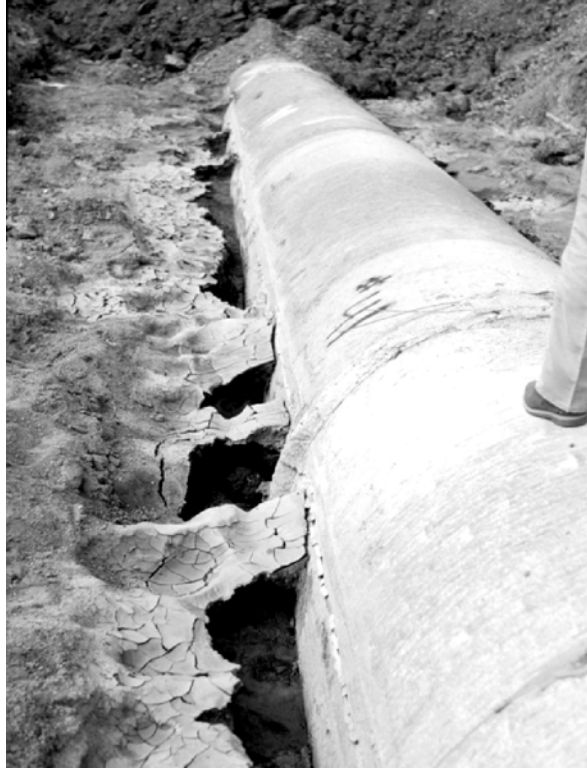
Figure 6 Too Many Fines for Saturation and Vibration
