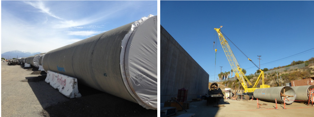
Figure 6a and b Pipe Manufacturers Offsite Storage and Site Storage
