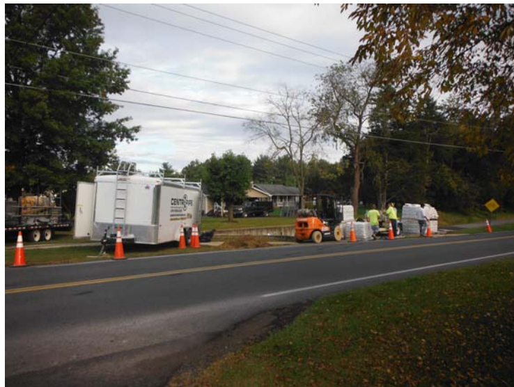
Figure 6: Trenchless repair leaves road open to traffic
