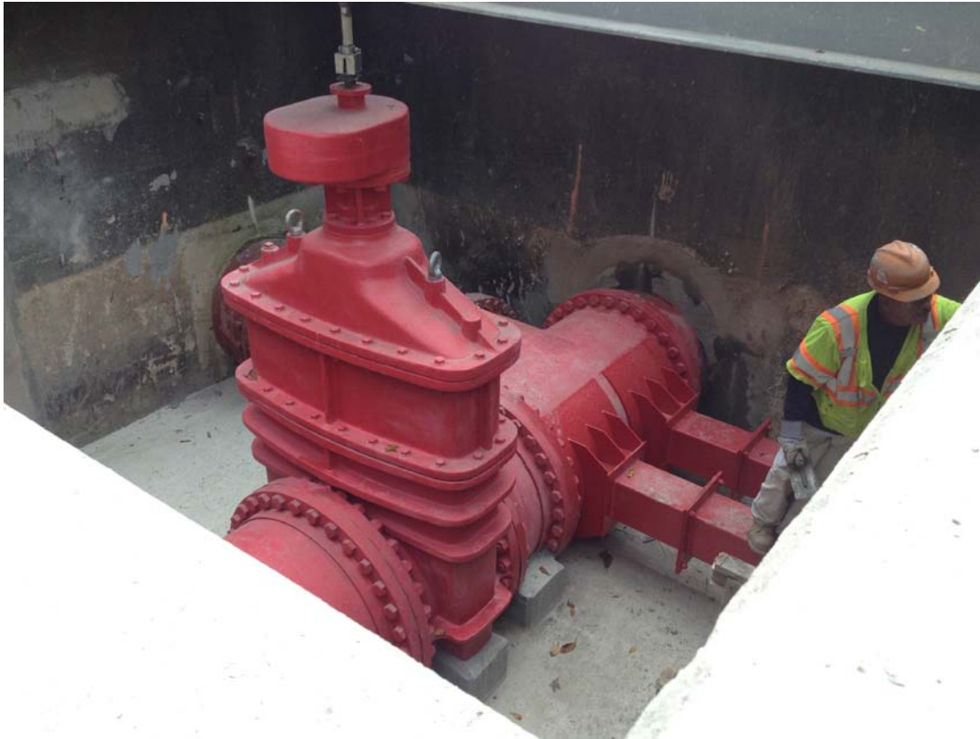
Figure 3. Completed outlet structure with new gate valve and removable thrust blocks
