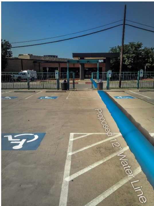
Figure 2 Building along Proposed Alignment
