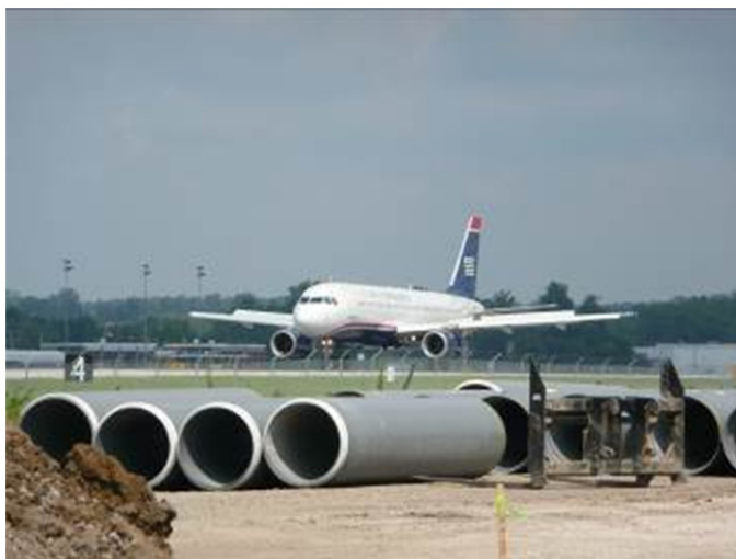
Figure 5. Triple Wall PP Pipe on the Port Columbus International Airport Project
