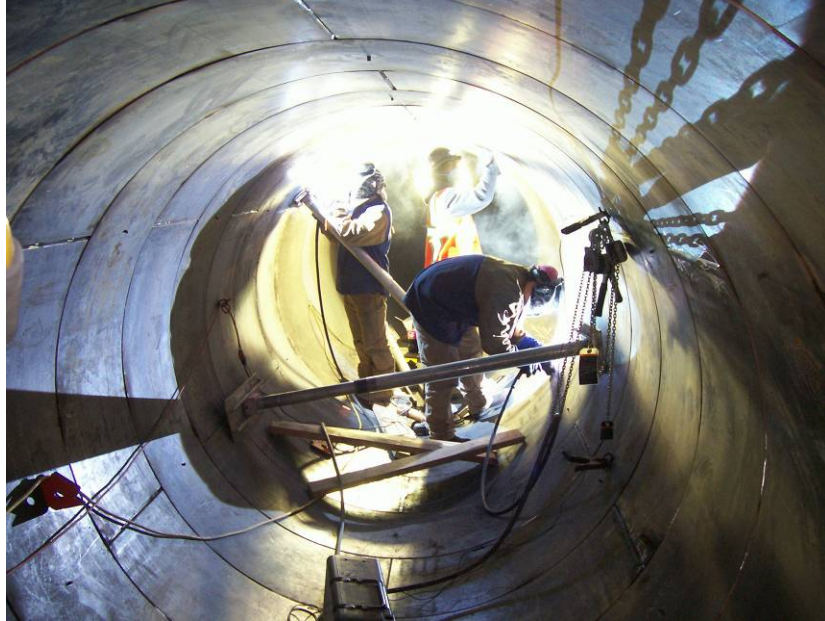
Figure 4: Internal Repair of 78-inch PCCP with Epoxy Coated Steel Lining
