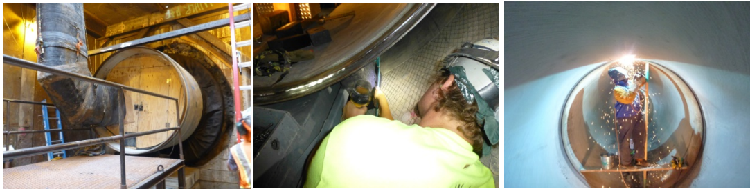
Figure 9a, b and c Pipe Placed Against I-Beam, Blocking and Welding
