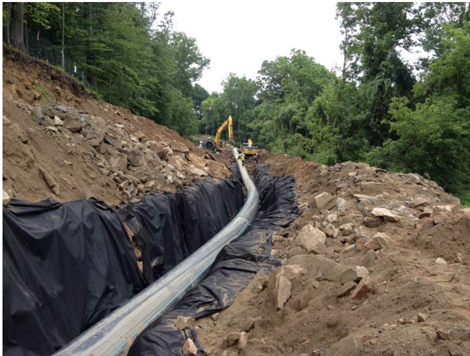
Figure 2: Installation of the winding 30-inch HDPE water main
