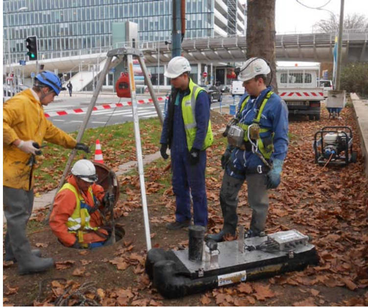
Figure 4. The SewerVUE MPIS and field crew before deployment in Boulogne-Billancourt.
