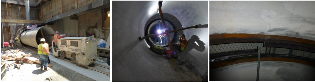
Figure 8a, b and c Pipe Installation and Placement
