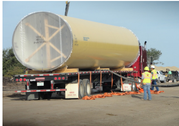
Figure 10: 50-ft Section of Pipe on Truck w/ End Cap
