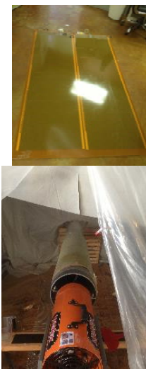
Figure 5. LaminaHeat and propane heater tried in curing the pipe.
