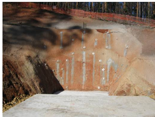
Figure 4. (above) Retrieval portal site and the temporary support
