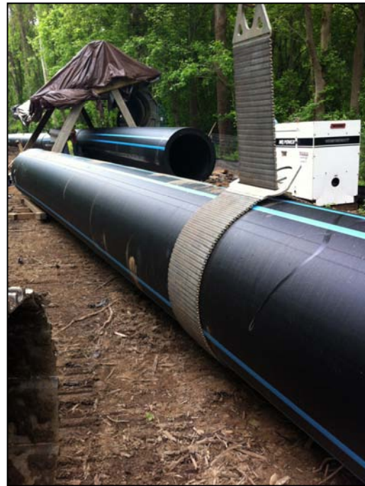
Figure 5: Steel Strap used for lifting the pipe
