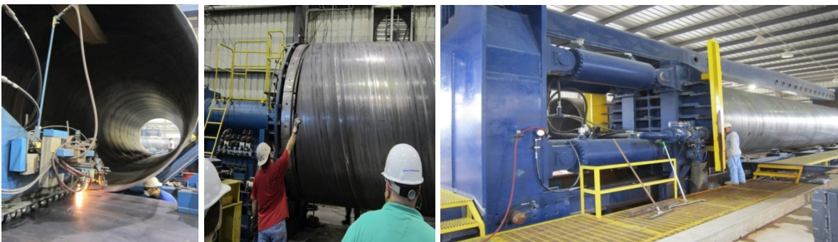
Figures 5a, b, c: Interior Submerged Arc Welding, Expanding Bell-End of Cylinder, Hydrostatic Testing of 108-inch Cylinder to 267 psi
