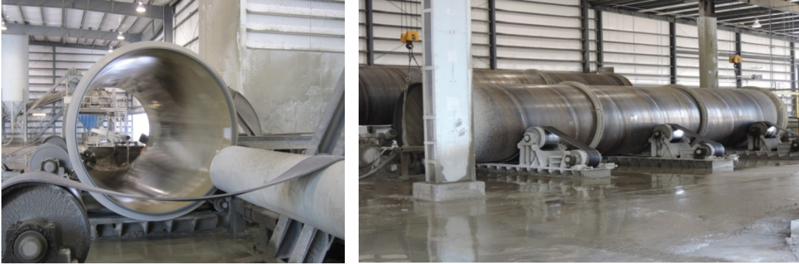
Figures 7a,b: Cement Lining of 25-ft Long Cylinders, 50-ft Long Cylinders
