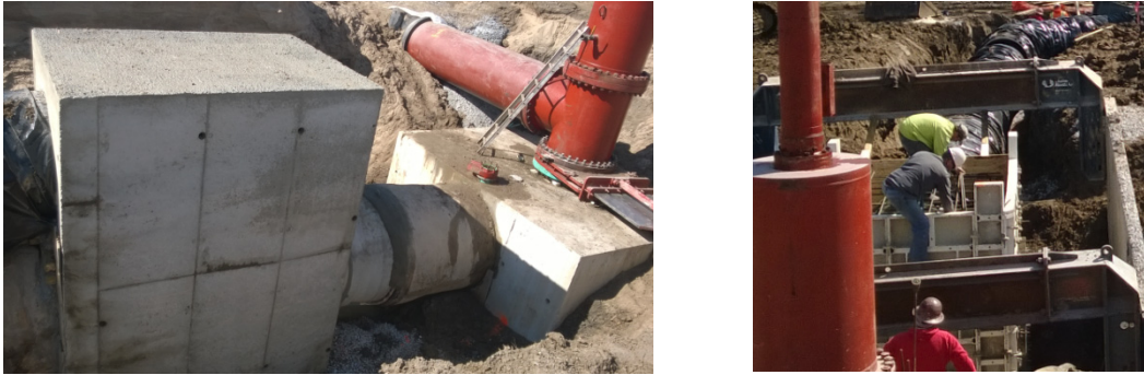
Figure 20 Fittings and connection encased in concrete Figure 21 Connecting new pipeline
