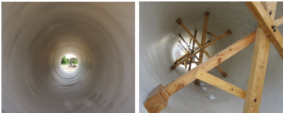
Figures 8a, b: Finished Interior of Lined Pipe, Installed 6-Point Stulling
