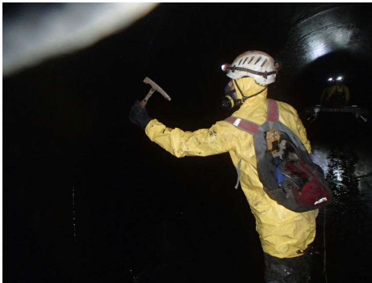
Figure 1. Inspector Sounding the 102-inch Force Main
