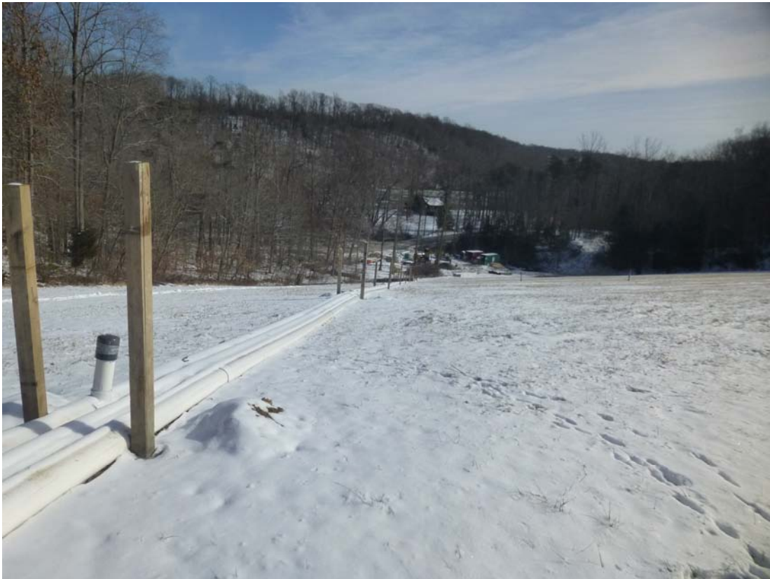
Figure 2. Downstream view from the top of the dam showing siphon pipes
