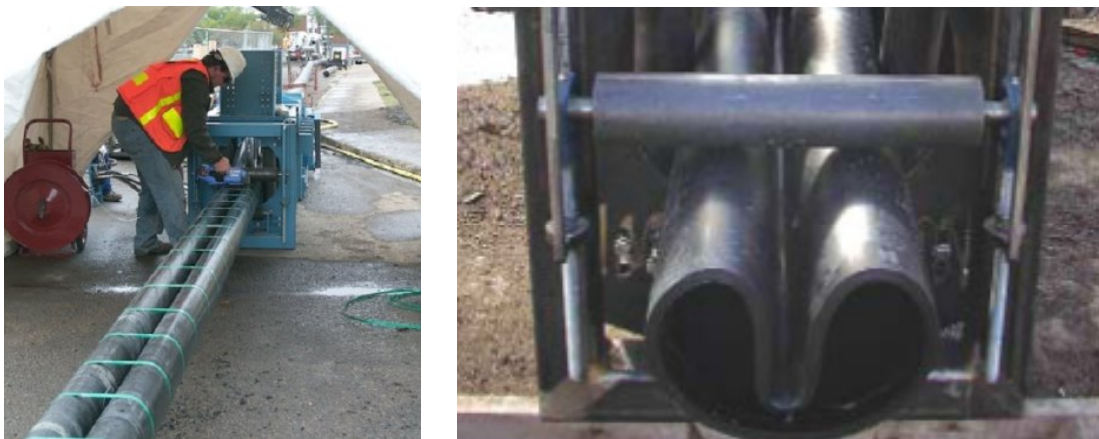
Figure 4. Fold and form process. (Source: Insituform)
