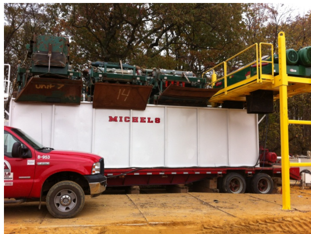
Figure 5 –Tunneling Material Dewatering Operations
