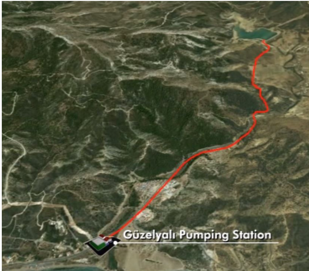
Figure 8: Güzelyalı Pumping Station
