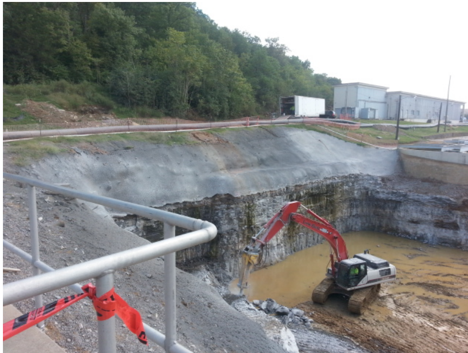
Figure 4. Location of pipeline in relationship to excavation slope
