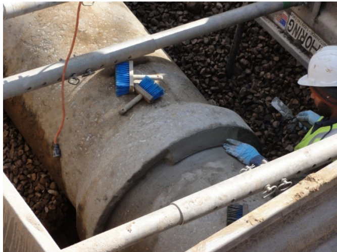
Figure 4. Repair of concrete joint with packed grout
