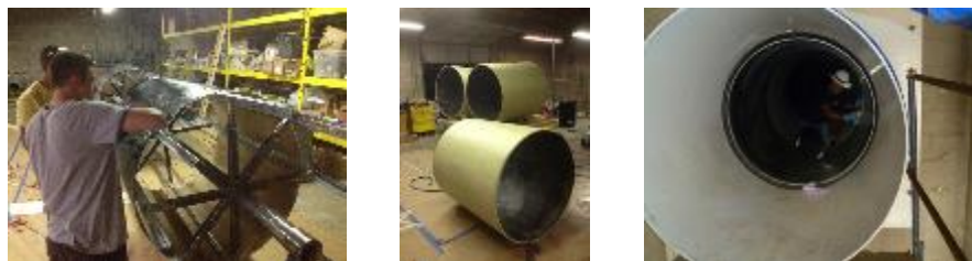
Figure 2. Making and installation of honeycomb-FRP pipe used for repair of pressure pipe.
