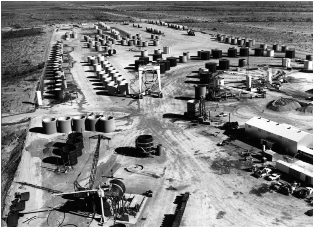
Figure 1 – 1978-79 Onsite Manufacturing Facility
