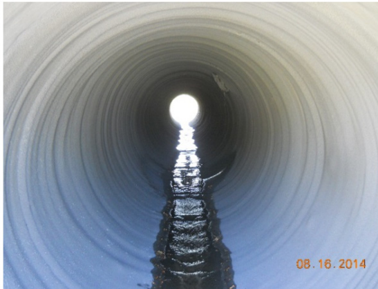
Figure 9. Finished liner.
