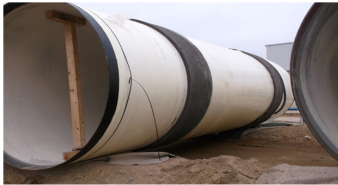
Figure 15: Two Mortar Bands on 25-ft Section of 108-inch Polyurethane Coated Steel Pipe
