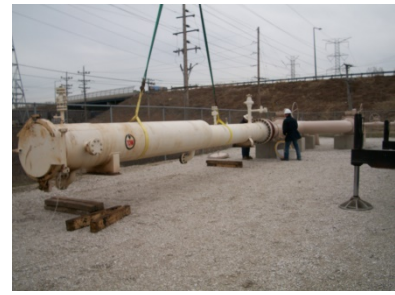
Figure 12 Launch connection point Figure 13 Unloading launcher Figure 14 Installing receiver
