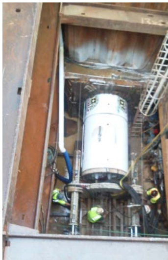
Figure 3. MTBM Launched from Shaft 6
