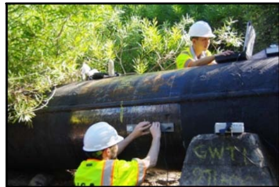
Figure 10. BEM scanning on exposed pipe section.
