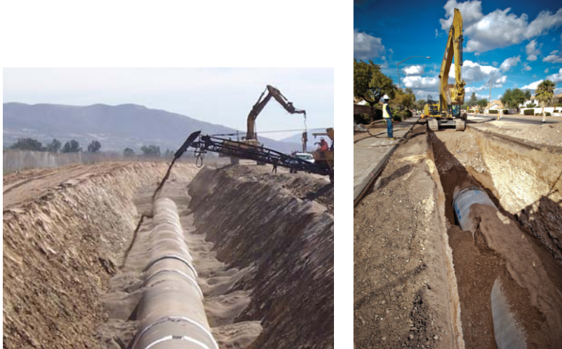
Figure 14 – Backfilling Large and Small Diameter Flexible Pipe
