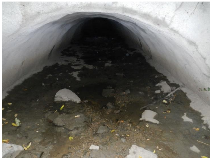
Figure 3. Photo Showing Shotcrete near North Street, Year 2013
