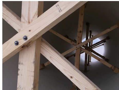
Figure 15: 5 sets of a 3-stull spider configuration
