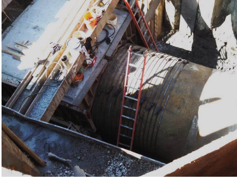
Figure 4. Tendon Repair of 102-inch PCCP
