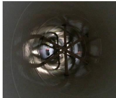
Figure 10: Two inside stull sets are visible
