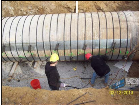
Figure 6 – EPT Tendons Being Installed
