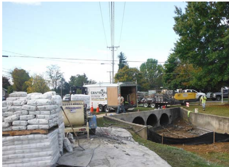
Figure 5: Minimal off-road staging area for equipment and materials
