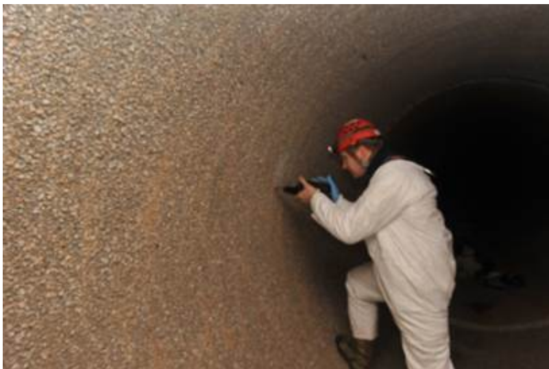
Figure 4. Evaluation of Inner Concrete Core via Rebound Hammer Test
