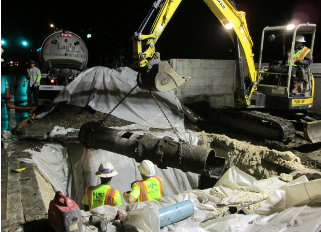
Figure 8. Red Bug Lake Road Existing Pipe at Tie-in Location
