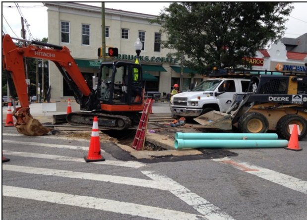
Figure 5: Open Trench Point Repair
