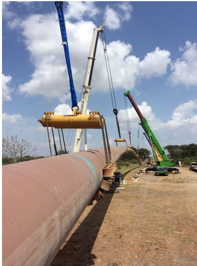
Figure 5: HDD Installation
