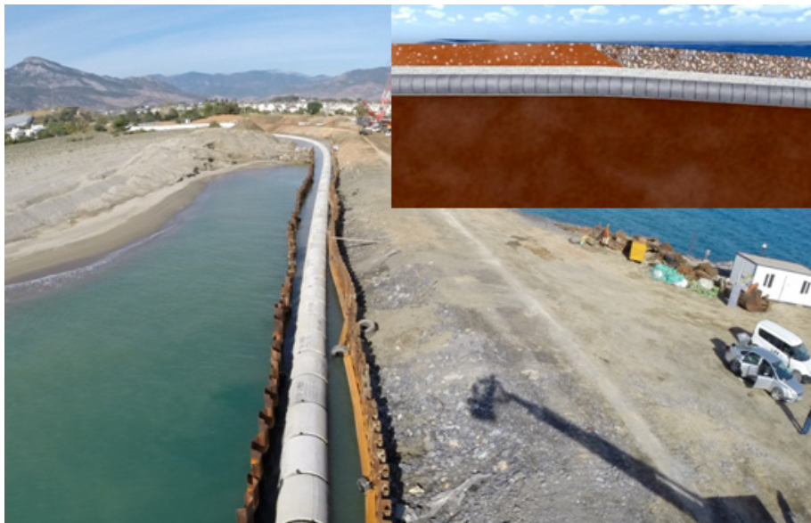
Figure 5: PE 100 Pipe In-Shore Transition
