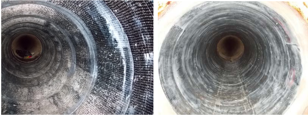
Figure 2. Completed Installation of CFRP on a Buried Pipeline
