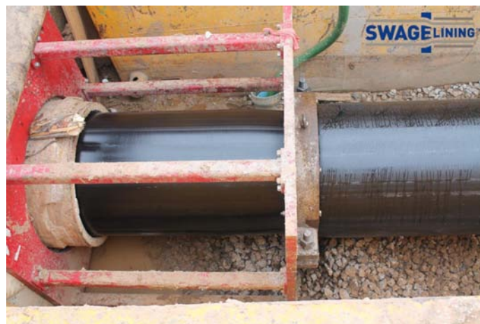
Figure 2: Swagelining™ process as HDPE is pulled through the reduction die.
