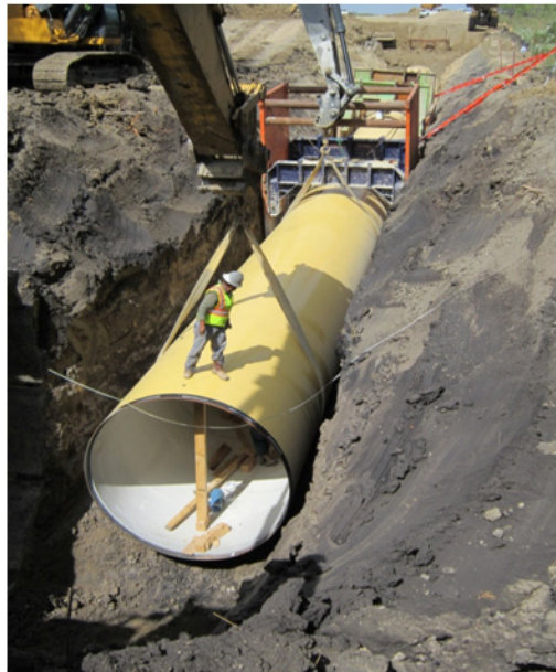
Figure 12: Pipe Handling in Trench
