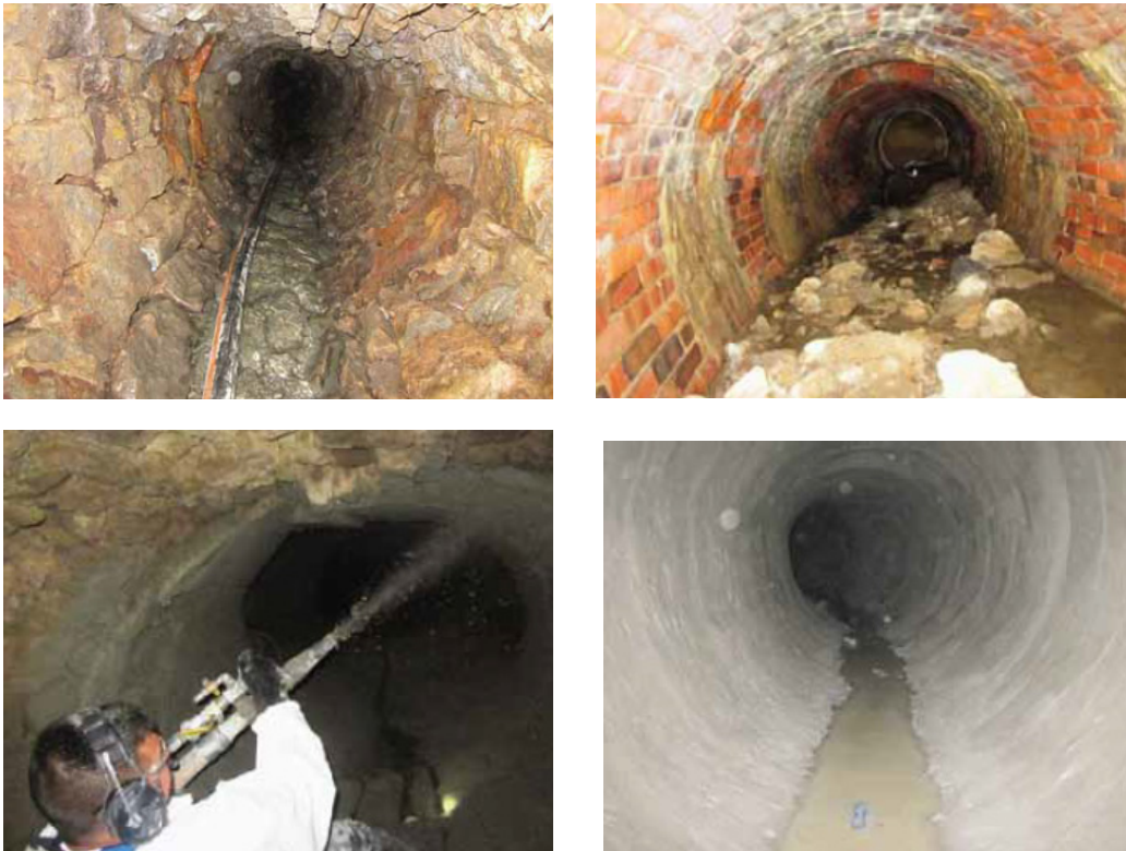
Figure 10: Images from the jobsite for the MSD in Cincinnati Ohio
