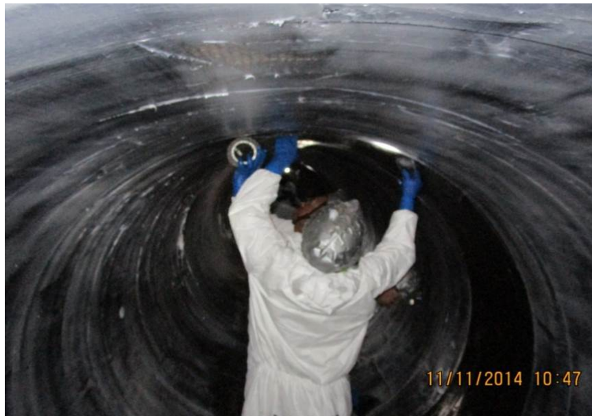
Figure 8. Application of hoop direction layer of CFRP
