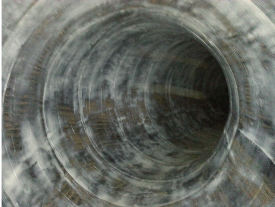
Figure 10. Completed CFRP installation at 45° bend
