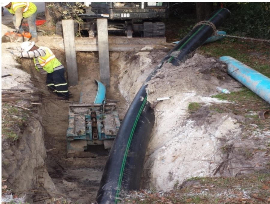
Figure 6. Pipe Bursting
