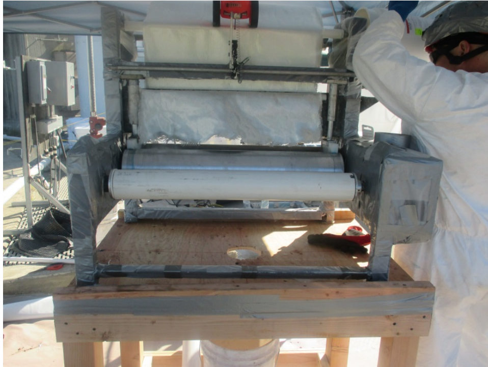
Figure 6. Glass fabric being saturated with a two-part 100% solid epoxy using a mechanical saturator
