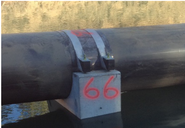
Figure 4 - Typical Precast Concrete Ballast represents a typical ballast. This is a departure from the more traditional two-piece ballast having concrete blocks both above and below the pipe, and proved to be an improvement that significantly facilitated ballast placement, and limited pipe rotation during placement.
