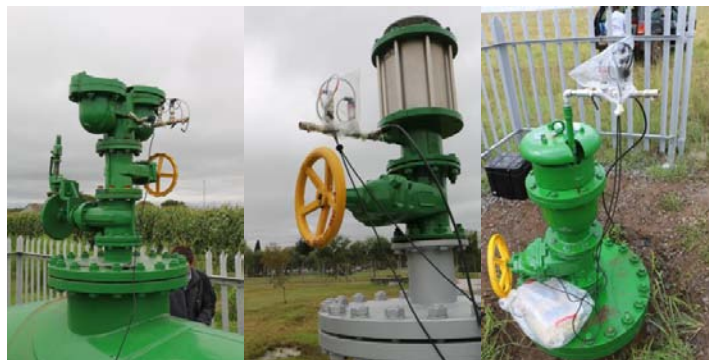
Figure 6: Typical pressure logging site arrangement
