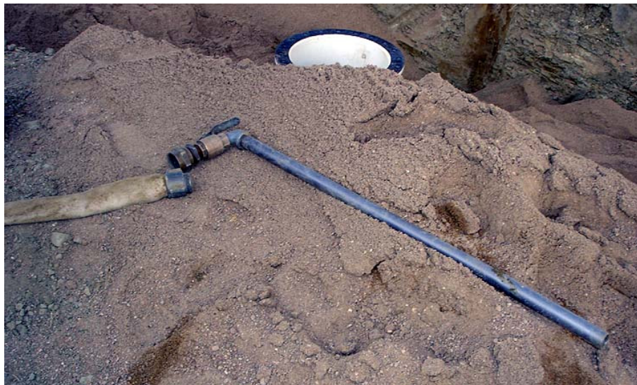
Figure 5 Rigid Insertion Tool for Jetting Water for Denver Water Board Project
