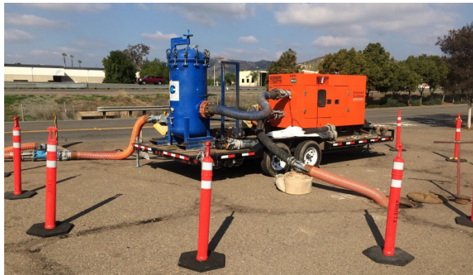
Photo 1. Typical Dewatering Operation
