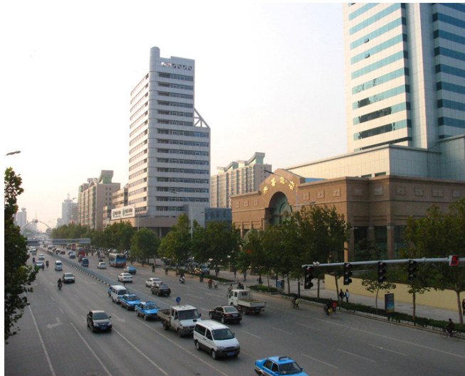
Figure 1. Location of the buried concrete pipes
