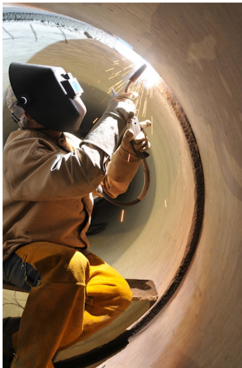
Figure 2. Field welding of interior double lap-welded joint.
