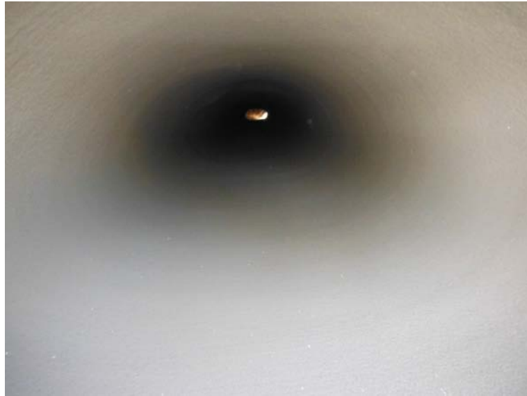
Figure 8: Smooth, seamless, watertight, and structurally sound rehabilitated culvert
