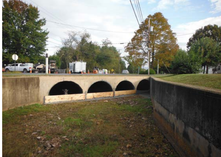
Figure 1: Four parallel culverts under Dogwood Avenue
