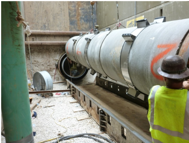
Figure 2 Casing Spacer/isolators
