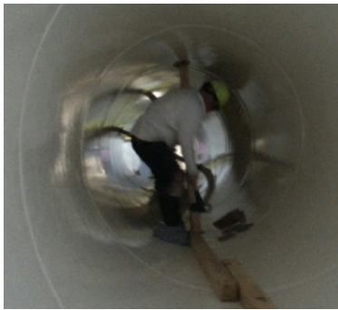
Figure 7: The Vertical stull is fit into place
