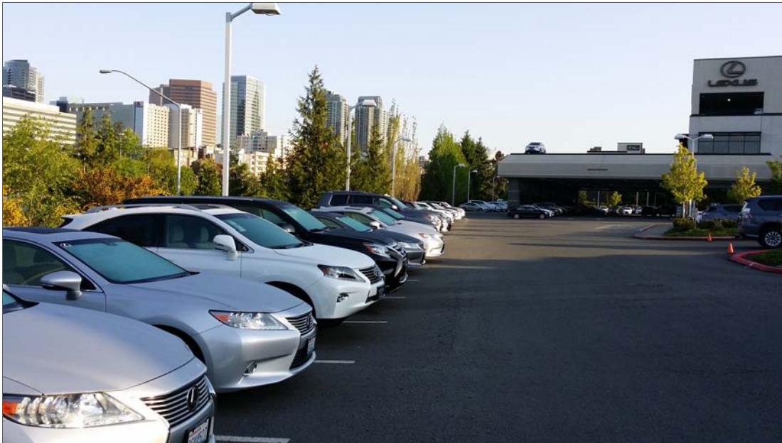
Figure 5. New sewer alignment through Lexus parking lot
