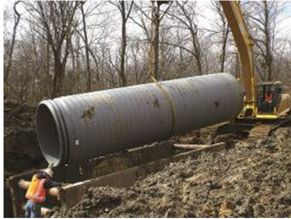
Figure 4. Moberly 60-inch Double Gasketed ASTM F2764 Installation
