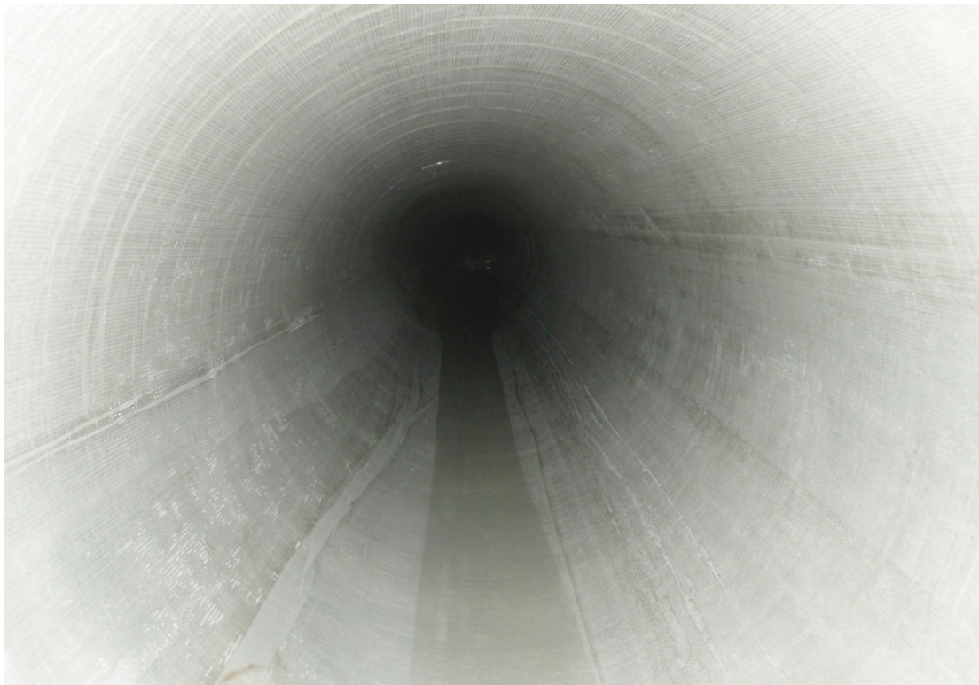
Figure 8. CIPP lining in pipe. (Source: MMSD)
