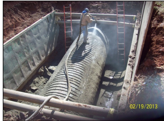
Figure 7 – Shotcrete Installation on EPT
