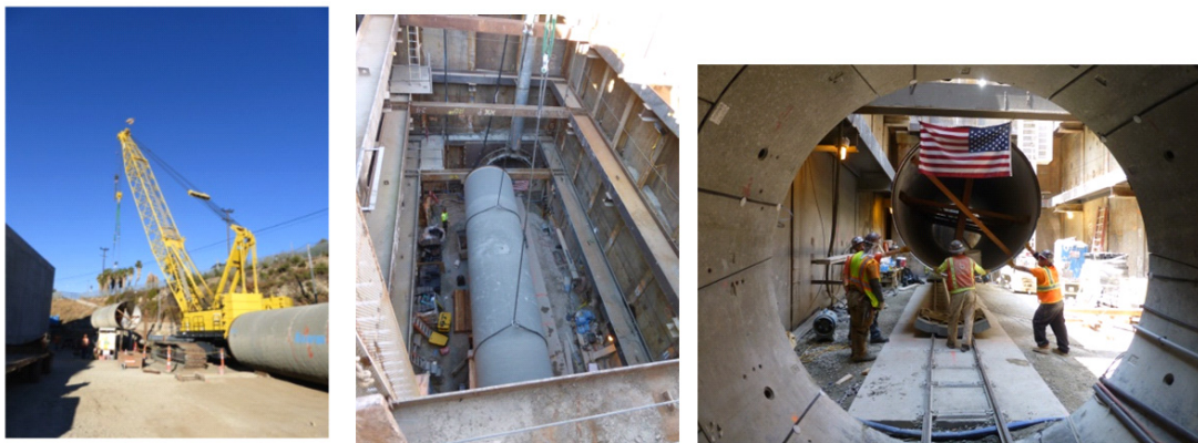
Figure 7a, b and c Pipe Installation
