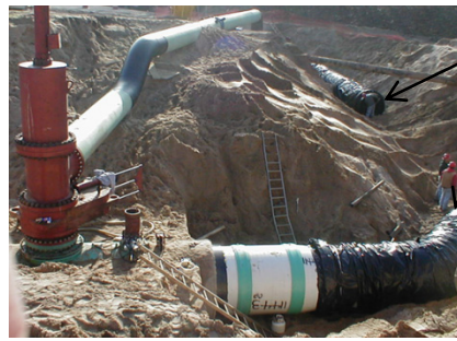
Figure 18 Plugging machine and bypass in operation
