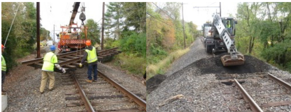
Figure 3: Removal of track for pipe installation
