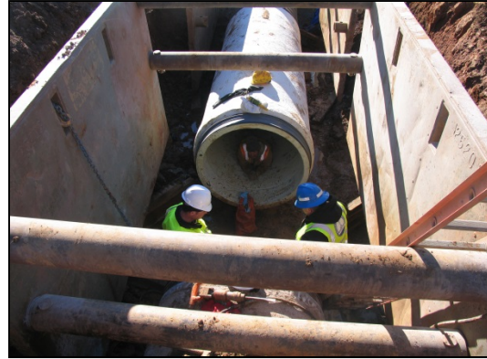
Figure 11 –Pipe Section Being Replaced
