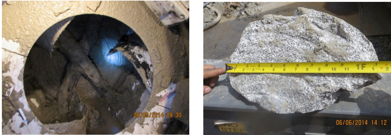
Figure 5. Boulder encountered during pipe jacking
