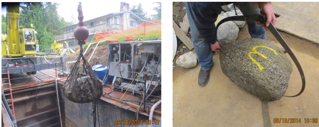
Figure 7. Obstruction (rock #3) being removed and measured
