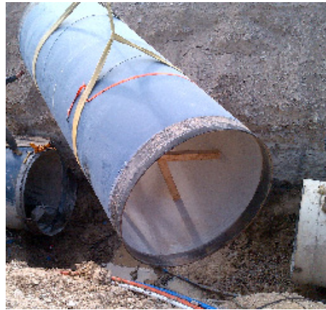
Figure 17: 66-in pipe joint being placed in the trench
