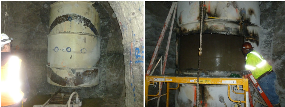
Figures 8a and 8b. Vertical Intake Shaft and Initial Cylinder Cutting.
