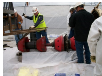
Figure 15 Brush cleaning pig after completing run Figure 16 DEF tool extracted from receiver
