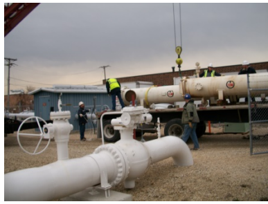
Figure 12 Launch connection point Figure 13 Unloading launcher Figure 14 Installing receiver
