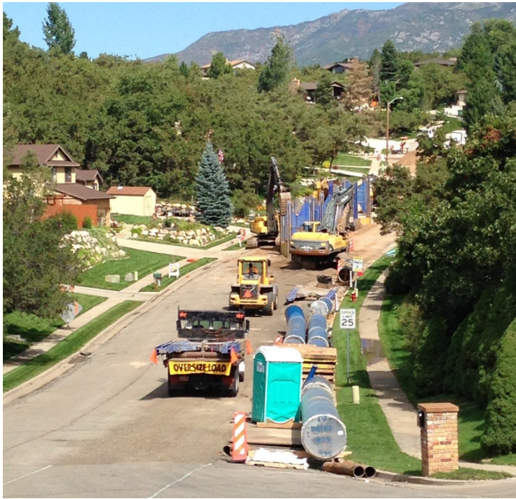
Figure 9. Pipeline Construction in Residential Streets
