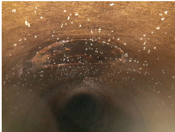
Photo 6. Quagga mussels attached to RCP
