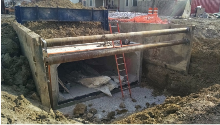
Figure 7. Precast Concrete Box Installation on North Street
