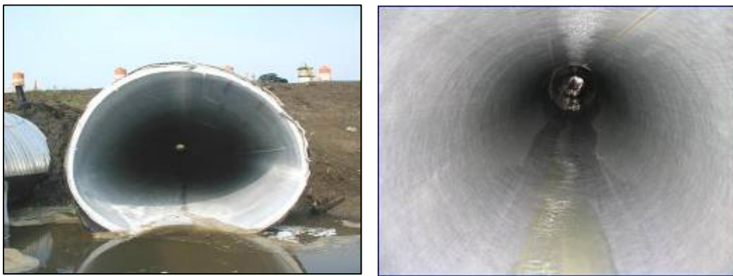
Figure 1. Completed Installation of CIPP
