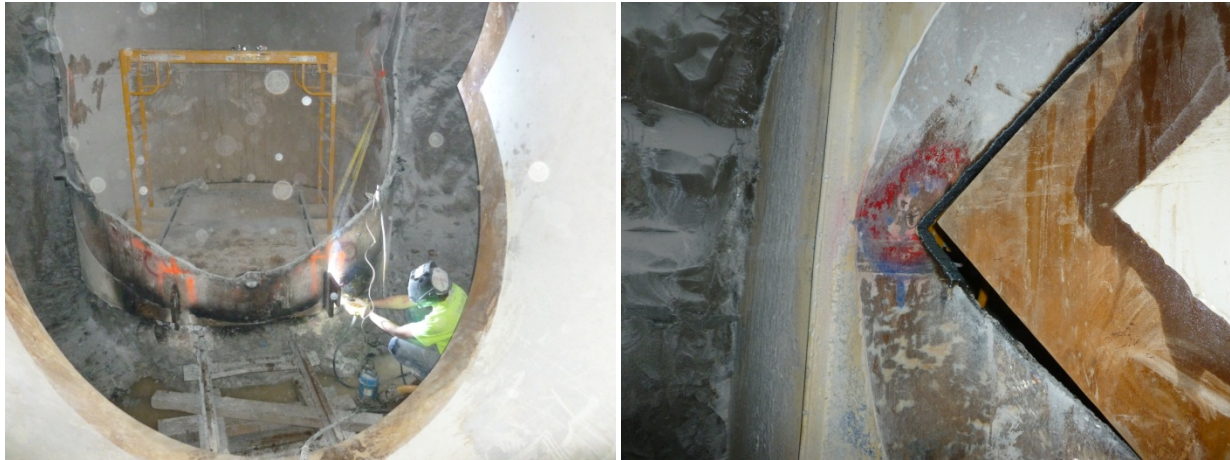
Figures 9a and 9b. Rough Cut-out and Trim Cuts.
