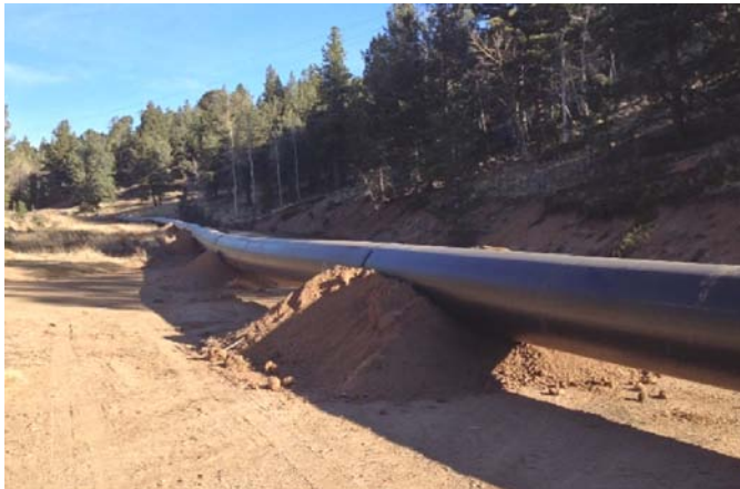
Figure 6- Fused HDPE Transfer Pipe prior to floating
