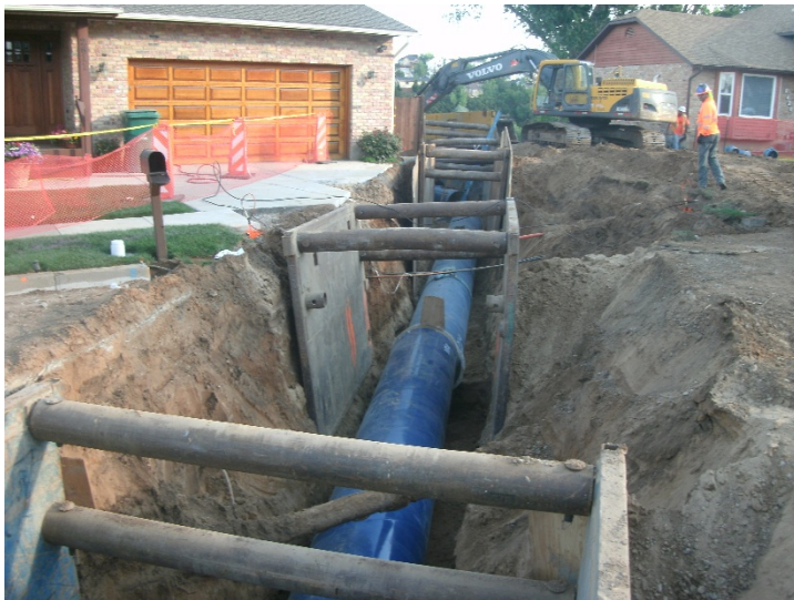
Figure 8. 36-inch Pipe Installation Near Residential Homes
