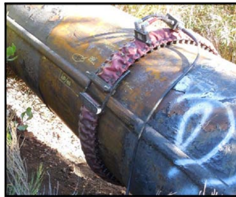
Figure 8. Guided wave testing on exposed reach near a riveted joint.
