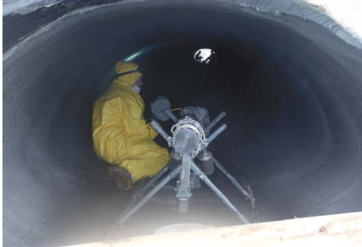
Figure 7: Spincaster and sled
