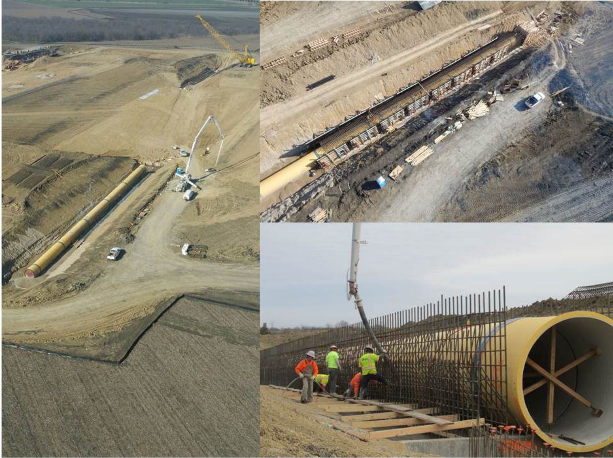
Figure 5 - Construction of Encasement on 108-inch Steel Inlet Pipe at JB3R
