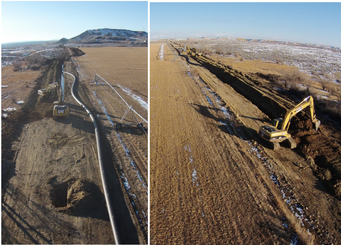
Figure 4. HDPE Pipe Installation
