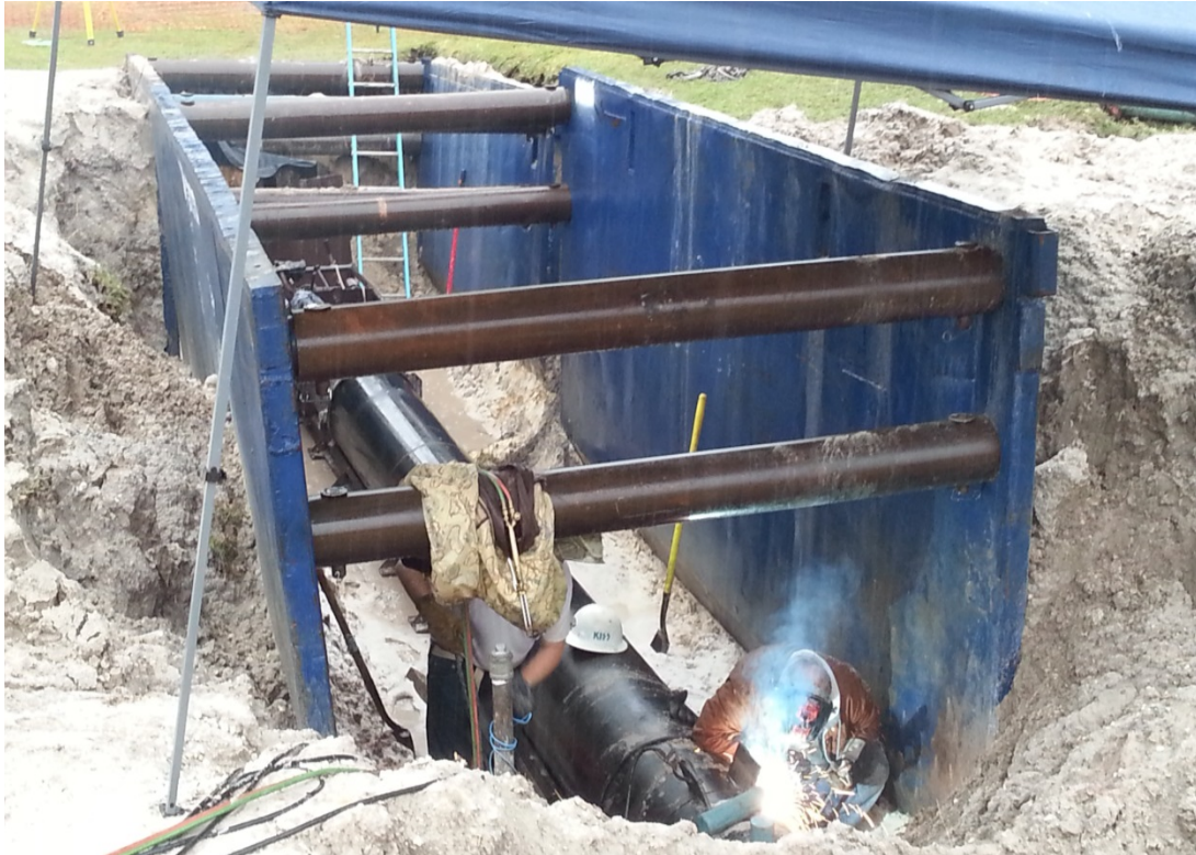
Figure 7. Welding Jack and Bore Casing
