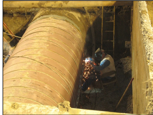
Figure 5 – Installed Repair Bands
