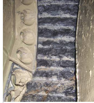
Figure 9. (above) Tunnel Face CH 576 m
