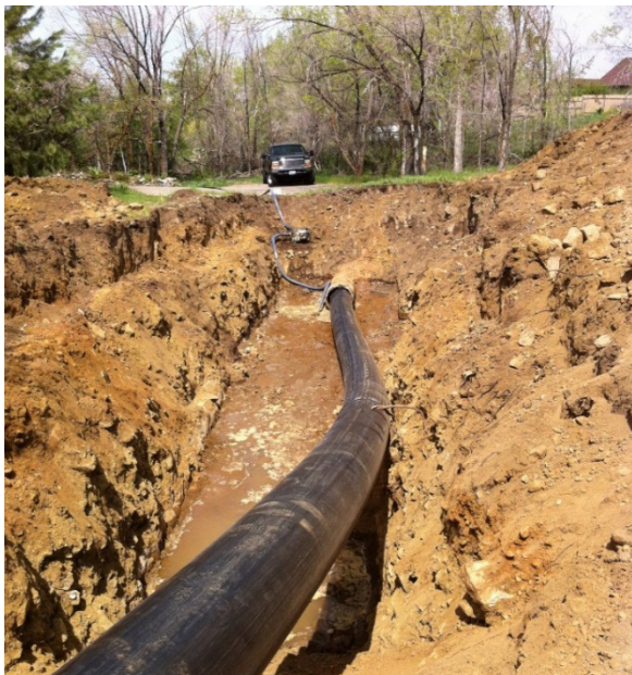
Figure 5- Slip-lining existing 27-inch RCP with 24-inch HDPE
