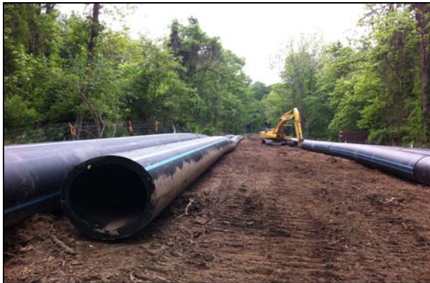
Figure 4: Staging of 400-foot sections of pipe
