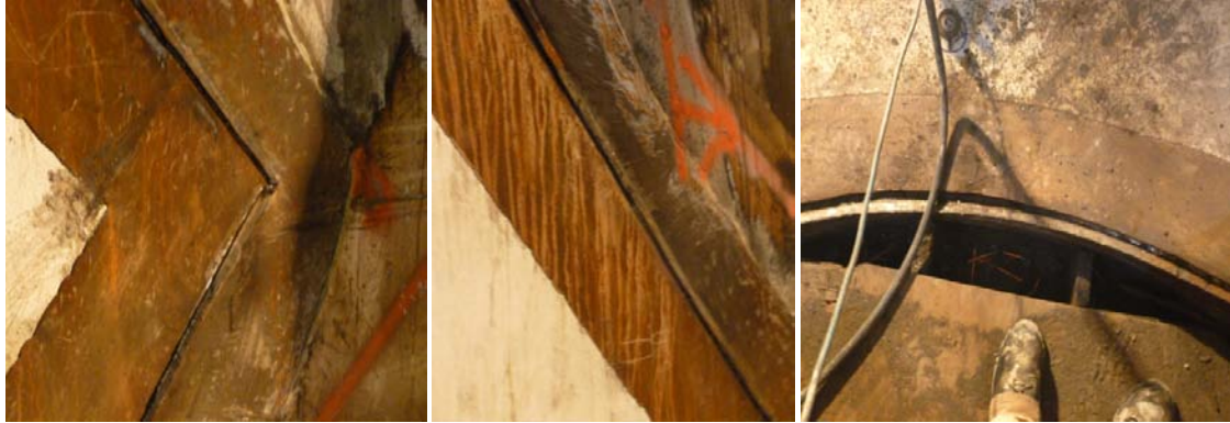
Figures 11a, 11b and 11c. Changing Joint Profile Around Circumference of Outlet.
