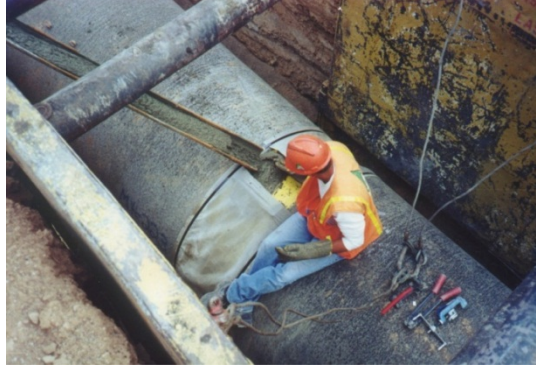
Figure 12 – Exterior Joint Grout
