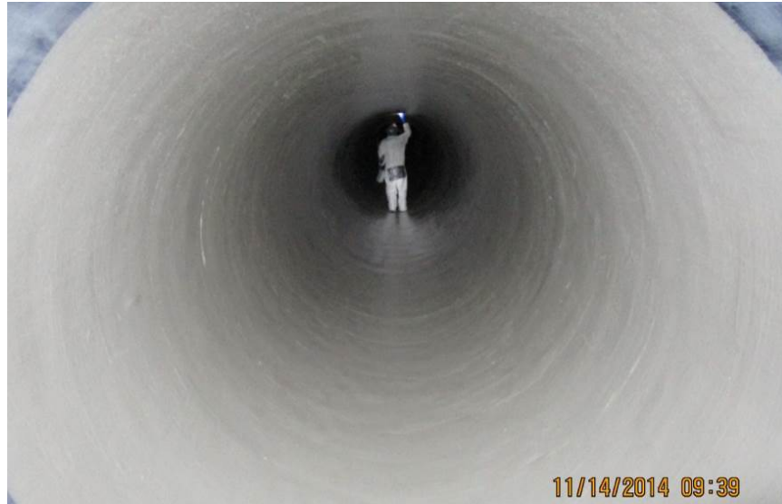
Figure 9. Inspection of the CFRP lining top coat
