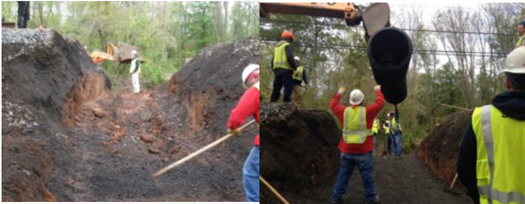
Figure 4: Preparation of trench and lowering of pipe
