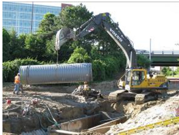
Figure 3. Backhoe Installation of ASTM F2764 Pipe
