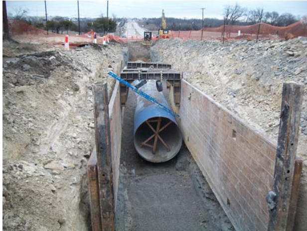
Figure 3. Backfilling Operations on the 96-inch Pipeline
