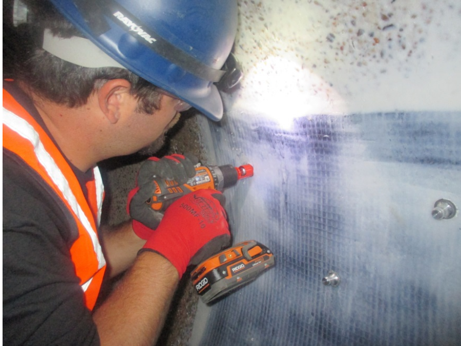
Figure 8. Pull test per ASTM D4541 being performed to verify surface preparation
