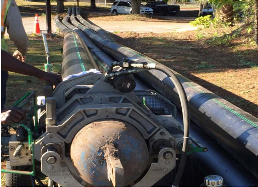
Figure 4. Fused HDPE Pipe
