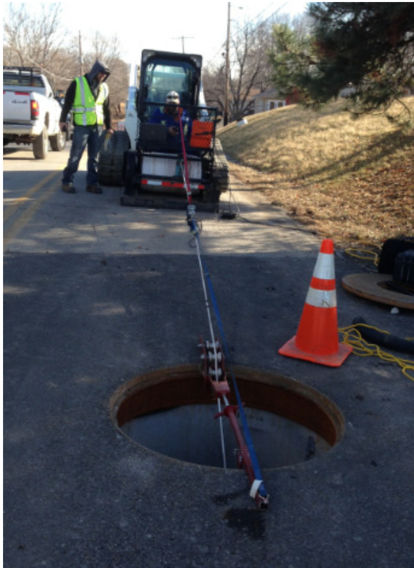
Figure 3. Winch Configuration for Inspection
