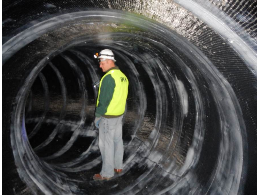
Figure 3. Inspection of the Installed CFRP Lining, prior to Top Coat Installation
