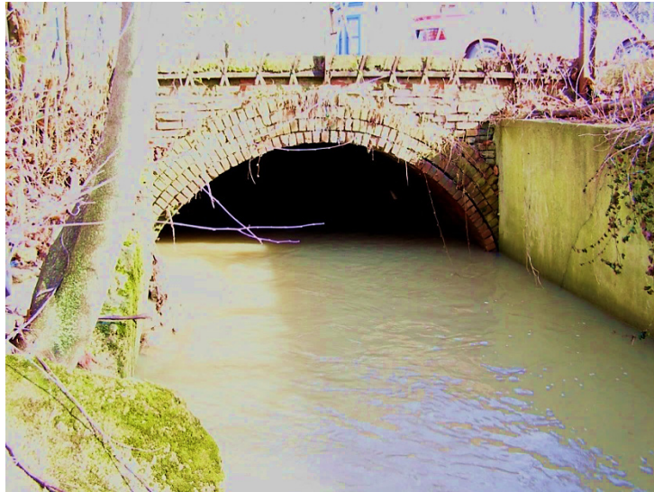
Figure 1. Photo of Original Potts Ditch at North Street
