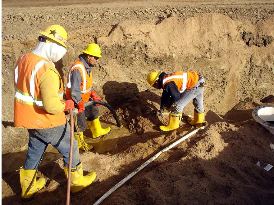
Figure 4 Using Jetting Insert and Vibration on Denver Water Board Project
