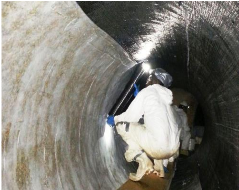
Figure 1. Typical process for Installation of CFRP inside a pipeline
