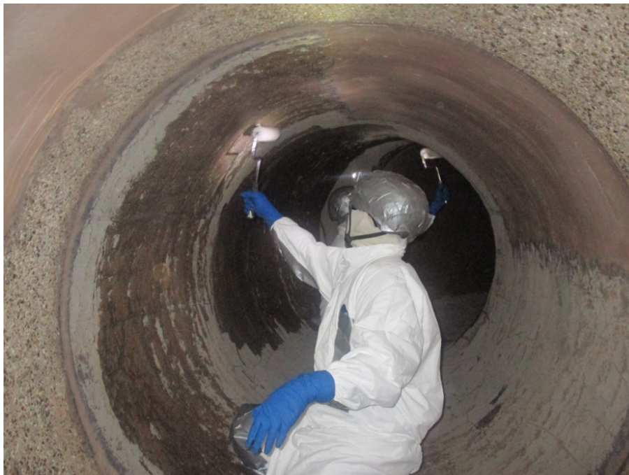
Figure 9. Primer epoxy being applied to concrete substrate adjacent to hole repair
