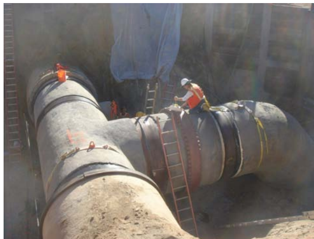
Photo 8 - Testing Of Assembly
