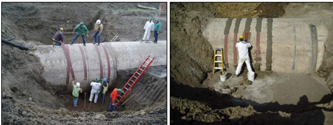
Figure 6 - Steel support band installation
