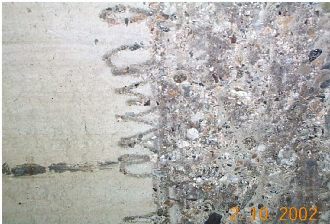
Figure 1 - surface preparation to pipe wall
