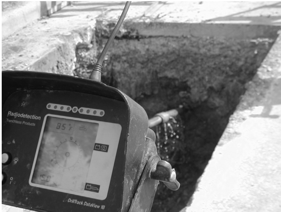
Figure 3 – Horizontal Directional Boring Equipment
