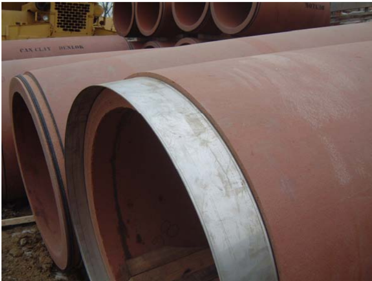
FIGURE 5 VCP Jacking Pipe
