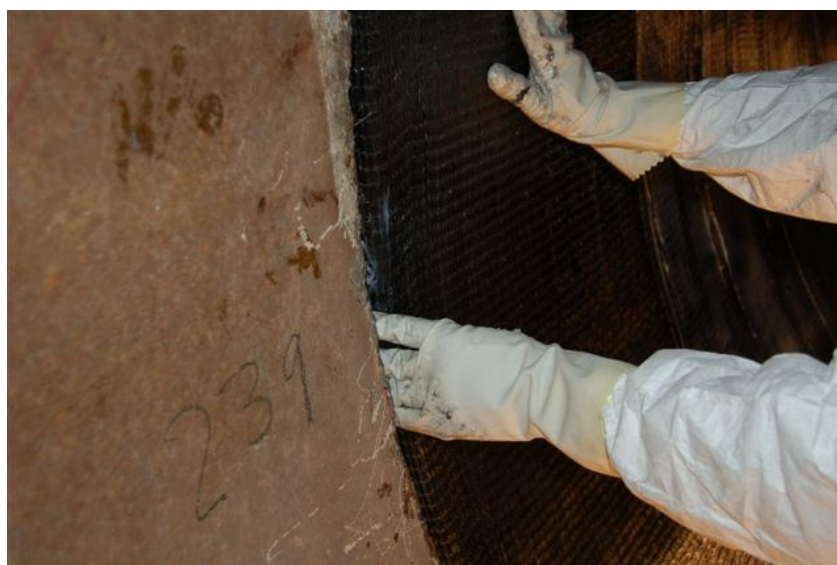
Figure 10 – Sealing of the Liner to the Steel Cylinder
