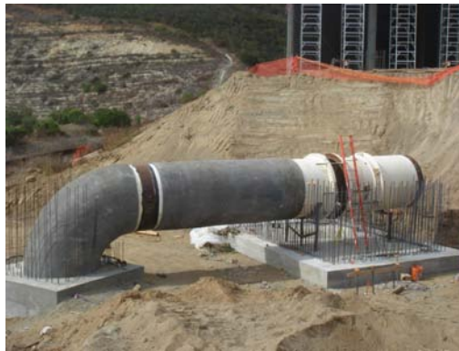
Photo 2 – 72-inch Yard Piping
