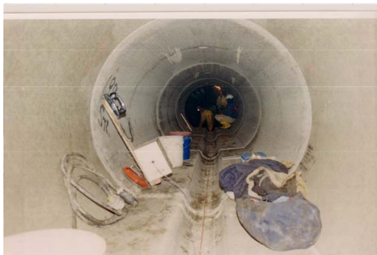
FIGURE 4 RCP with Cunnette installed in tunnel
