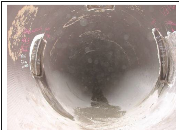
FIGURE 1 Typical Internal Surface Preparation for Non-Destructive Testing
