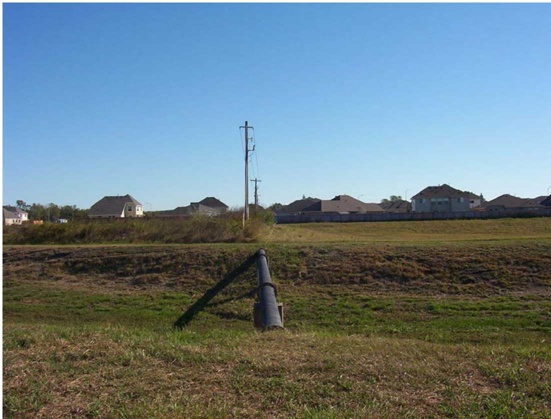
Figure 5: HCFCD with Existing 12-inch Force Main Aerial Crossing
