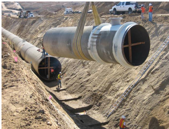
Figure 7. Bedding preparation and installation of 120-inch WSP for pipeline No.6.
