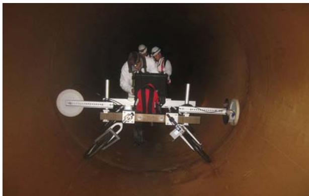
Figure 2: Electromagnetic inspection of the 102-inch Providence aqueduct
