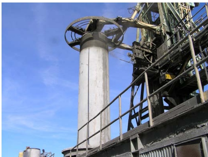
Figure 8. Pre-stressing Wire Being Placed on Newly Cast 54" PCCP
