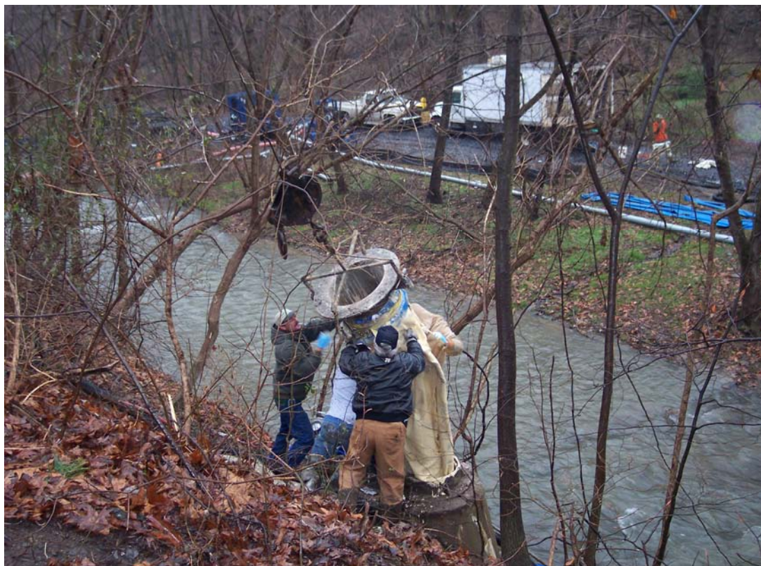
Figure 4 Installation of Cured-in-Place Manhole Liner
