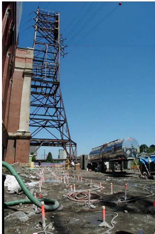
Figure 3. Sleeve port pipe for chemical grout along 54-inch consolidation conduit alignment.
