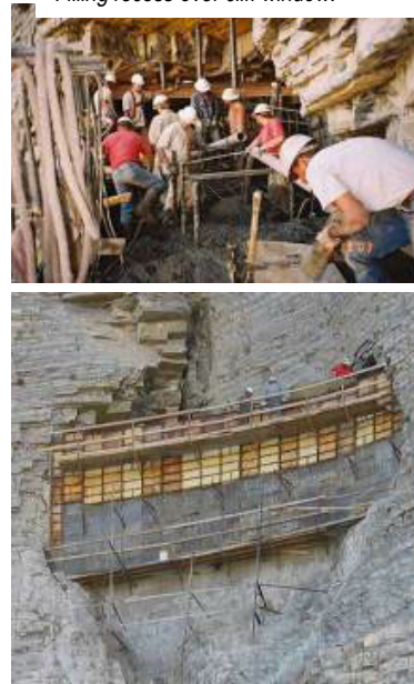
FIGURE 9 Filling recess over cliff window.
