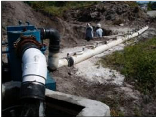
Picture 2: Well Pointing
