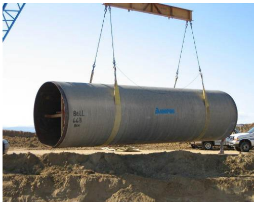
Figure 6. Unloading 120-inch mortar coated WSP for MWD's Pipeline No. 6.
