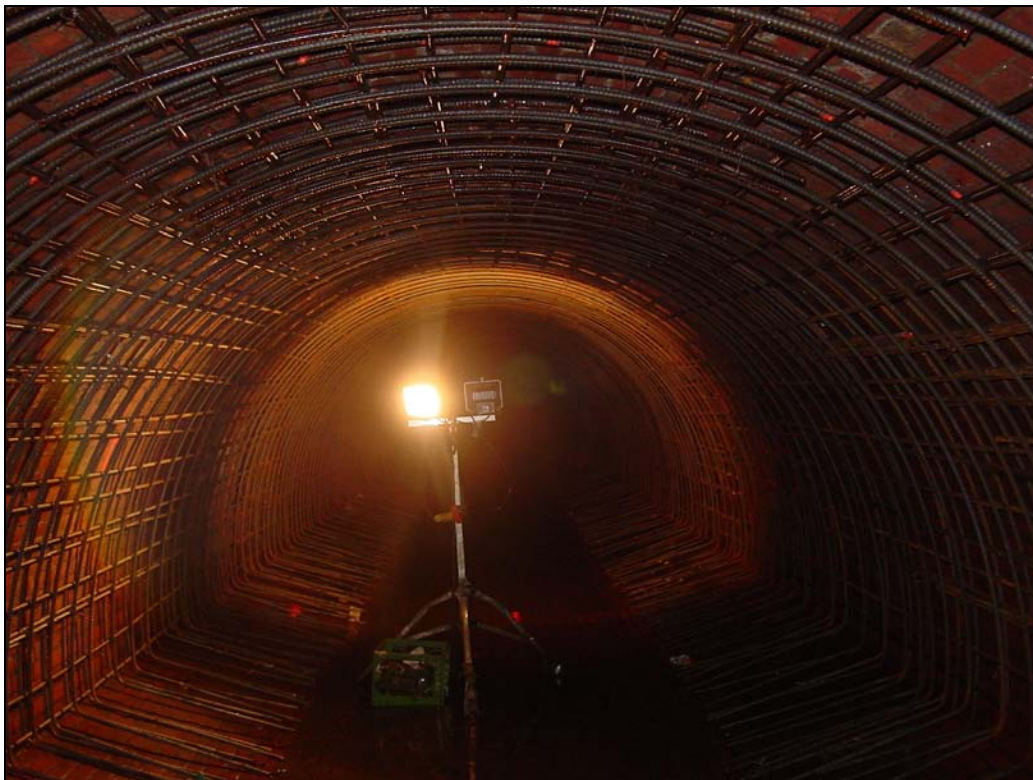
Figure 4 showing the steel reinforcing
