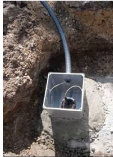
Picture 3: Accelerometer w Housing (no lid)
