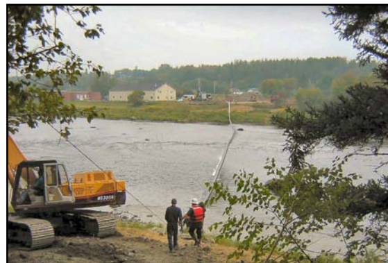
Photo 2: Towing pipe across river looking west
