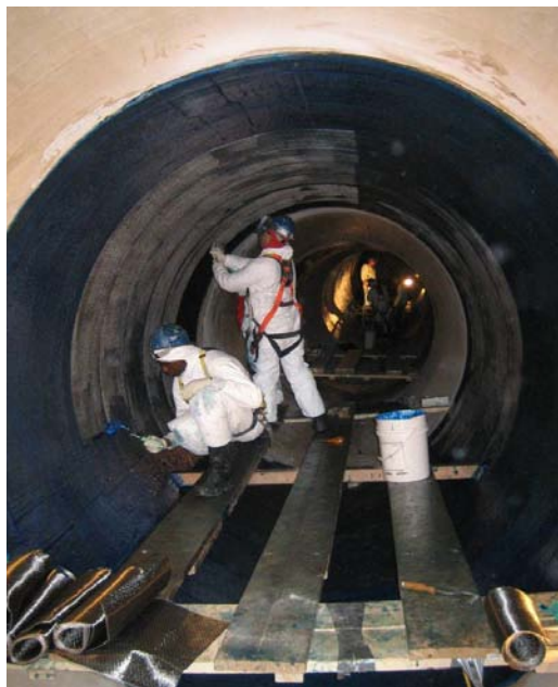
Figure 5: 2006 carbon fiber repairs
