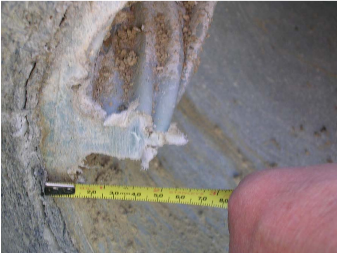
Figure 4: Close up of CIP liner fold.
