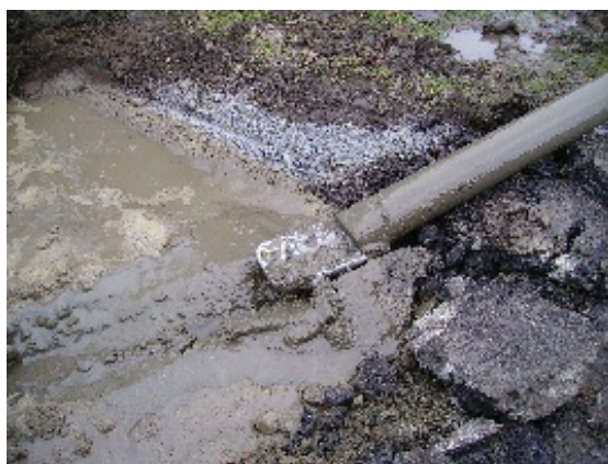
Spoon-style Bit suitable for use in wet clay
