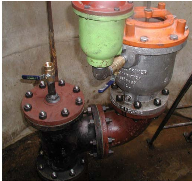
Figure 5 - Acoustic Emission Testing, introduced in 1996 requires insertion of hydrophones at regular intervals (Pressure Pipe Inspection Company photo)
