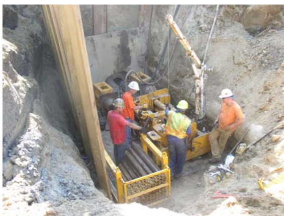
Figure 2 – Pipe Bursting Receiving Pit (Left) and Pipe Entry (Right) Pit
