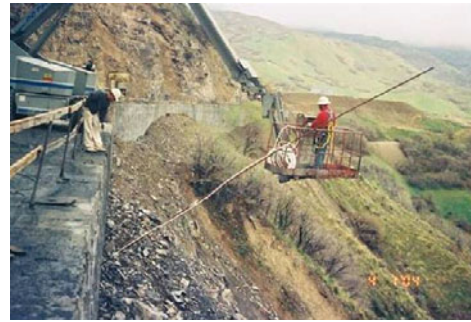
FIGURE 12 Installing rock bolt.
