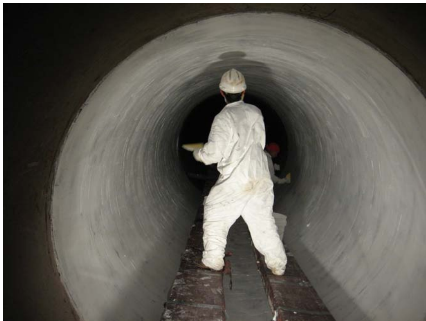
Figure 7 – Application of the Potable Water Coating
