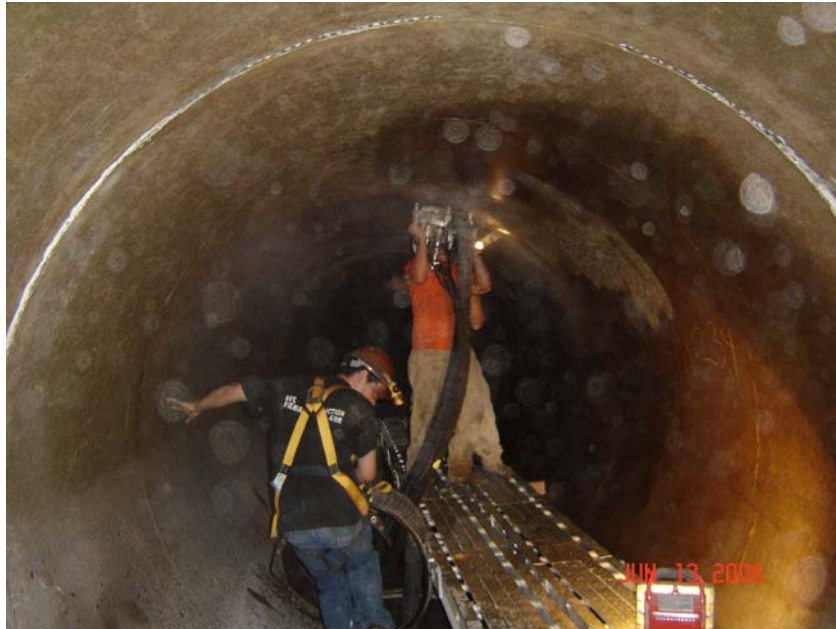
Figure 4 – Interior Cleaning of the Pipe Surface
