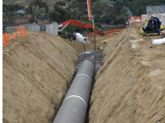
Photo 10 - CLSM Placed In Narrow Trench
