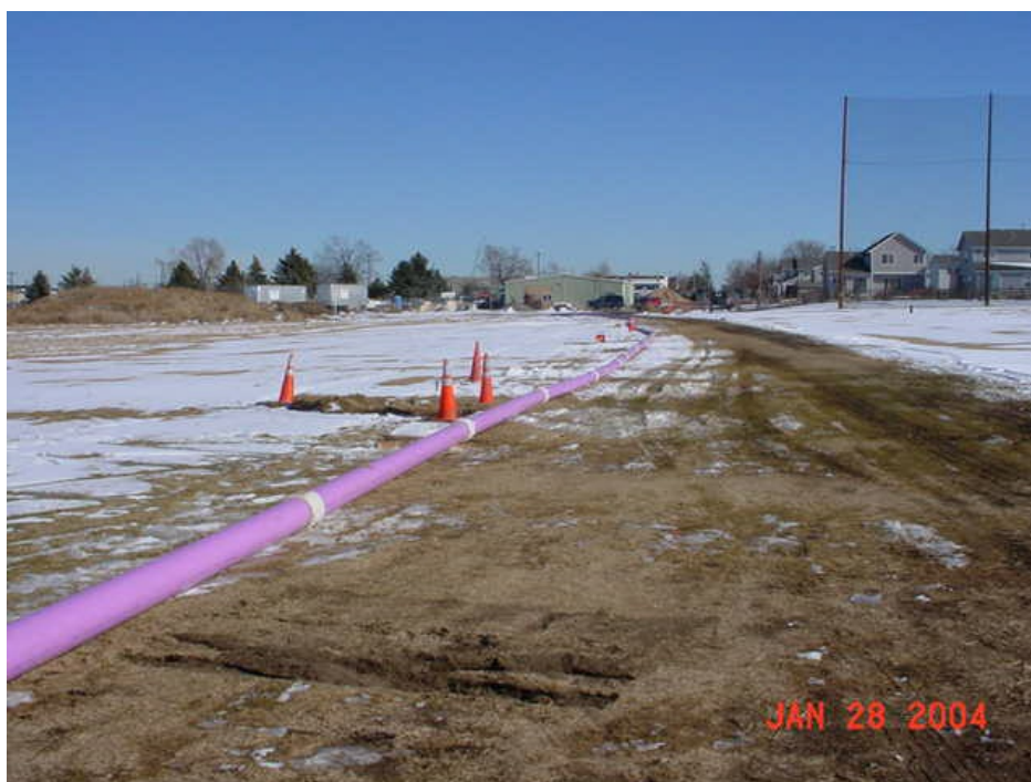
Figure 5 – Pipe laid out in the string method for HDD installation.
