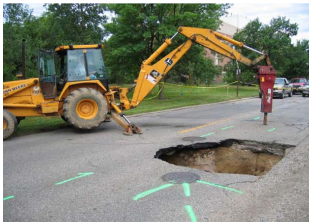
Figure 1 – MSU Service Road Pipe Replacement Construction
