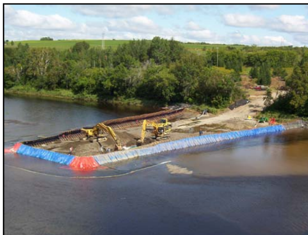
Photo 5: Aroostook River water main crossing, Presque Isle, Maine
