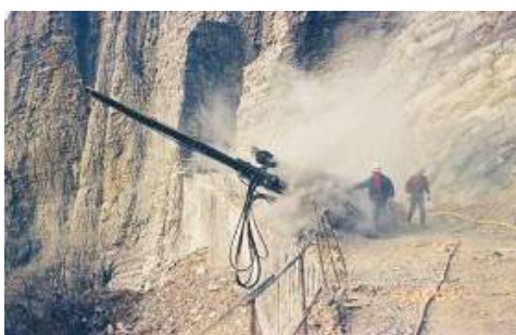
FIGURE 10 Drilling rock bolts with sleeves through encasements.
