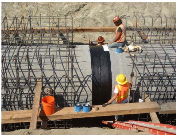
Photo 4 – Tape and Mortar Coating
