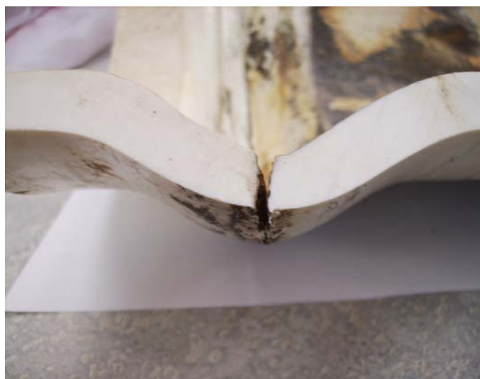
Figure 5: Pipe Samples from Original Force Main
