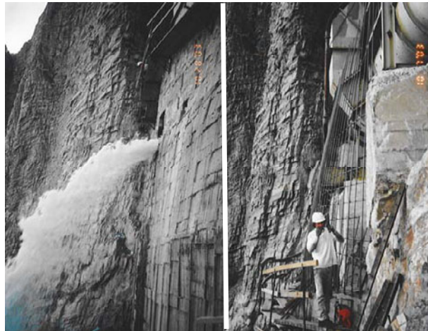
FIGURE 8 Textured concrete face at Spillway after (spilling) and before concrete placing.
