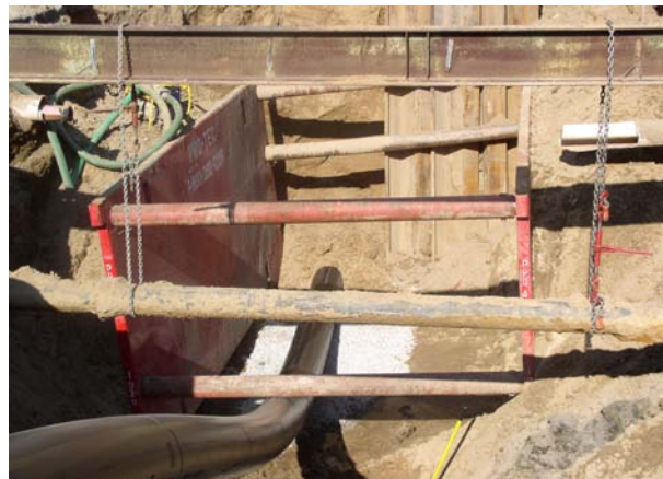
Figure 2 – Pipe Bursting Receiving Pit (Left) and Pipe Entry (Right) Pit
