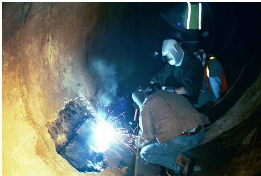
Figure 9 – Welding Repair of Fractured Steel Cylinder
