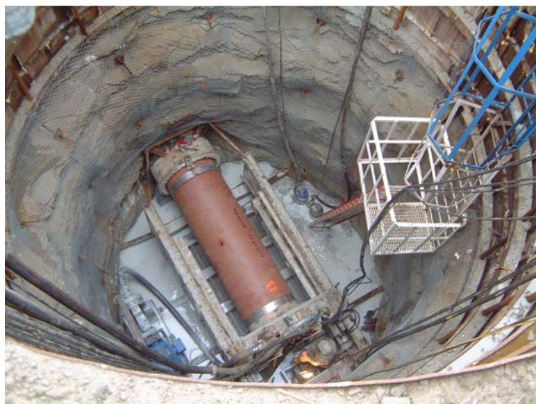
FIGURE 6 VCP Jacking Pipe Being Installed by Microtunneling in Rock
