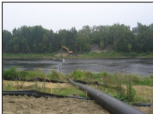
Photo 1: Towing pipe across river looking east
