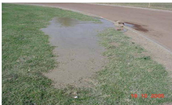
Figure 5 - Typical Slurry Frac-out
