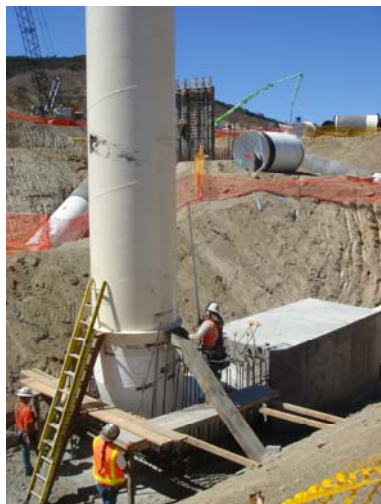
Photo 3 – Tape or Epoxy Coating
