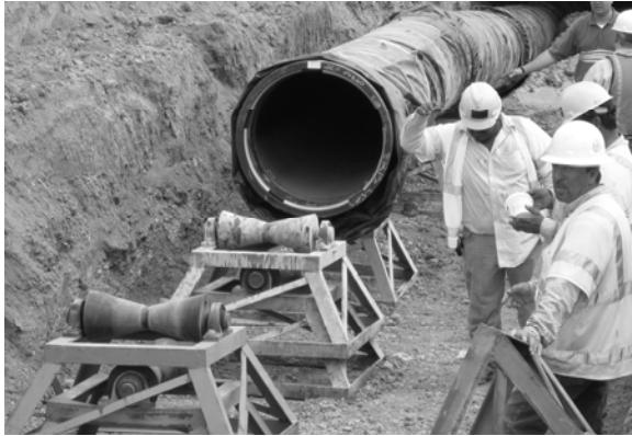
Figure 3 - Cartridge Assembly On Pipe Rammer
