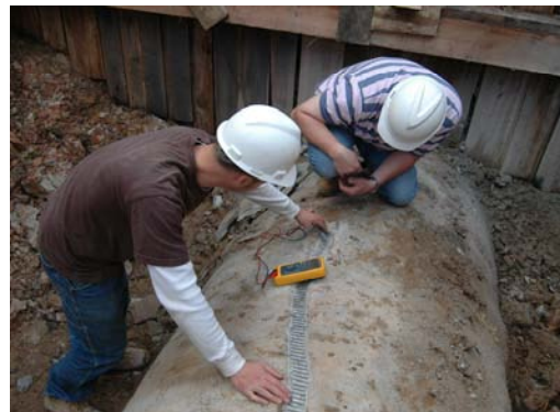
Figure 3: Resistivity testing being performed on a 54-inch pipe
