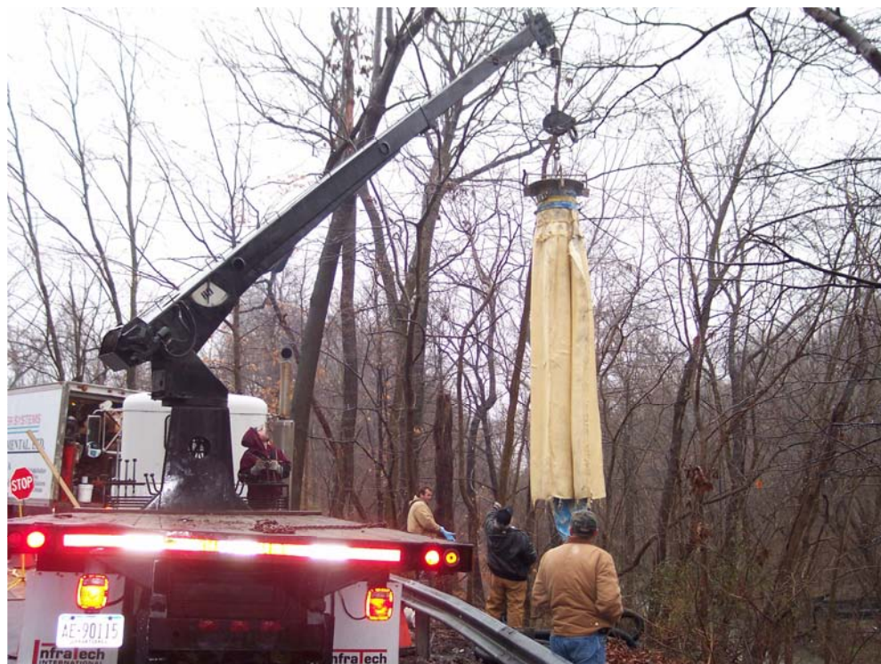
Figure 3 Cured-in-Place Manhole Liner
