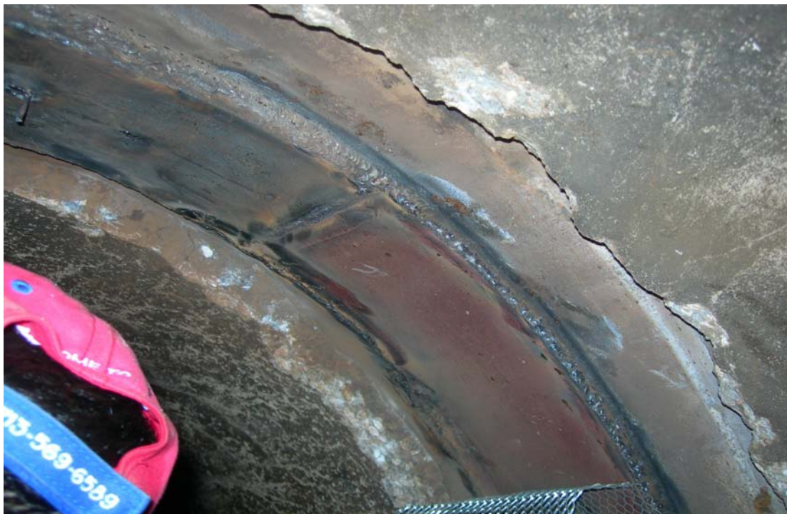
Exhibit 7: Completed internal butt-strap repair
