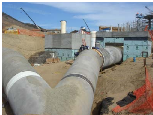
Photo 1 – 84-inch Yard Piping
