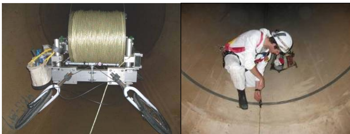
Figure 3 & 4 – Fiber Optic Cable Installation
