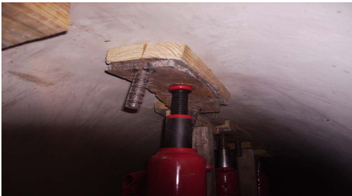
Photo 1: Hydraulic jacks with rubber and steel padding inside MK #35 along Alameda.
