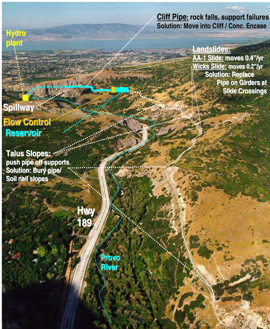
FIGURE 5 1998 photo of the lower 3.2 km (2 miles) of Provo Canyon with pipe reliability issues and solutions noted.
