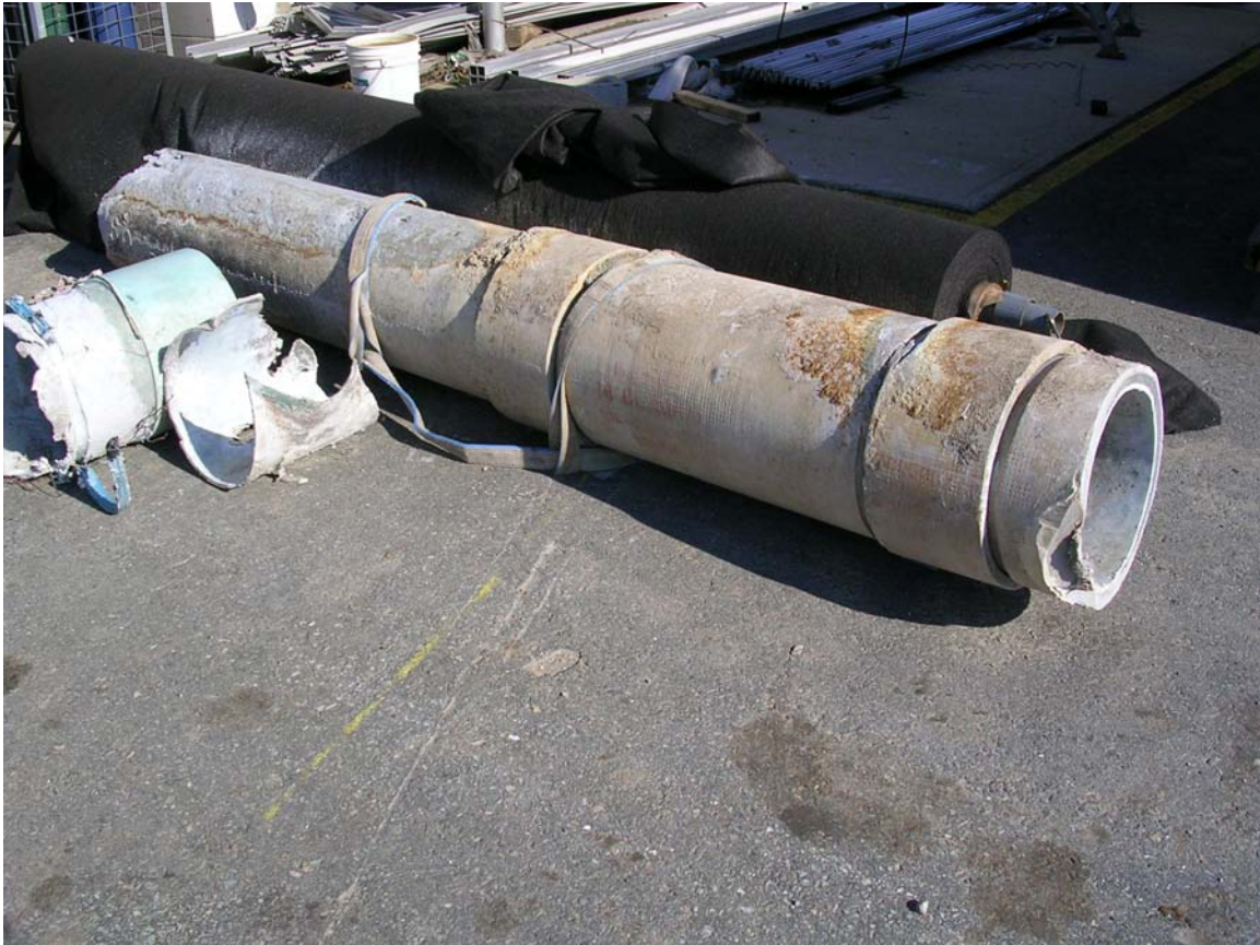
Figure 2: Exterior of removed 356mm (14-inch) diameter Asbestos Cement pipe.
