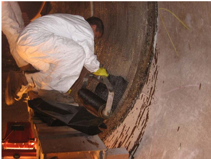
Figure 5 –Carbon Fiber Material Application
