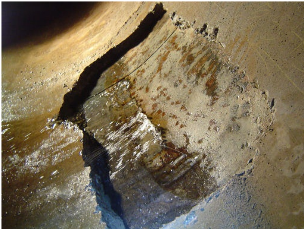
Figure 1 - Urgent Repair Pipe Mark 543
