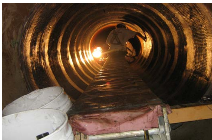
Figure 6. Lining of 54-inch PCCP Main with Carbon Fiber
