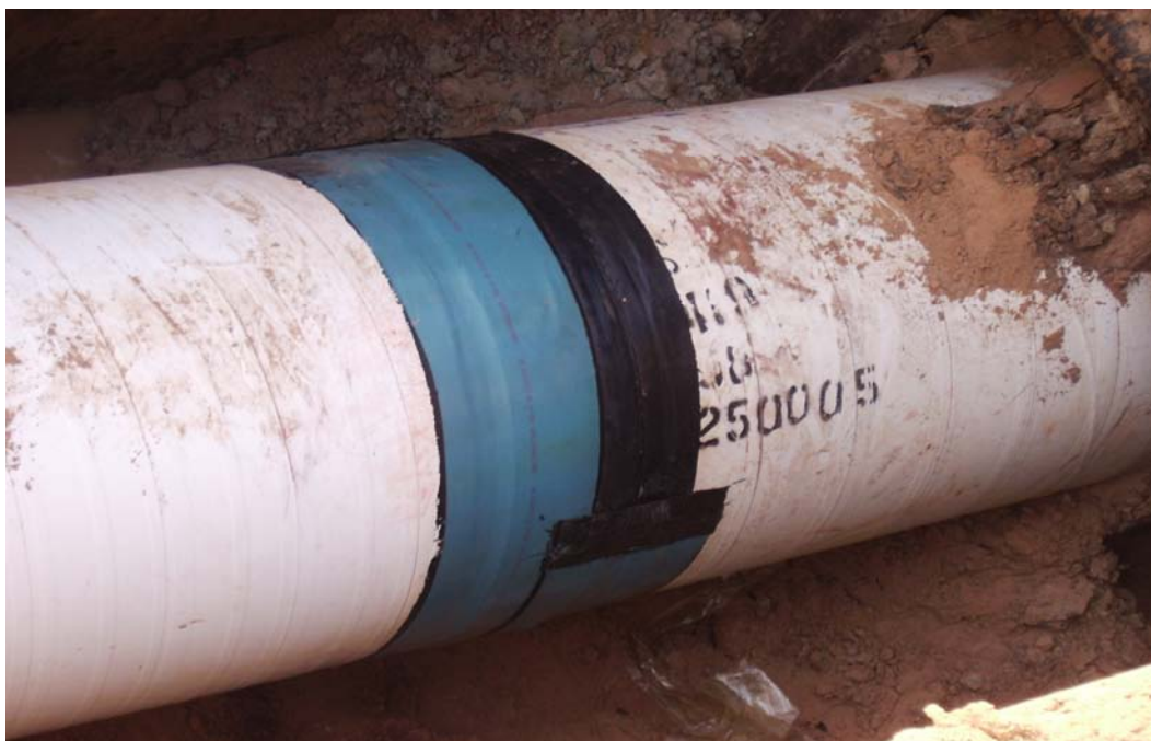
Photo 5: Heat-shrink tape placed at the joint between MK #94 and MK #95.
