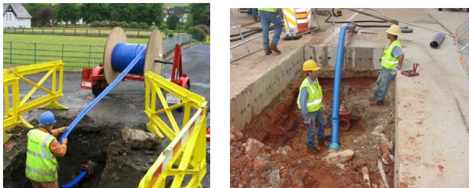
Inserting Folded Liner and Expanding Liner
