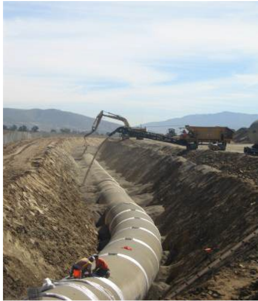
Figure 9. Water jetting of the backfill can be observed in the background.
