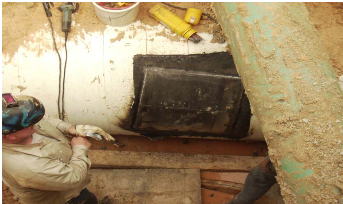
Photo 6: Steel patch being welded over removed portion of steel on MK #31
