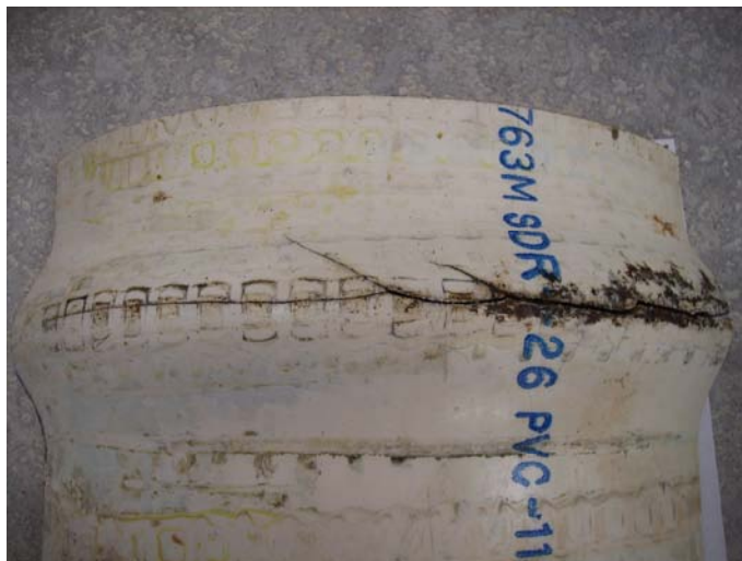
Figure 6: Pipe Samples from Original Force Main
