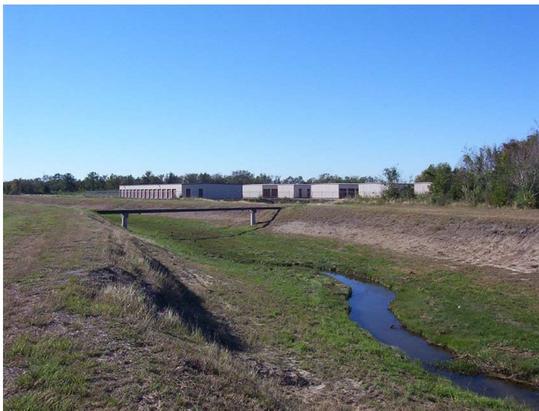
Figure 4: HCFCD with Existing 12-inch Force Main Aerial Crossing
