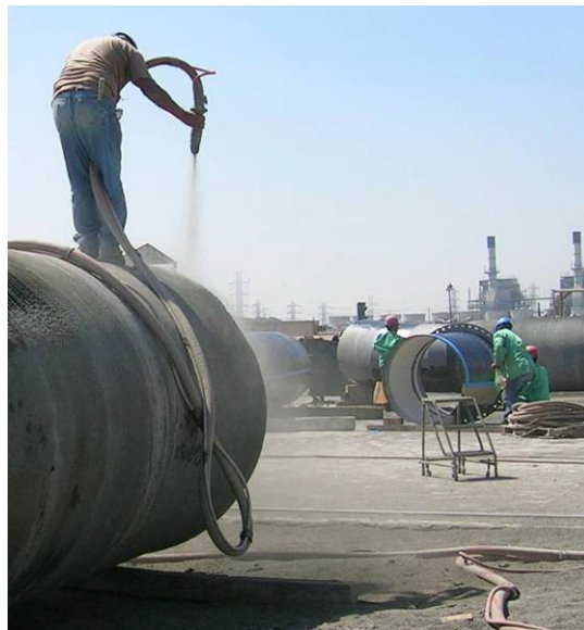
Figure 2. Pneumatic mortar application.
