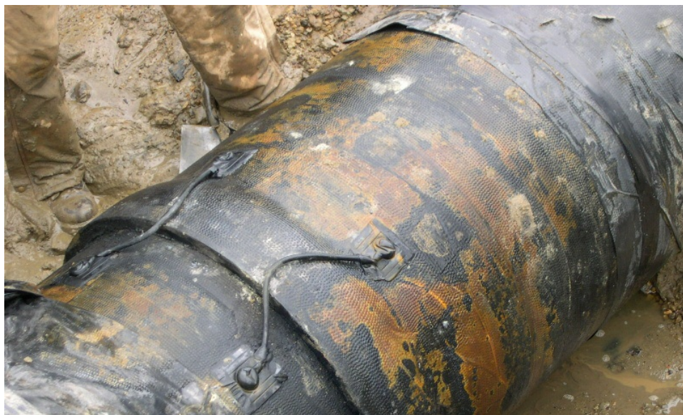
Figure 3. Ductile Iron Pipe Bonded Joint (Southwest Pipeline, 2004)
