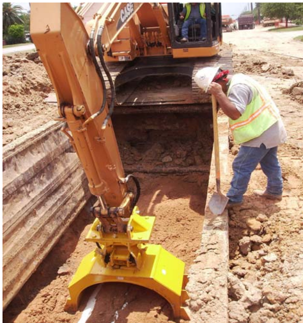
Photo 3: Excavator with vibratory attachment, compacting soil around MK #97.
