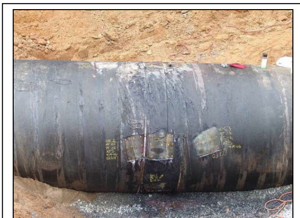
FIGURE 2 Typical External Surface Preparation for Non-Destructive Testing
