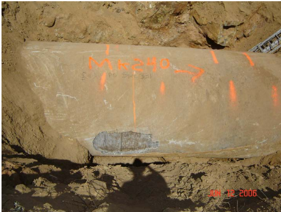
Figure 2 – Post Excavation and Removal of Mortar Lining
