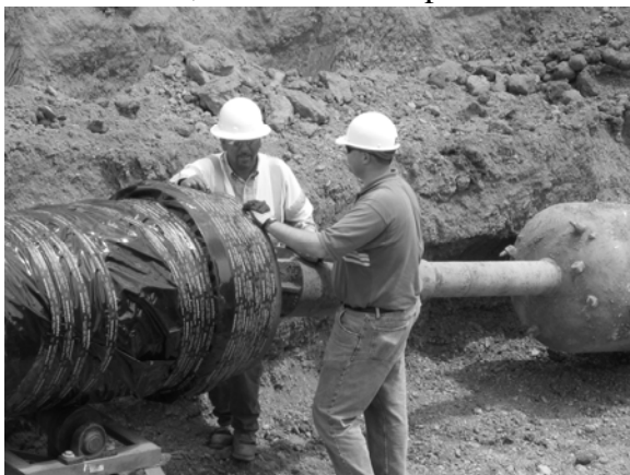
Figure 4 - Flex-Ring Pipe Ready for Pullback
