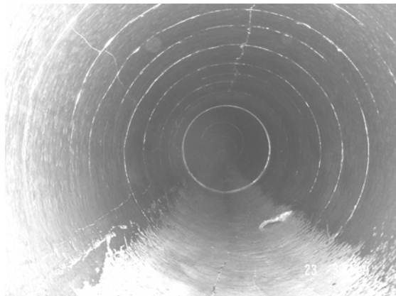
Circumferential cracks
